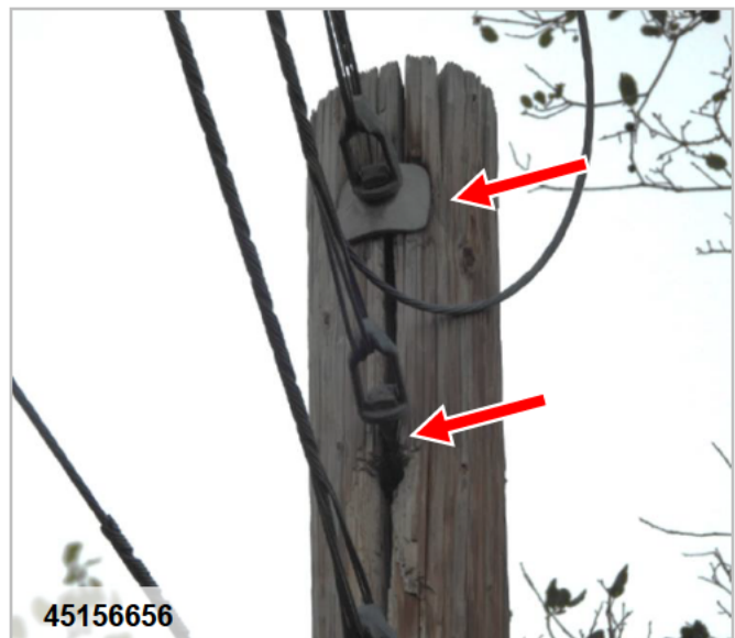
Cracks (along wood grain) through guy pole hardware FDA: Guy pole-Wood | Rotten | Replace
