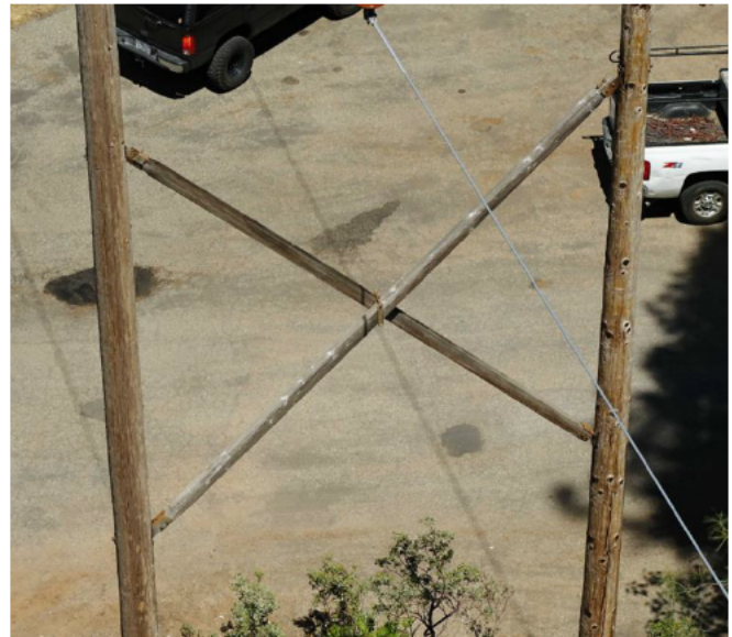
X-brace is weathered with no significant splits FDA: N/A
