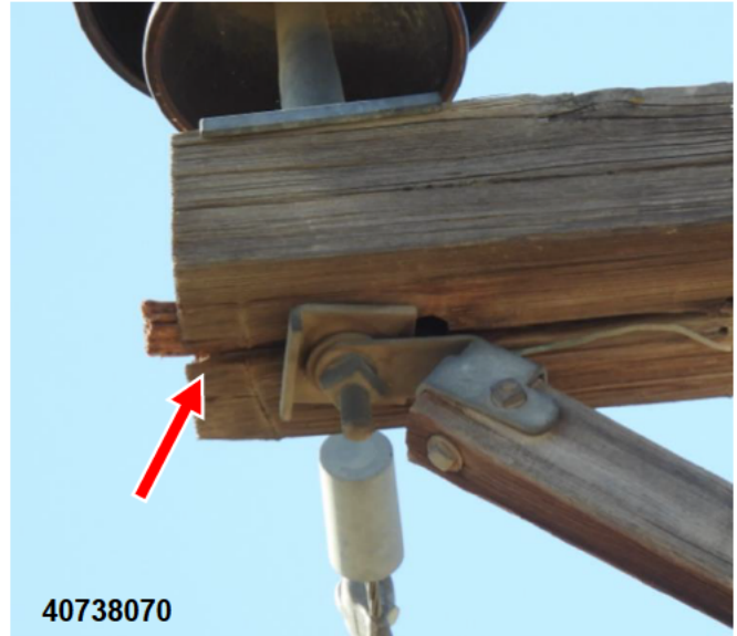
Split crossarm compromising hardware FDA: Crossarm-Wood | No good | Replace
