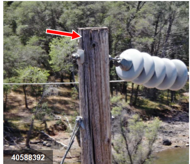
Split pole top, no anti-split bolt present. Dead-end hardware not slipping. FDA: Hardware-Wood | Missing | Install
