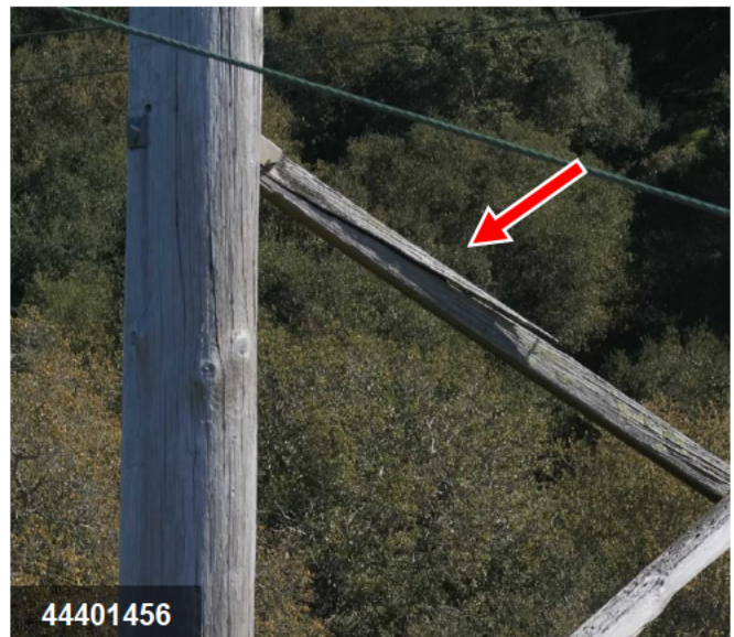
Broken H-frame cross brace FDA: Crossarm-Wood | No good | Replace
