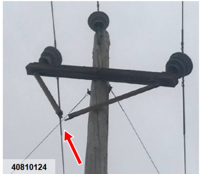
Broken crossarm bracing, compromising insulators FDA: Emergency-Wood | Other | Replace
