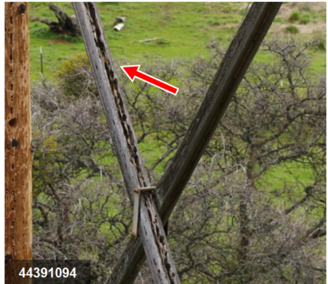
Rotten H-frame cross brace FDA: Crossarm-Wood | No good | Replace
