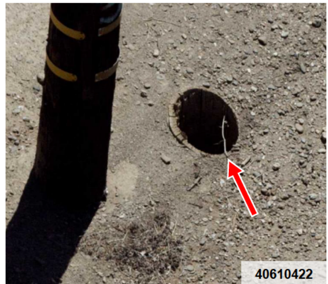
Rotten pole butt. Hole may destabilize the structure.
