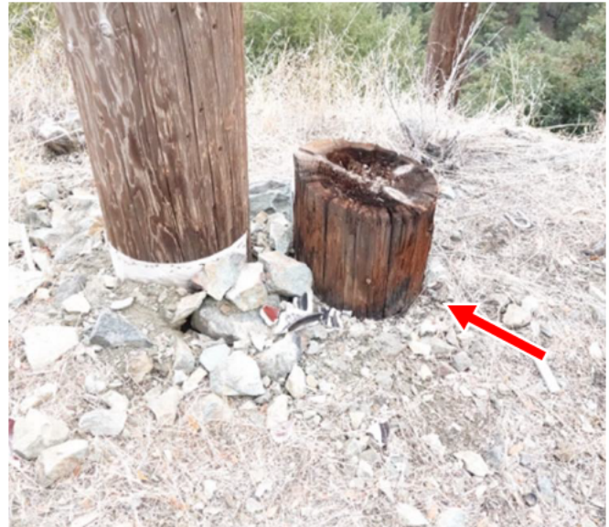
Old pole butt is not rotten FDA: N/A
