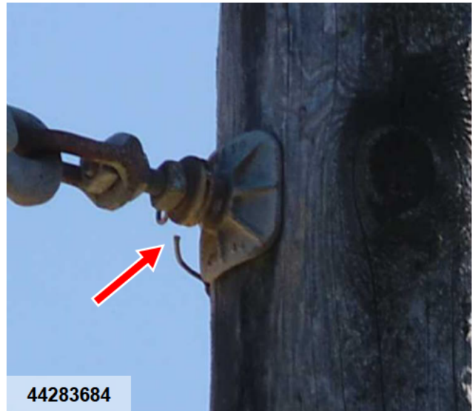
Broken bond wire, < ¼" gap FDA: Emergency | Storm Related | Repair
