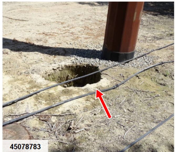
Medium hole (~2' deep) near base of pole. No public access. FDA: Structure-Wood | Debris | Remove
