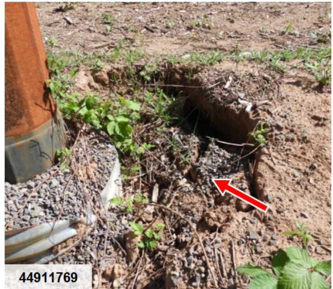
Erosion around pole FDA: Structure-Wood | Debris | Remove
