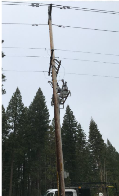
Pole < 3' out of plumb FDA: N/A
