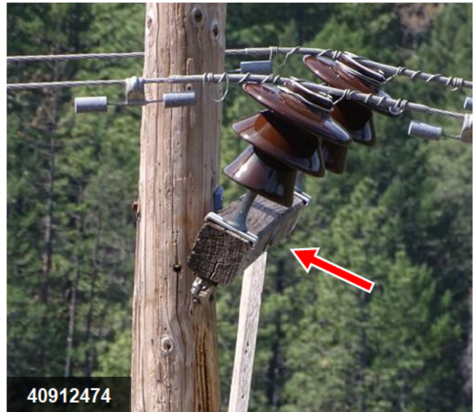
Twisted crossarm impacting insulators FDA: Crossarm-Wood | No good | Replace
