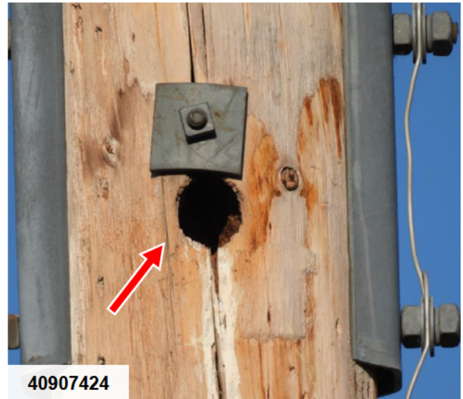
Medium woodpecker hole at pole top near hardware FDA: Structure-Wood | No Good | Replace
