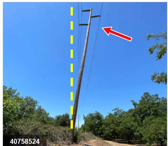
Pole out of plumb, ~5' FDA: Structure-Wood | No Good | Replace
