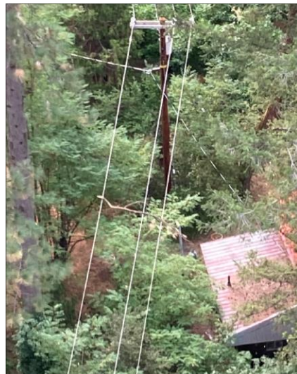
Figure 5: Image of Veg Related Hazard in Sierra County – Tree Branch Caught in Multiple Overhead Phases
