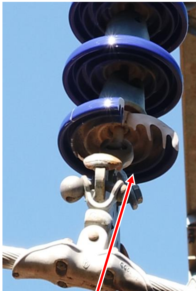
Porcelain disc cracked to the cap.
