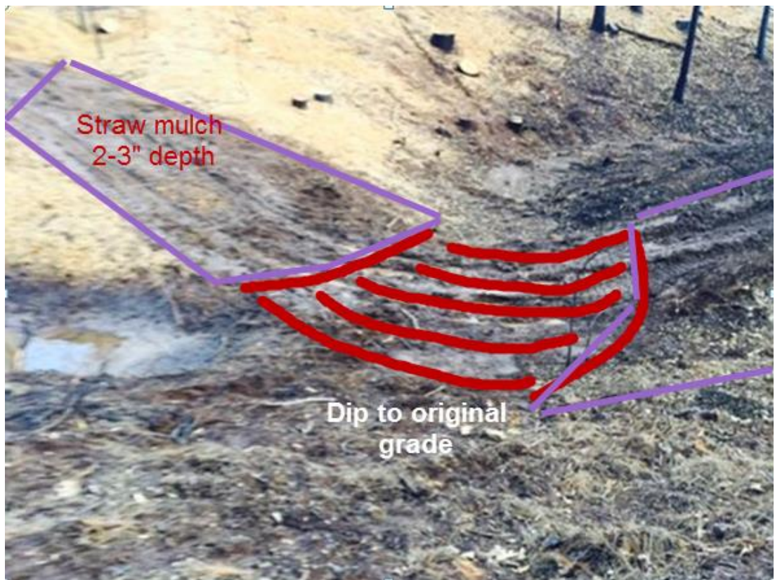
Photo 22- Watercourse crossing restoration detail upon work completion
