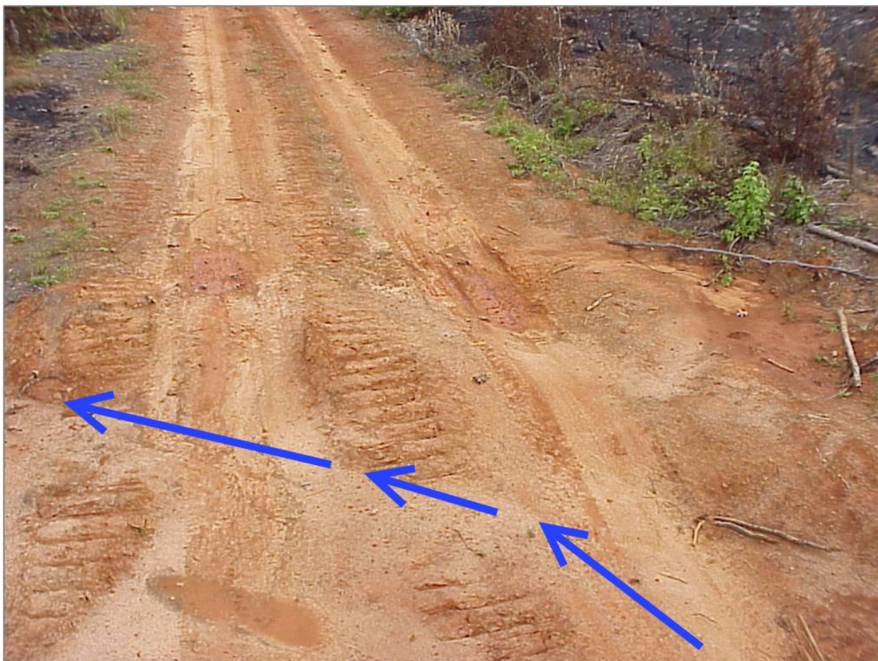
Photo 20- Waterbreak properly constructed. Waterbreak crosses the entire width of the skid trail.
