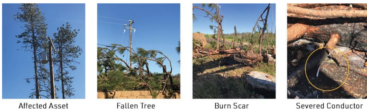
FIGURE PG&E-22-11-1: COVERED CONDUCTOR EFFECTIVENESS – EXAMPLE 1
