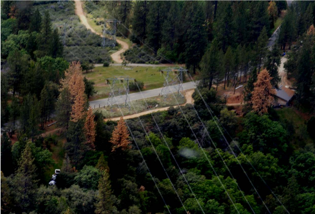
Photo B-16. Hazard Trees Identified Adjacent to a Powerline in a Region 5 Forest
