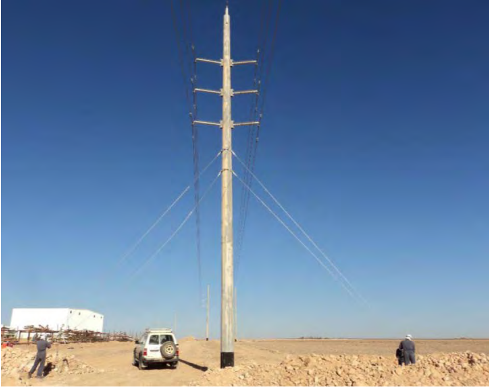
Photo B-9. Example of Guy Wires on a Pole
