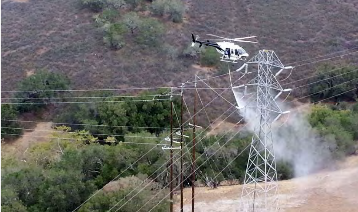
Photo B-1. Example of Utility Washing Insulators on a Transmission Tower
