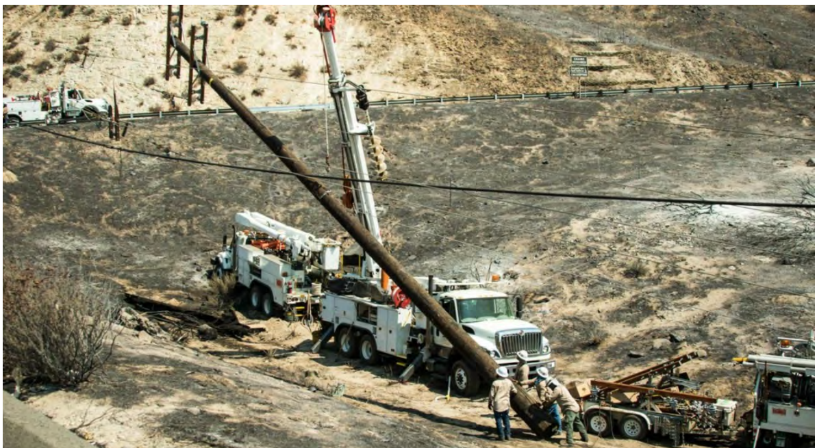
Photo B-19. Emergency Work Following a Wildfire
