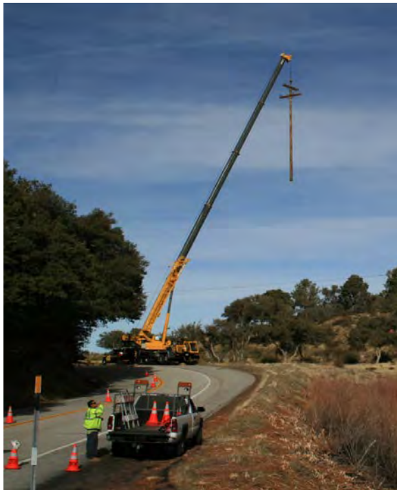
Photo B-14. Pole Set by Crane
