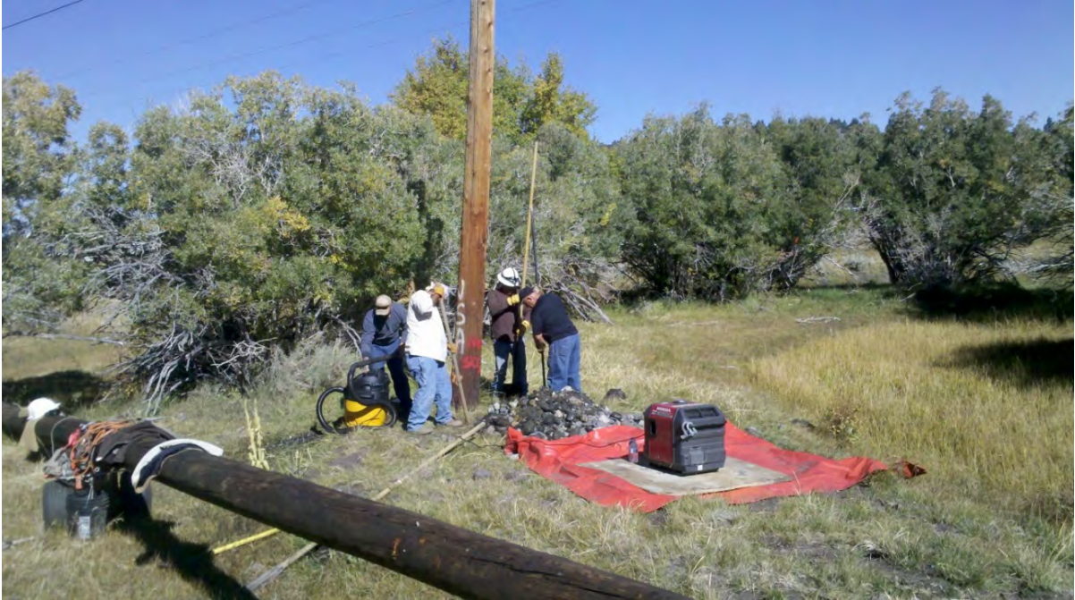
Photo B-11. Hole Excavation – Spoon, Spade, and Bar
