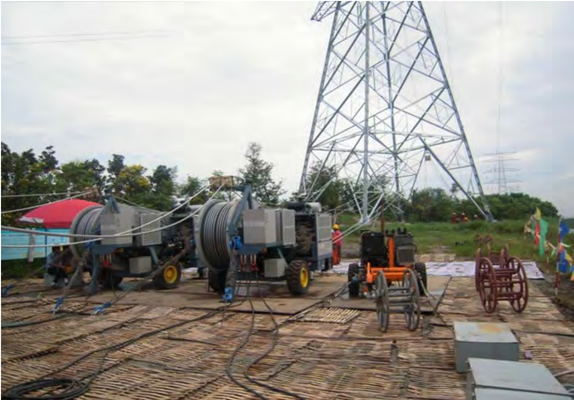
Photo B-18. Example of Large Reconductoring Project
