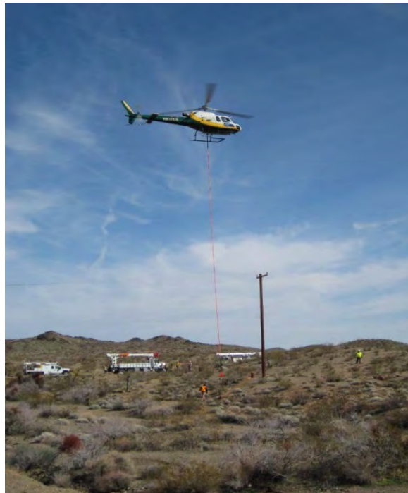
Photo B-15. Pole Set by Helicopter
