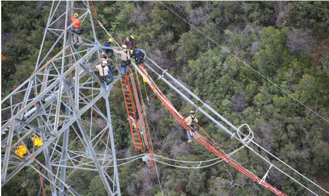
Photo B-3. Example of Utility Working on a Transmission Line
