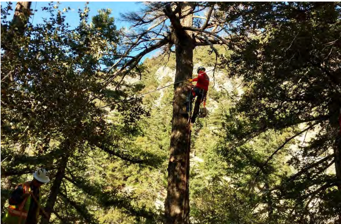
Photo B-17. Utility Crew Topping Hazard Tree
