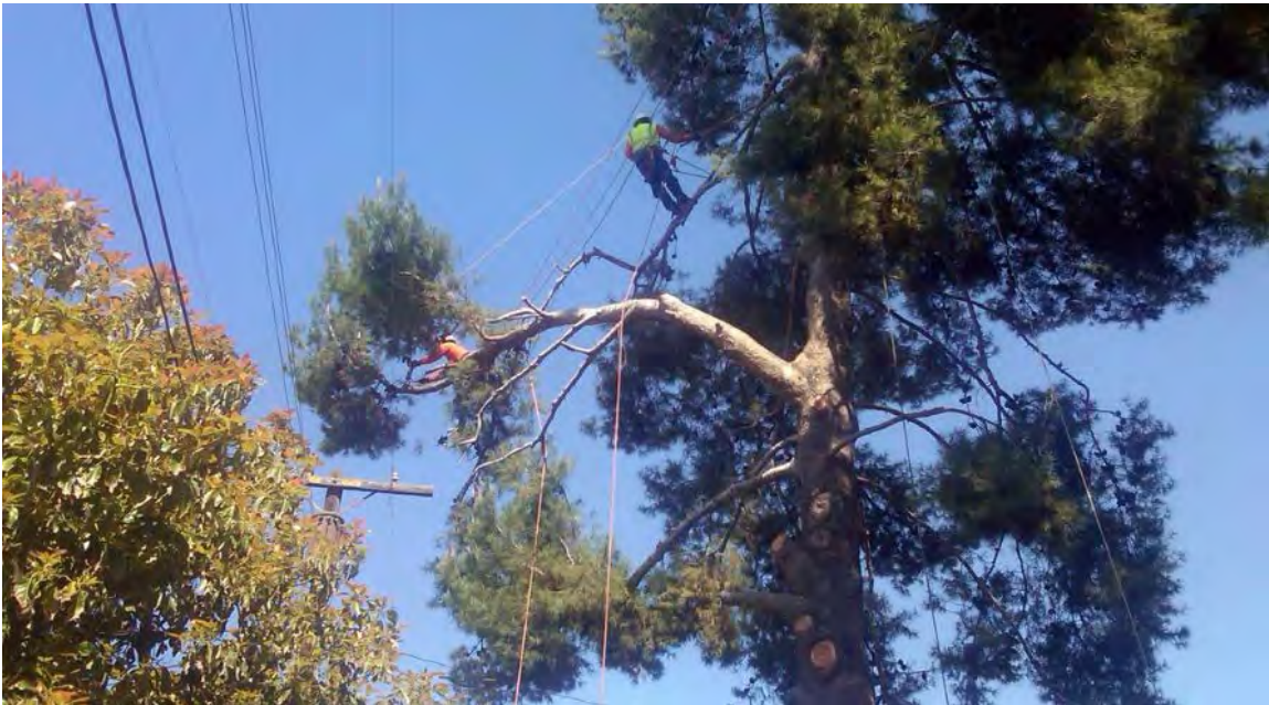
Photo B-8. Example of Utility Clearing Powerlines of Vegetation
