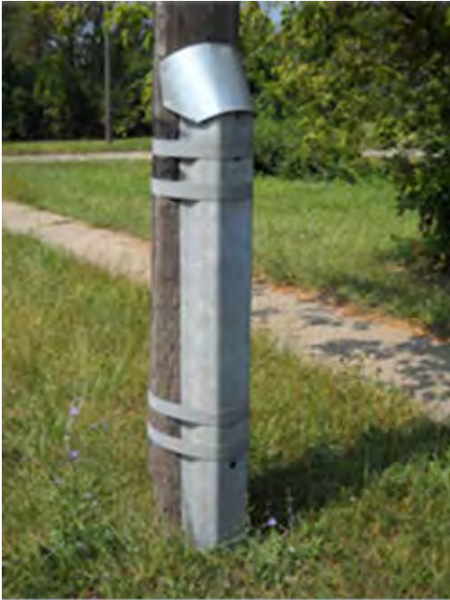
Photo B-4. Steel Trussing on a Wood Pole
