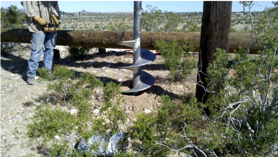
Photo B-10. Drilling New Pole Location
