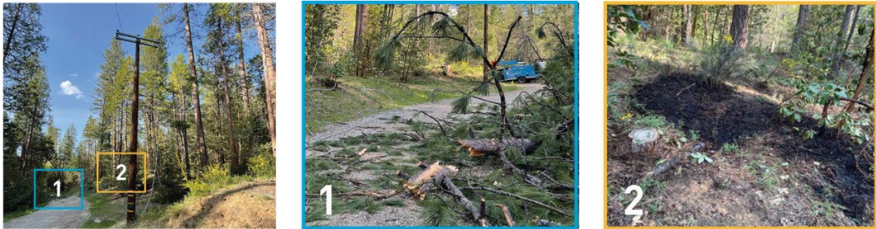
FIGURE PG&E-22-11-2: COVERED CONDUCTOR EFFECTIVENESS – EXAMPLE 2
