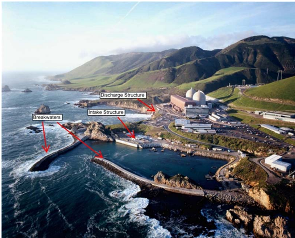
FIGURE 4-1 DCPP'S INTAKE STRUCTURE, BREAKWATERS, AND DISCHARGE STRUCTURE LOOKING NORTH
