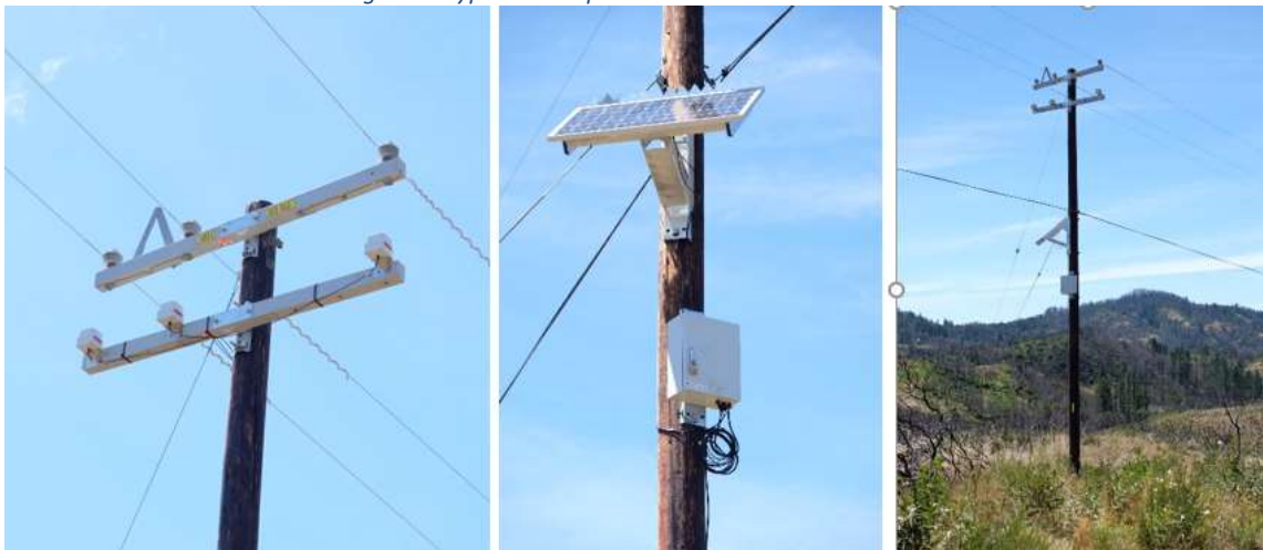
Figure 9. Typical solar-powered RF data collection unit
