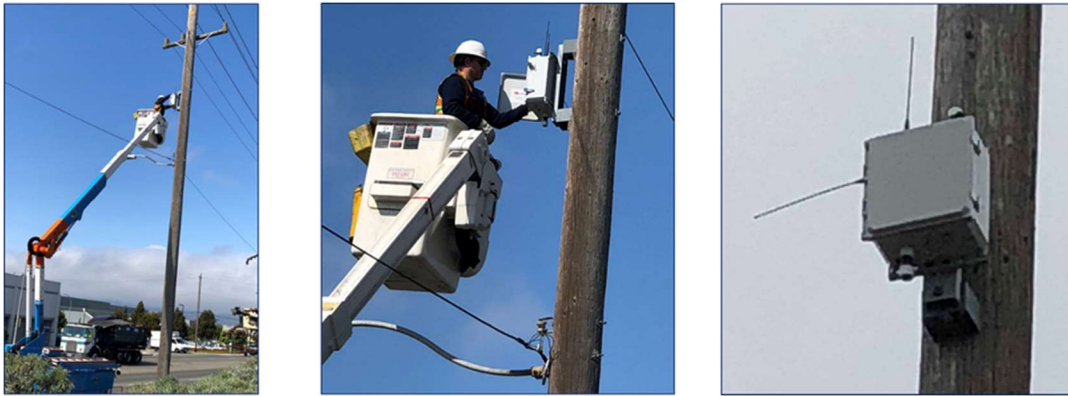
Figure 3. DRLM Sensor Installation
