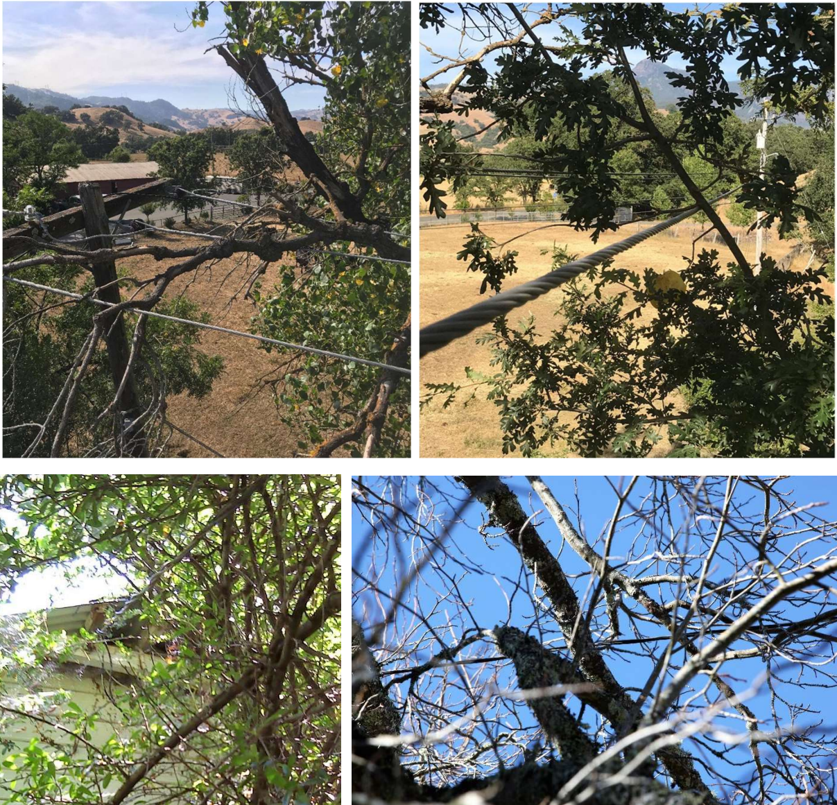
Figure 11. Examples of vegetation on secondary conductors
