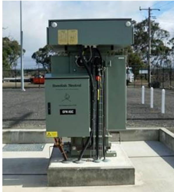
FIGURE PG&E-7.3.3-5: ARC SUPPRESSION COIL / GFN
