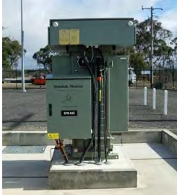
FIGURE PG&E-7.3.3-5: ARC SUPPRESSION COIL / GFN
