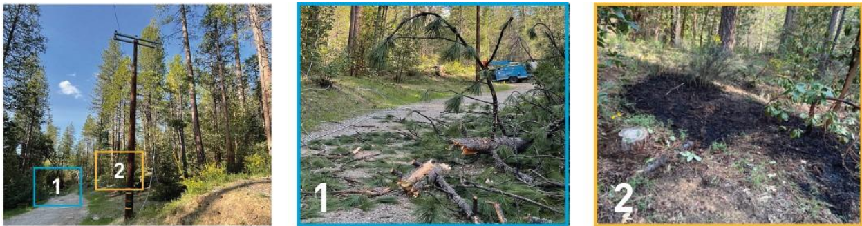
FIGURE PG&E-22-11-2: COVERED CONDUCTOR EFFECTIVENESS – EXAMPLE 2
