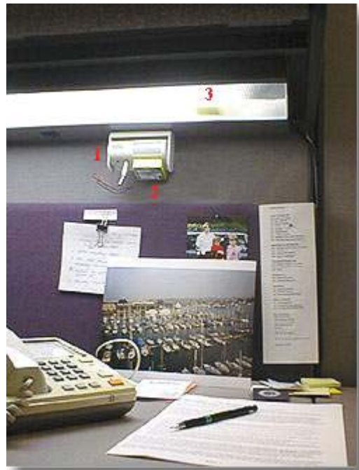
Figure 3 Occupancy study toolkit placed to monitor of under-cabinet task light use and occupancy.
