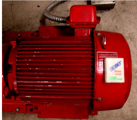
Figure 4: Motor logger installed on pump motor
