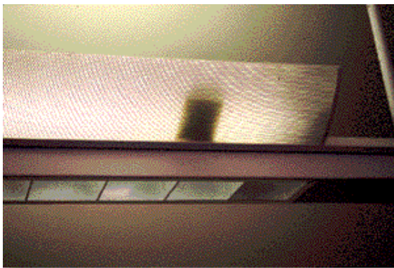
Figure 1: A HOBO logger placed close to the lamp of an overhead fluorescent lighting fixture
