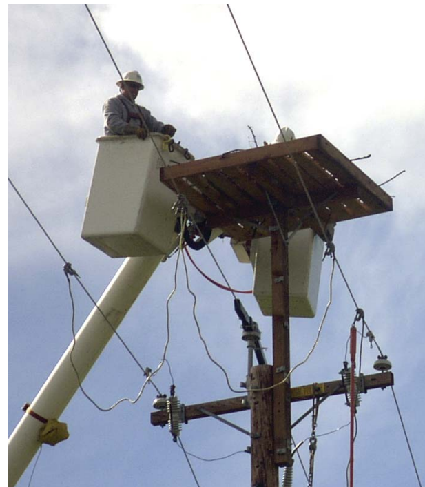
A PG&E crew installs a nest platform near Clear Lake. Nest platforms reduce outages and are preferred by large birds, such as ospreys.
