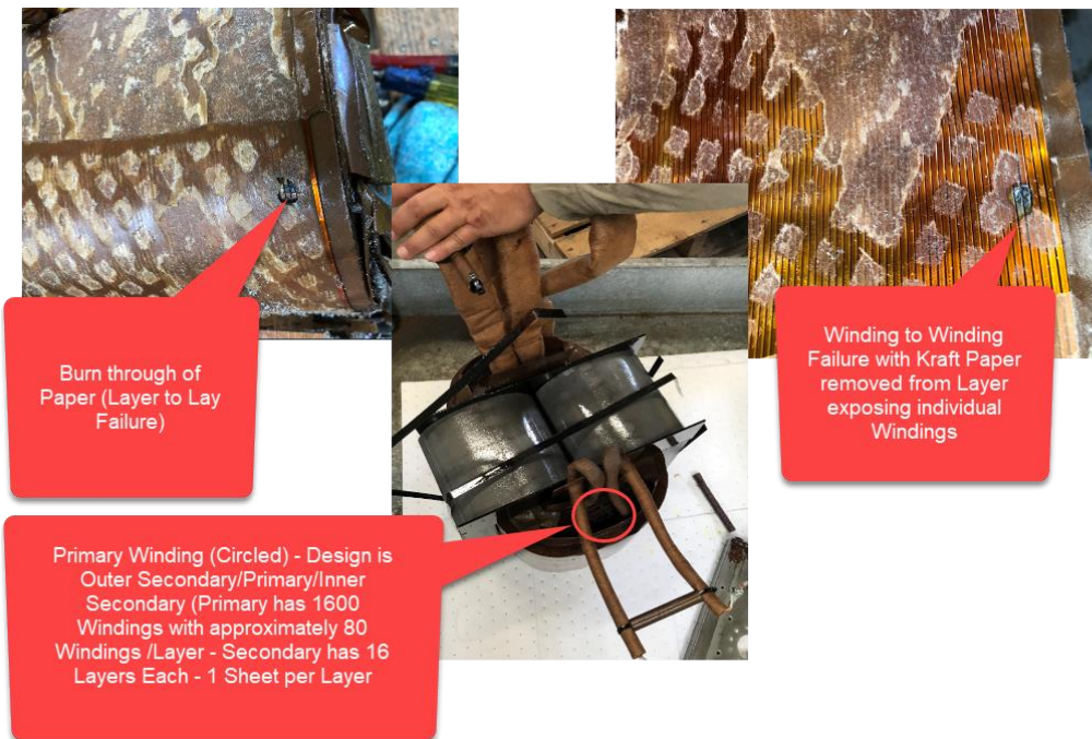
Figure 21: Photos from windings failure teardown
