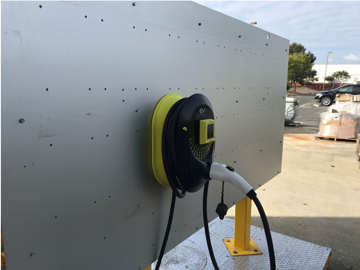
Figure 16. Commercial EVSE Install - Fremont Meter Farm
