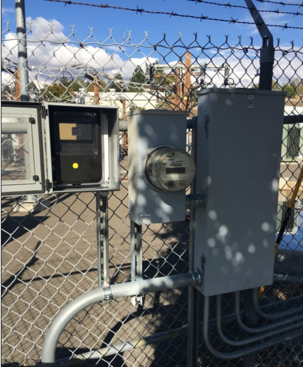
Figure 23. Retrofit Installation–ATS in San Ramon
