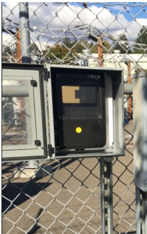
Figure 24. Retrofit Box Install
