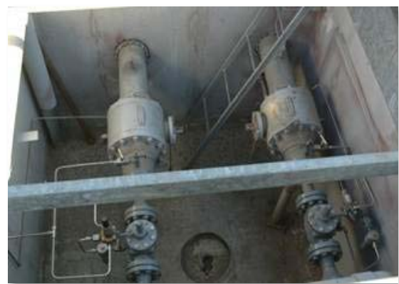
Figure 12 – A Simple Station – Vaulted
