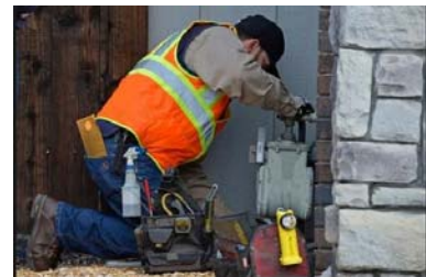
Figure 14 – PG&E Employee Working on CCE
