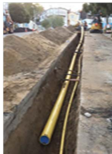
Figure 13 – Distribution Main Replacement Project
