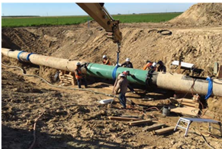
Figure 22 – Pipeline segment replacement following a strength test.
