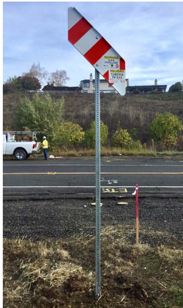
Figure 29 – Crew completing the installation of a new pipeline crossing marker
