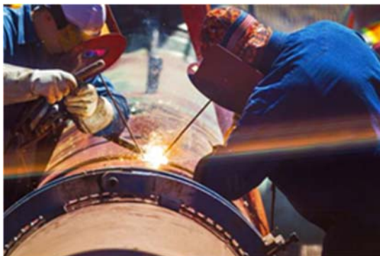
Figure 16 – Two PG&E Welders
