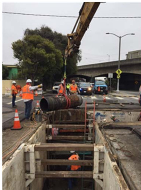
Figure 23 – Crew Replaces Vintage Pipe in San Francisco
