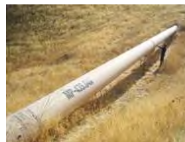
Figure 10 – Transmission Pipeline Span
