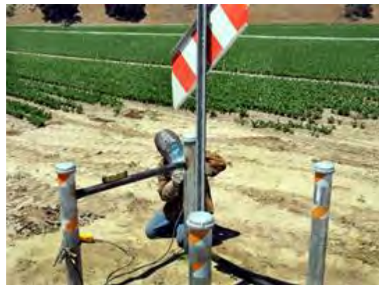
Figure 29 – Installing a Pipeline Marker and Physical Protection
