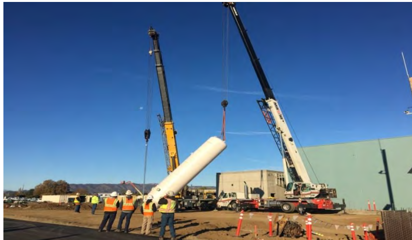
Figure 52 – Construction in Progress at PG&E’s Winters Training Center
