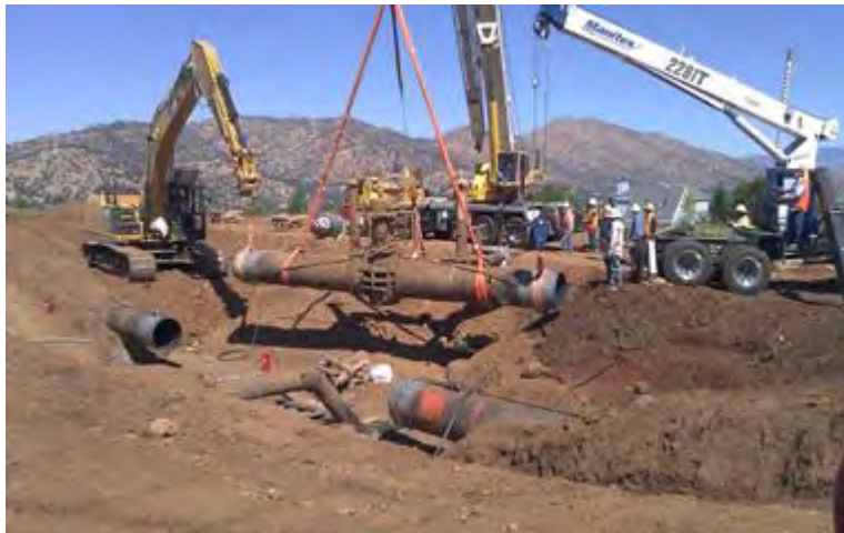
Figure 18 – Main Line Valve Removal Before a Strength Test
