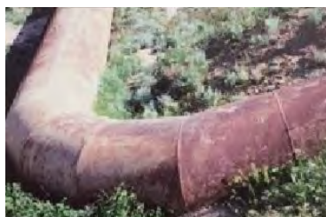
Figure 20 – Miter Bends
