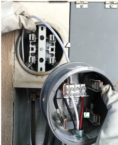
Figure 5 Extend Insulated Wires Past the LFNC Conduit
