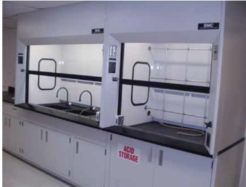
Figure 5.01 Example of horizontal sash chemical fume hoods
