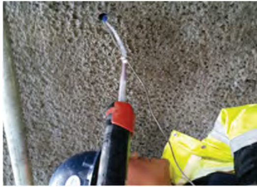
Filling an anchor bolt hole with epoxy.
