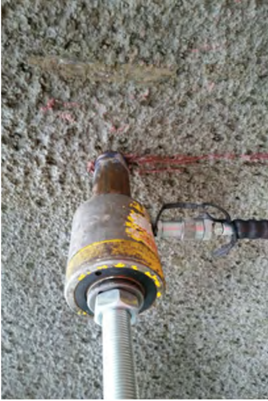
Anchor bolt testing.
