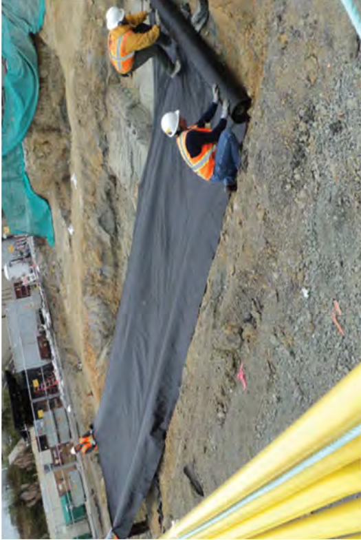
Laying geotextile before backfilling north Unit 2.
