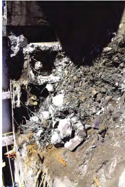
Debris from the north-south tunnel ready to be loaded out.
