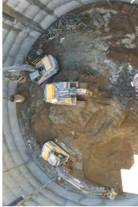
Removing concrete from -58' EL to -66' EL.
