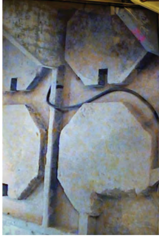
The final cleaning in the LRWB.
