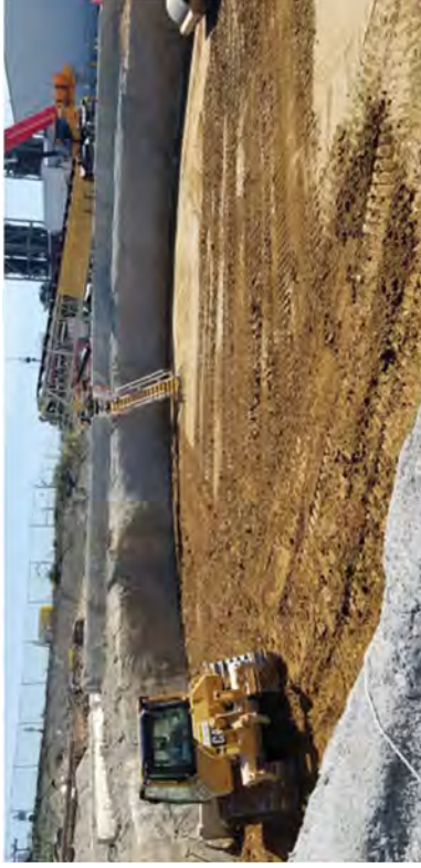
Impermeable layer installation
