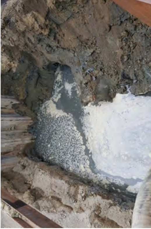
Groundwater control in Area D.
