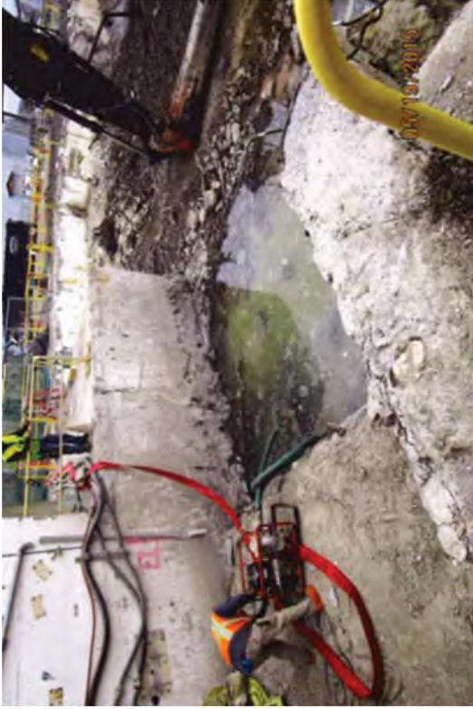
Dewatering the excavation.
