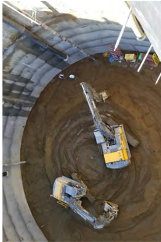
Excavating the first 1-foot cut of re-use soil.
