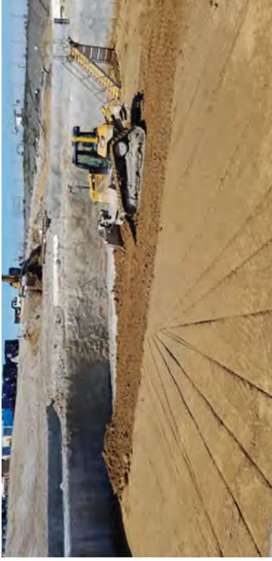
Impermeable layer installation
