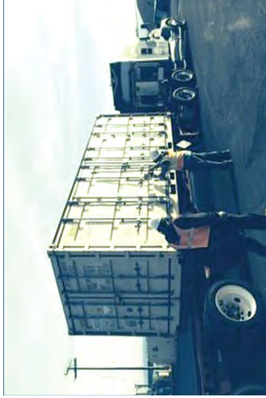
Performing the final survey and inspection on a container containing DAW, filters, demineralizer vessel, and resin before it is shipped to a waste facility.
