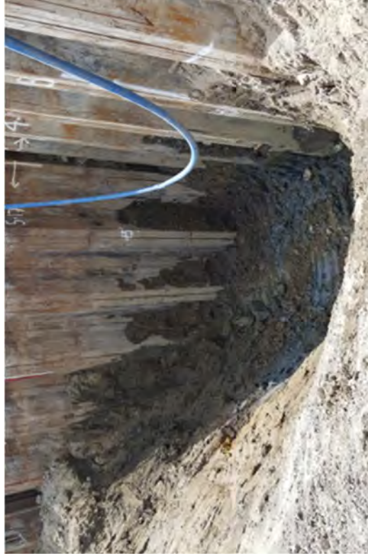
Continuing to excavate and backfill Area D.
