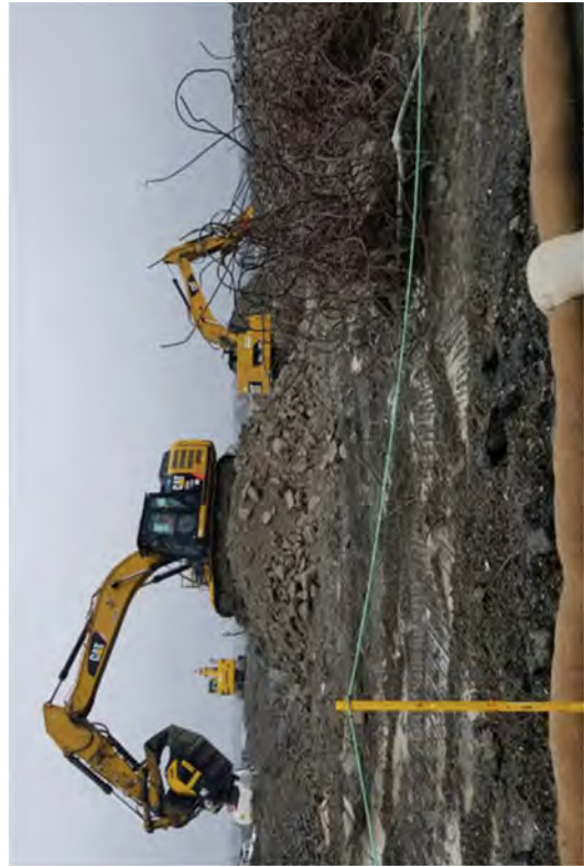
Processing concrete.
