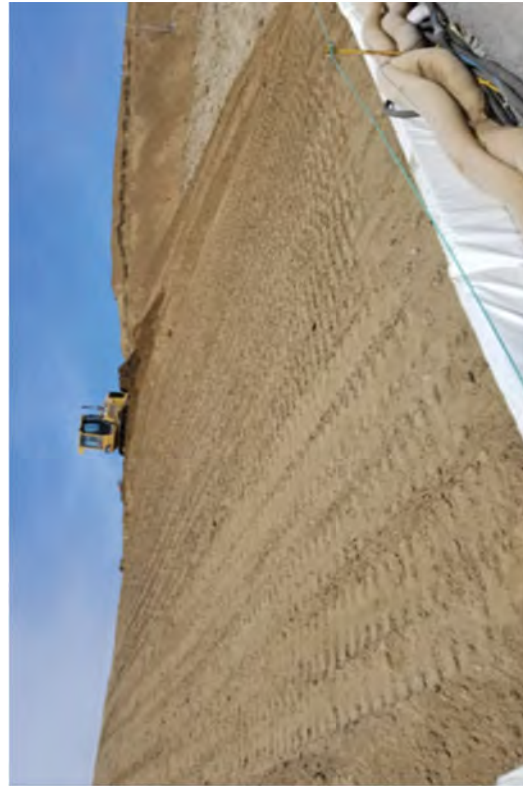
Reshaping the upper yard soil stockpile.
