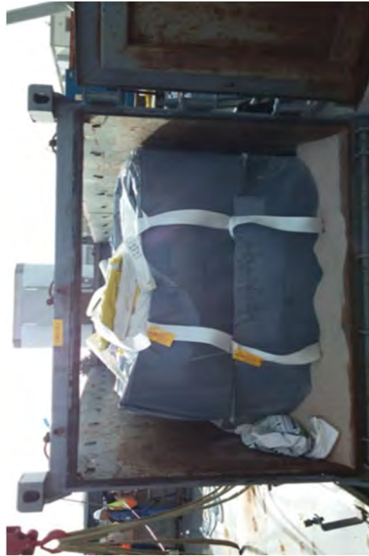
Waste boxes with concrete debris from the LRWB.
