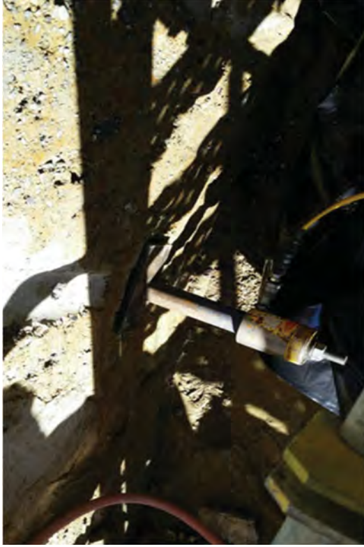
CSM Wall stair tower anchor bolt testing.
