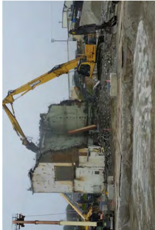
Demolishing the RFB roof.
