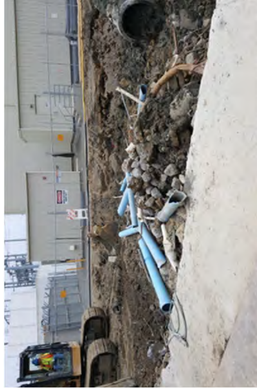
Commodity and pipe removed from Area A.
