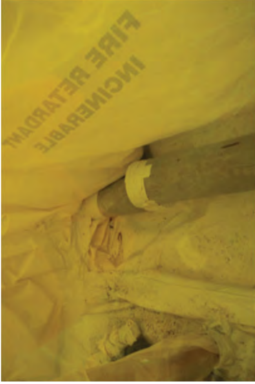
This obstruction had to be cut inside an enclosure.
