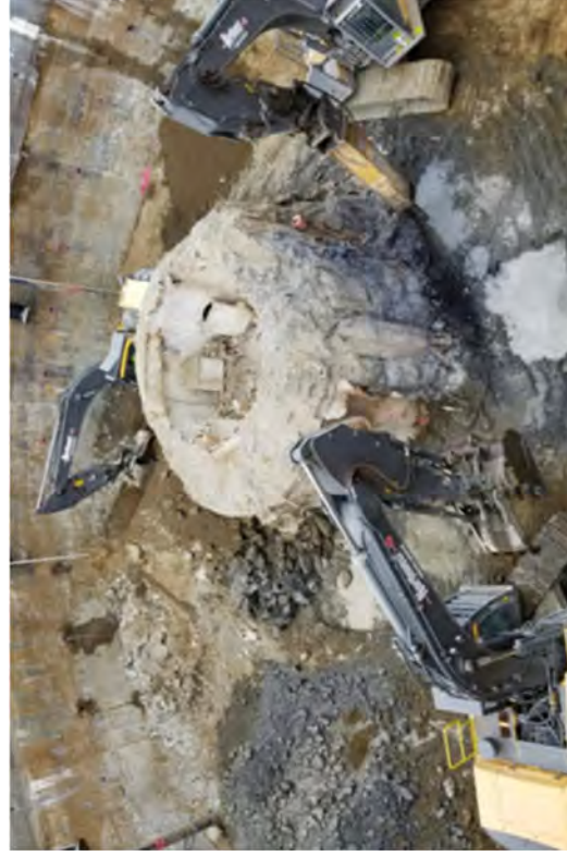
Demolishing the outer concrete of the Caisson at -24' EL to -30' EL.
