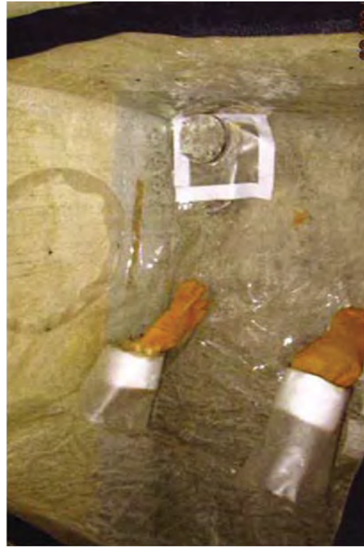
A glove bag set-up to survey pipe in the Demineralization Room.
