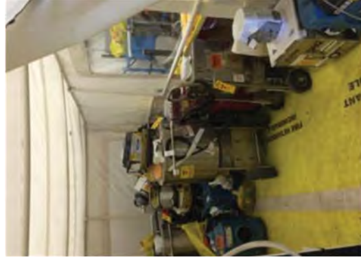
HEPA vacuums and bags being prepared for processing and disposal.
