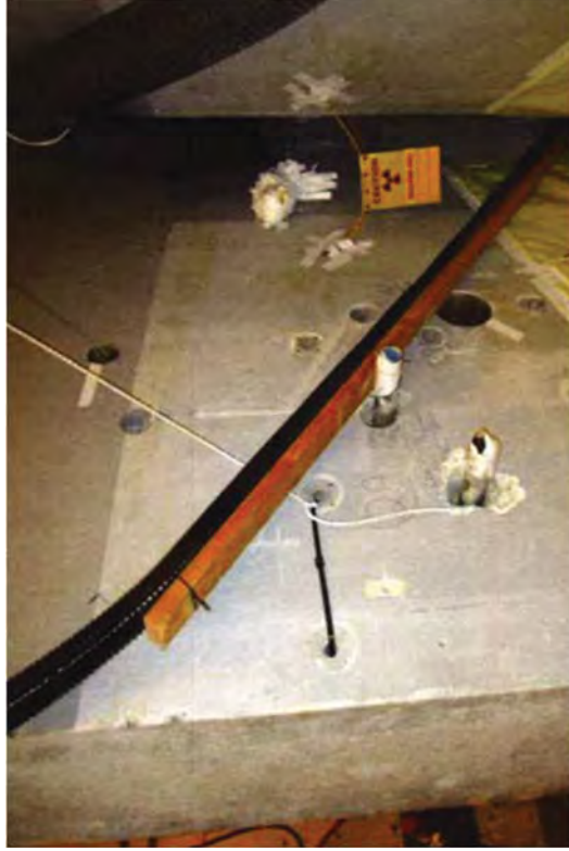
Part of the makeshift chute into the west pipe chase.
