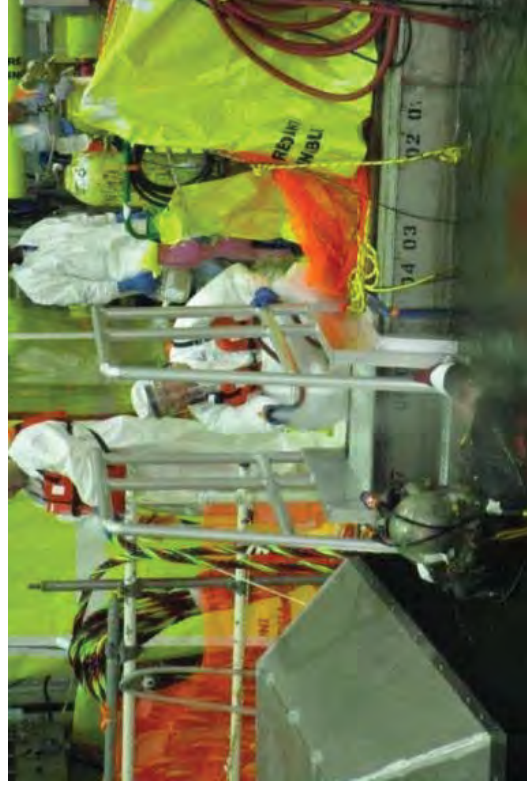
A Diver exiting the SFP after performing the first cut on the liner.
