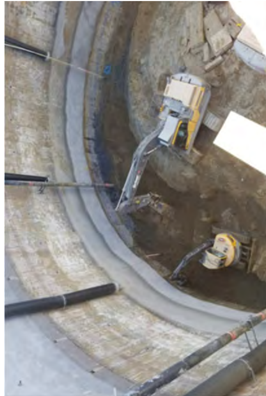
Removing re-use soil from -46' EL to -52' EL.
