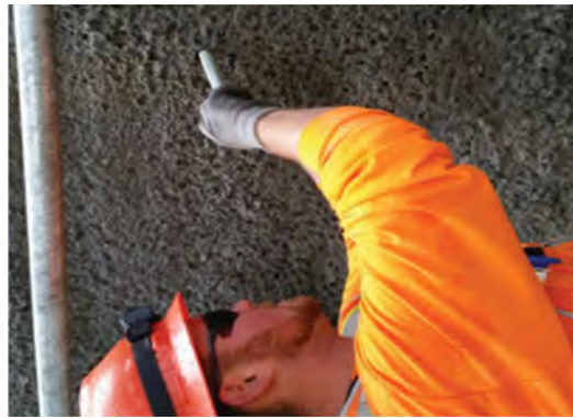
Setting an anchor bolt into the CSM wall.
