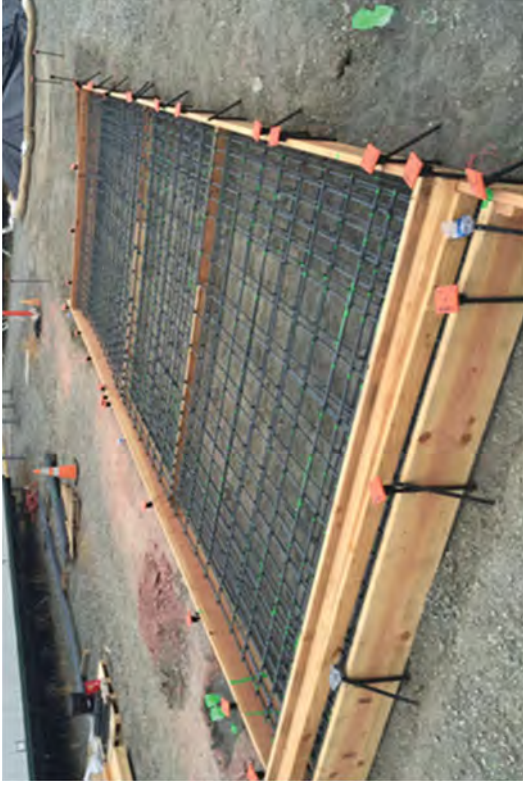
The completed forms with horizontal rebar installed.
