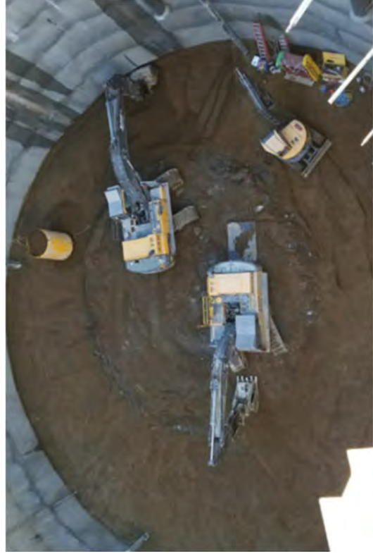
Excavating material for re-use at -70' EL to -74' EL.
