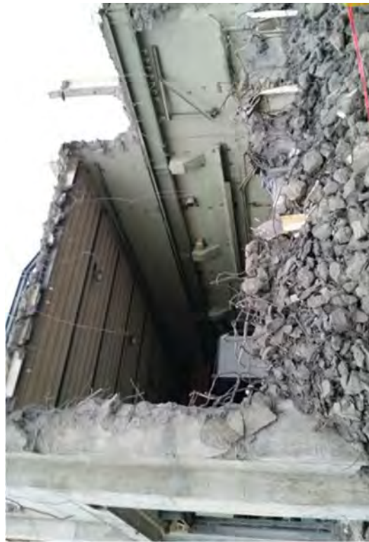
The RFB during morning inspection.
