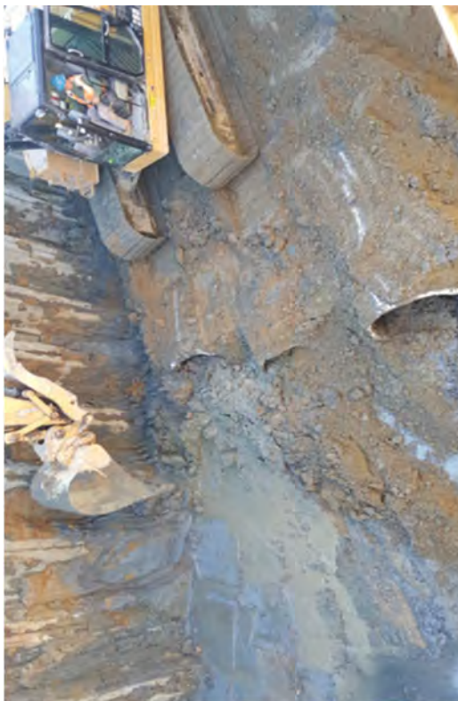
Pipe excavated for removal in Area C.
