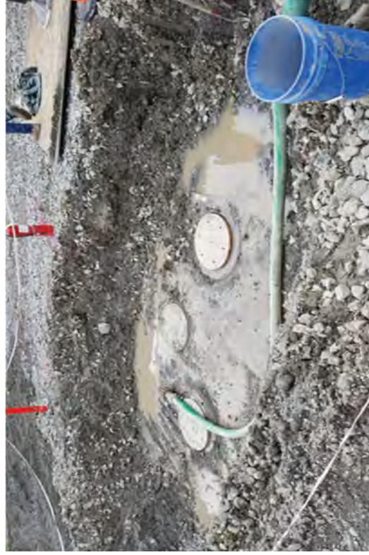
The abandoned Vortex vault that was dug out and exposed.
