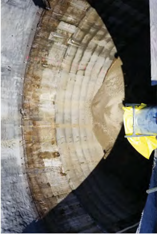
Continuing to backfill the Caisson excavation.
