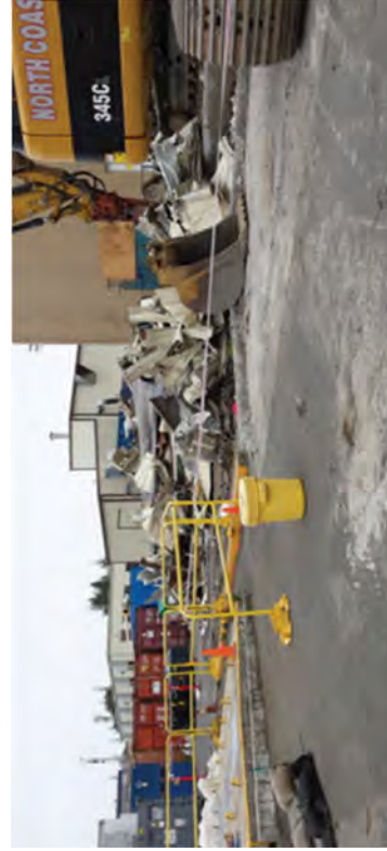
Size-reducing sheet metal and steel so that it could be loaded into an intermodal.
