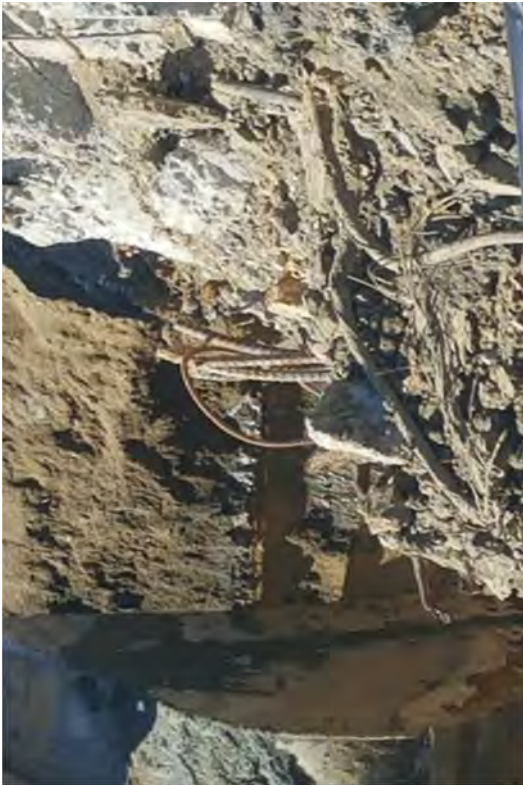
Circulating Water Lines Removal
