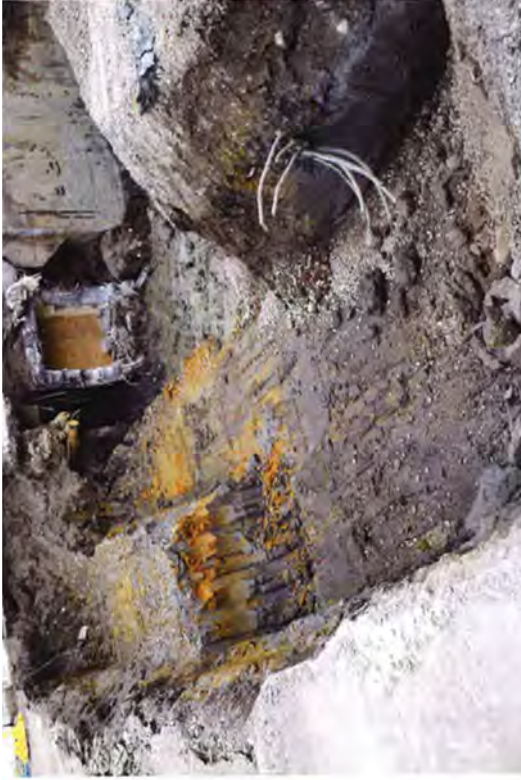
North Yard Pre-Trench
