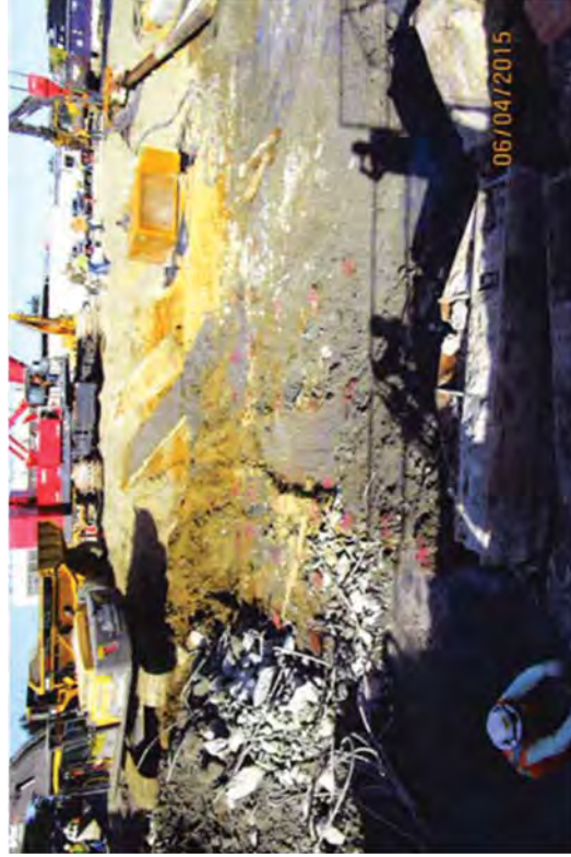
Wooden plings marked for extraction.
