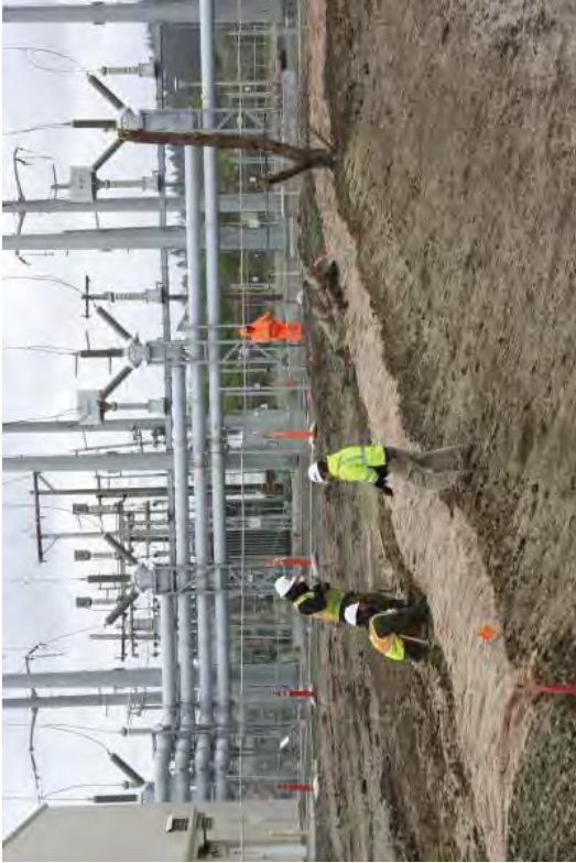
Jute matting being placed to protect hydro seeding.
