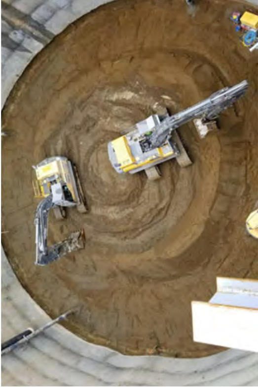
Excavating re-use soil at -68' EL.
