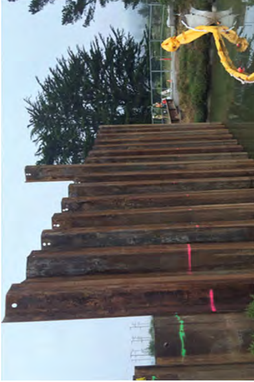
Installing Intake Canal sheet piles.
