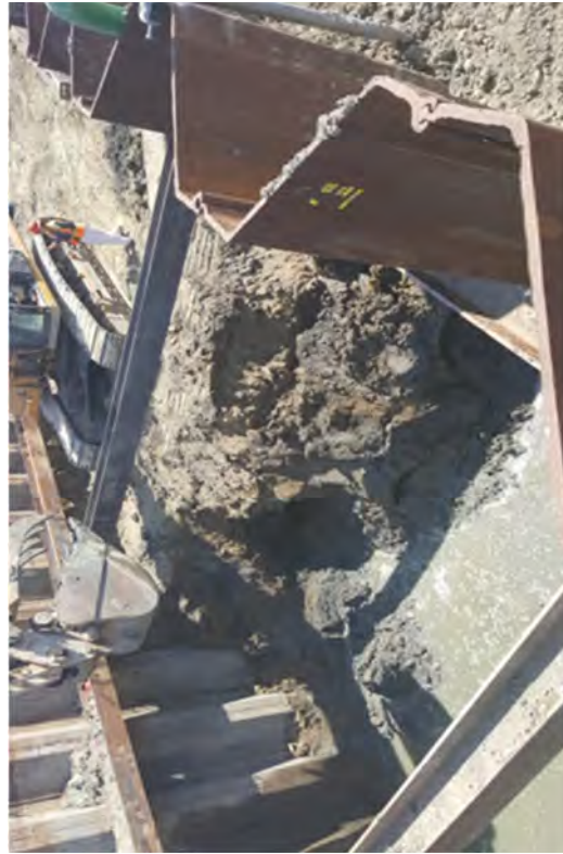
Removing pipe from the deep excavation of Area C.
