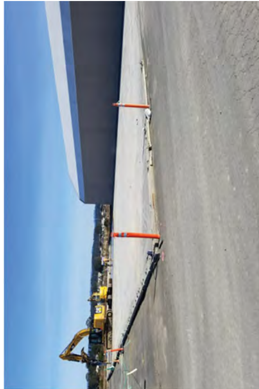
Dewatering the SMF slab to the GWTS.
