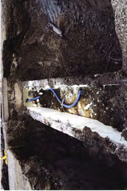
The remaining section of LRW tunnel exposed.
