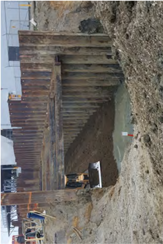
Circulating Water Lines Removal
