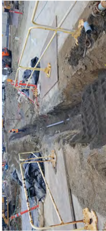
The sewer line trench in the process of being backfilled.
