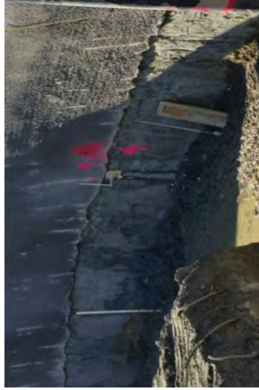
Completed core hole grout set-up.
