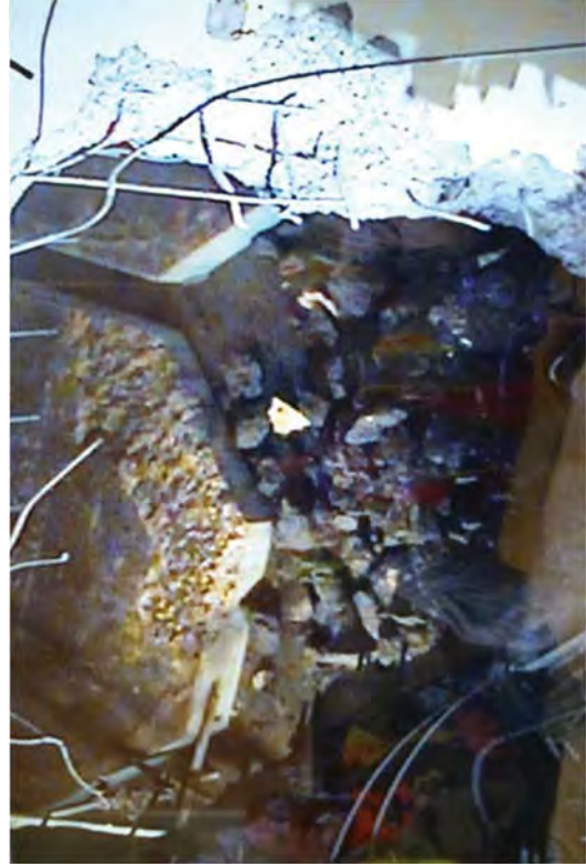
The concentrated waste tank wall opening layout and demolition
