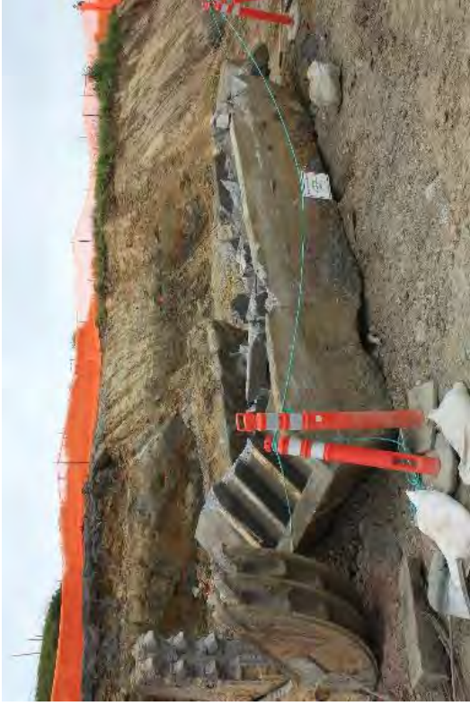
Old steps behind Unit 2 in bank removed.
