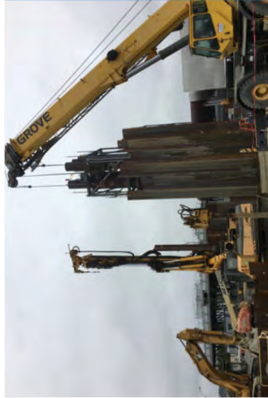
Installing sheet pile in Area C.
