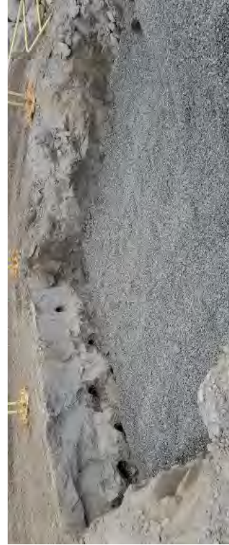
15 foot CSM breach.
