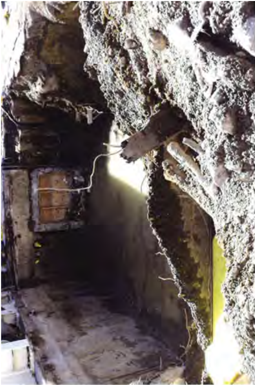
North Yard Pre-Trench
