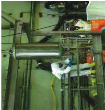
Lifting the solids collection filter from the SFP before plugging its drain and moving it to the decontamination and wrapping area.
