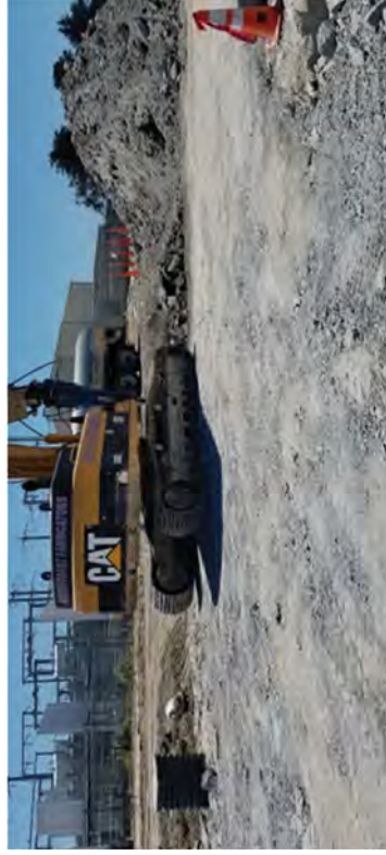
Slurry Cap removal.
