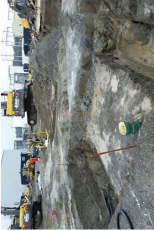
Caisson Pre-Excavation
