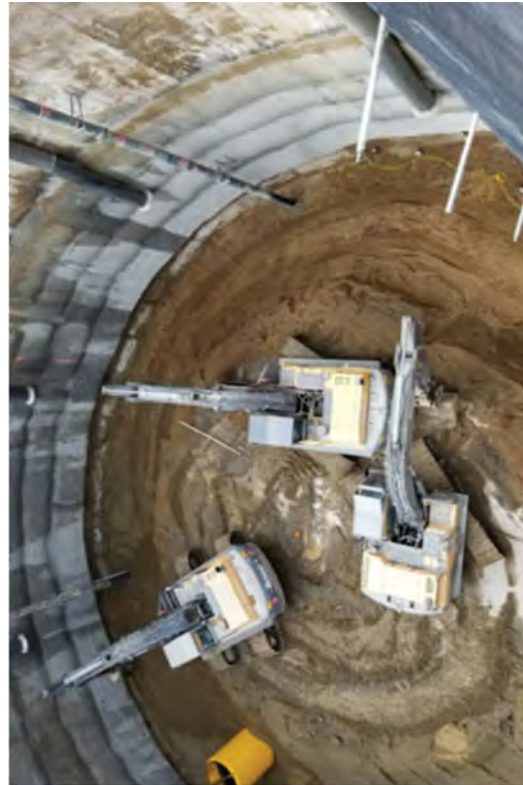
Removing soil for re-use from -60' EL to -66' EL.
