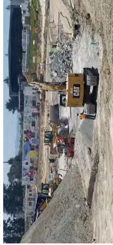
Slurry Cap removal.
