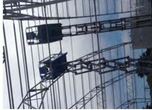
Erecting the SMF Tent 1 Structure.
