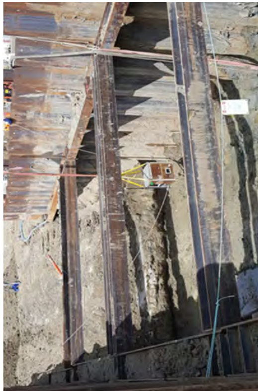
Area D after completing the radiological FSS survey.
