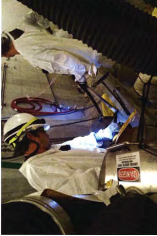
Cutting guard pipe at elevation -14' EL.
