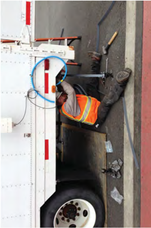
Affixing anchors to the GARDIAN trailers.
