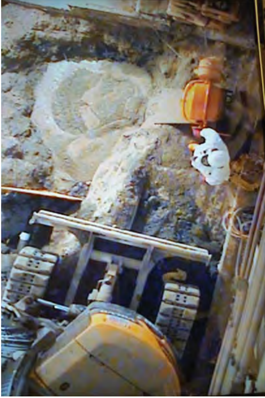
Grouting the LRW sump.
