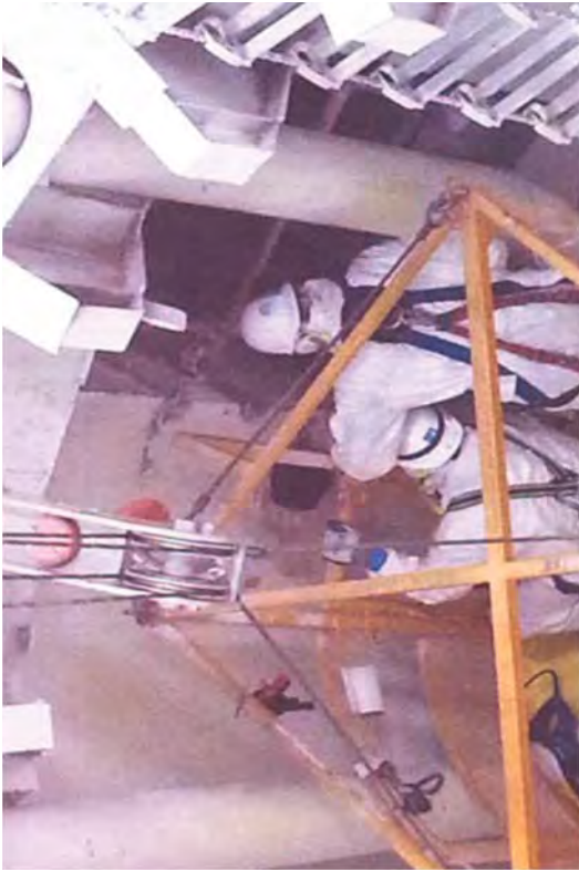
Capping the heat exchanger pipe in the drywell.
