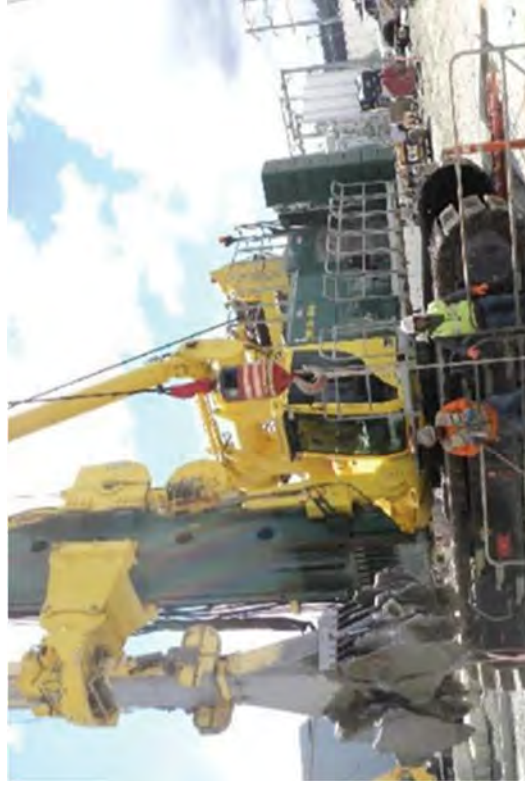
Technicians taking a sample from one of the last deep panels.
