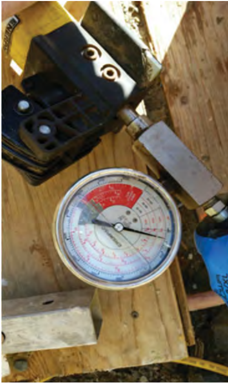
CSM Wall stair tower anchor bolt testing.
