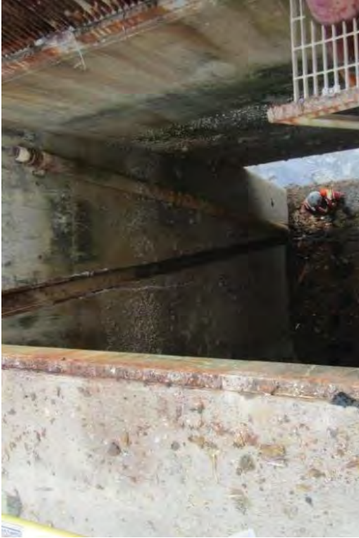
An Intake Structure cell before removing barnades and surveying the walls.
