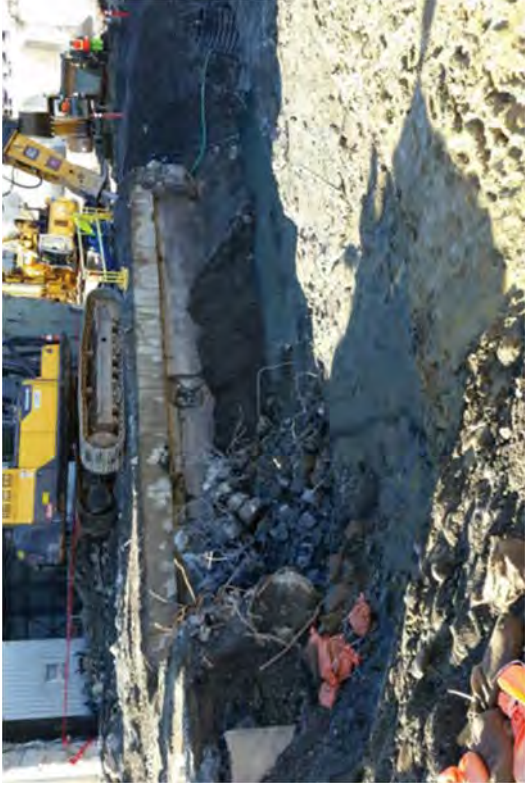
Removing the Off-Gas Tunnel.
