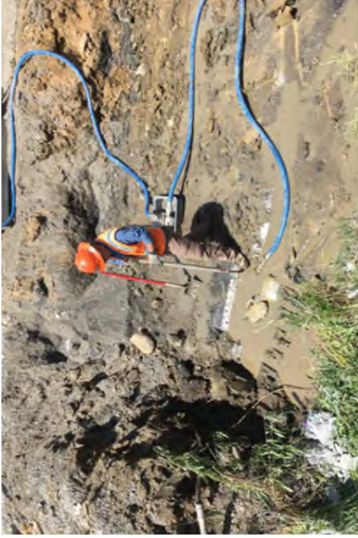
Pumping ground water out of an OWS raceway excavation.
