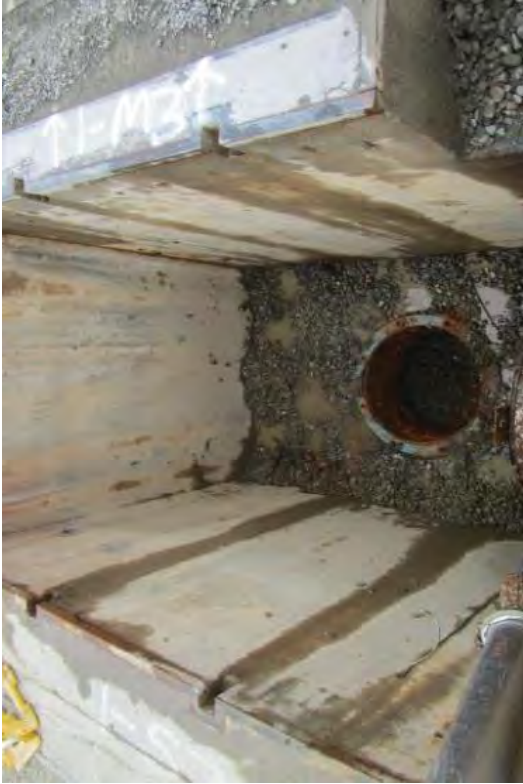
A pipe exiting a shallow cell.
