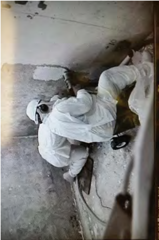
Shaving the walls of the concentrated waste tank room.
