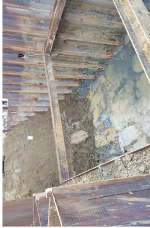
Backfilling material into Area D.
