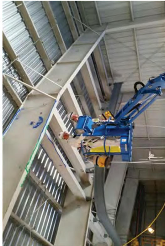
Decontaminating the West End of the LRWB.
