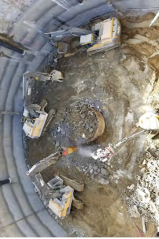
Demolishing concrete at -52' EL to -58' EL.
