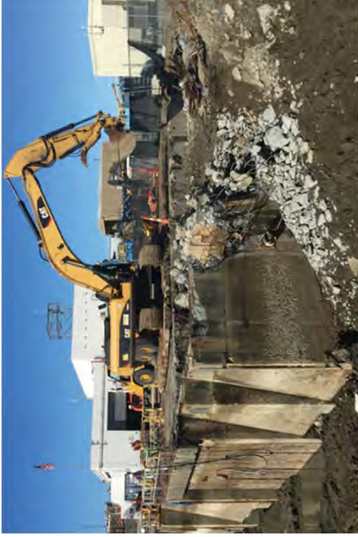
Demolishing the Unit 3 Intake Structure.
