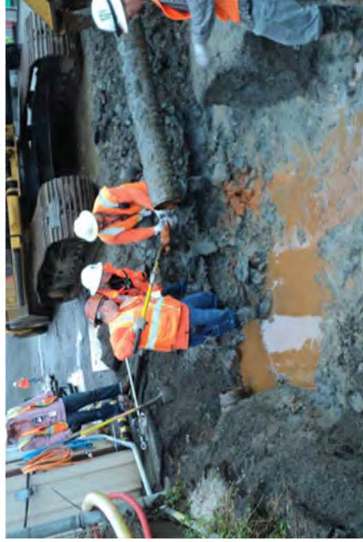
RP collecting samples from corrugated pipe.
