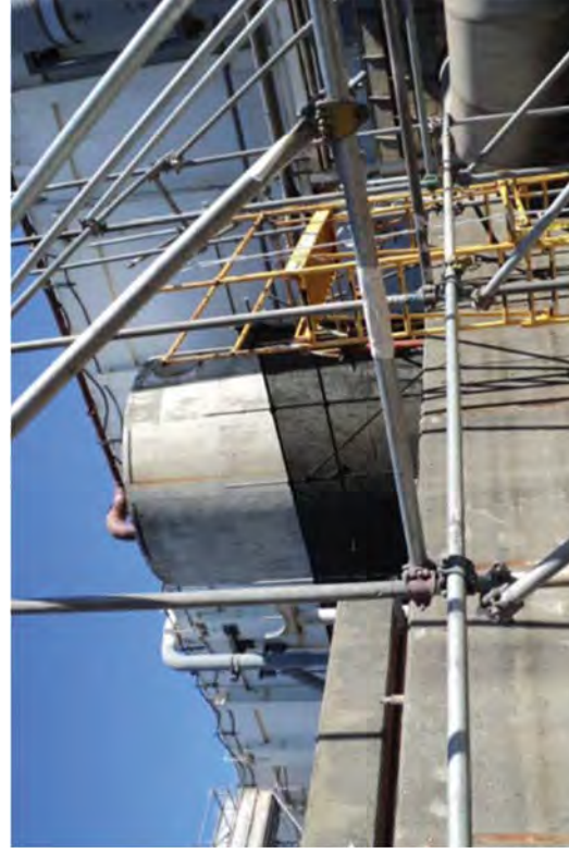
Scaffolding was installed to support a protective netting wall around building.
