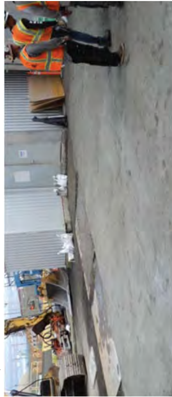
An excavator using the hammer to soften and penetrate the surface so that CLSM can penetrate after the final load out.
