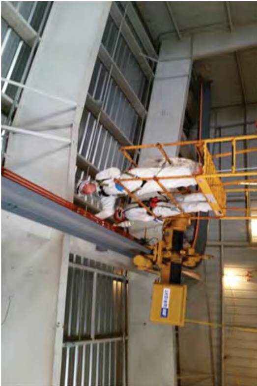
Decontaminating the interior roof beams of the LRWB.
