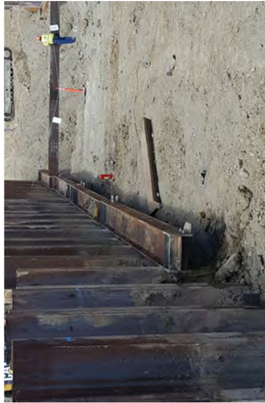
A water system installed on a sheet pile wall.
