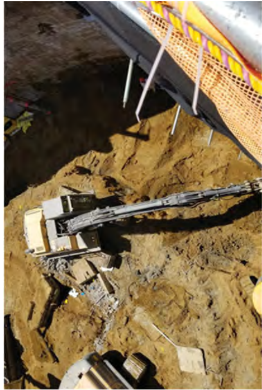
Removing soil from -34' EL to -40' EL
