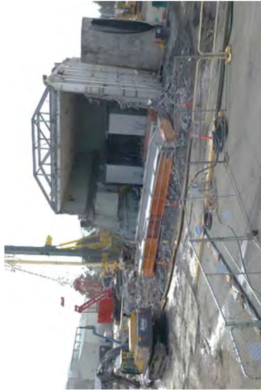
Preparing trolley rails for size reduction.
