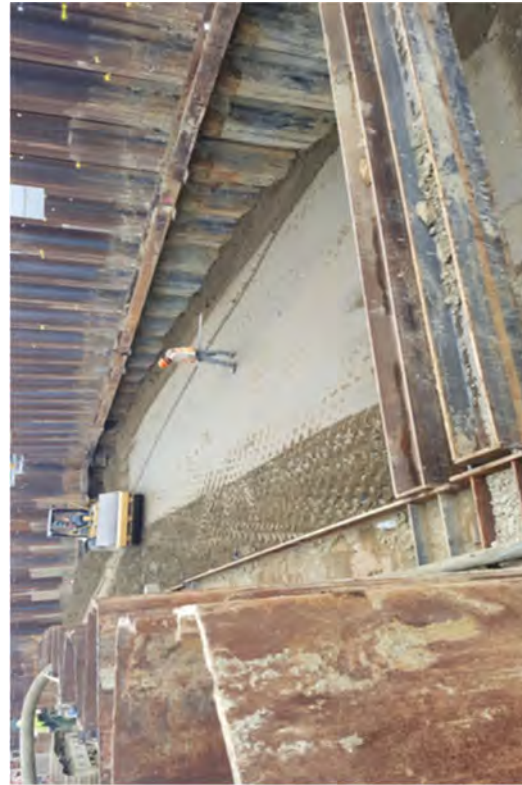
Compacting backfill.
