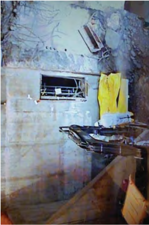
Preparing materials so they could be loaded out.
