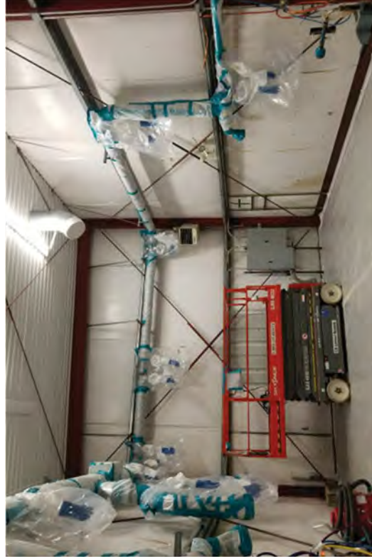
Ventilation removal prep.
