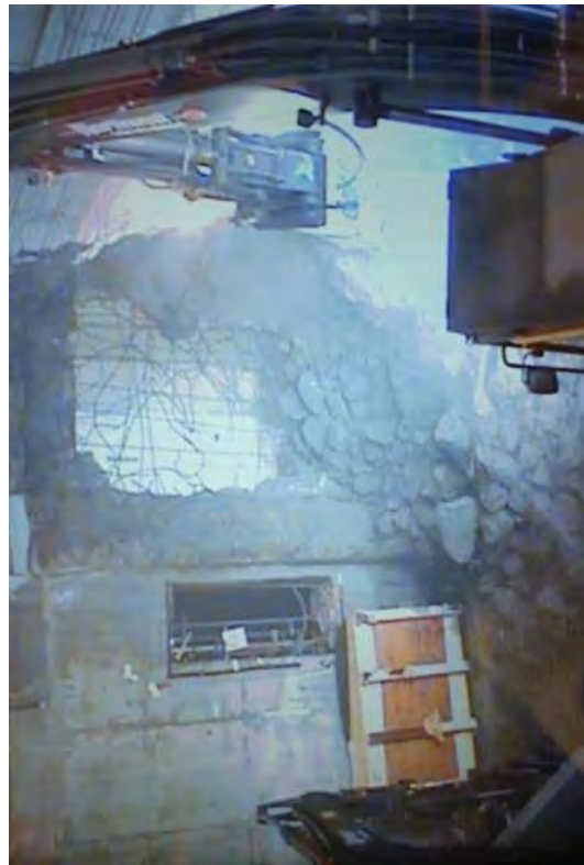
An excavator demolishing the LRW Concentrator roof and walls.
