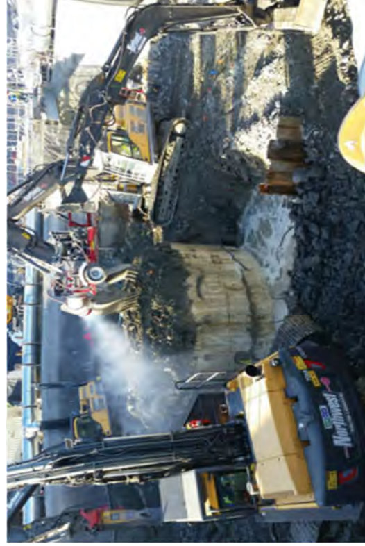
Backfilling the East Suppression Chamber.
