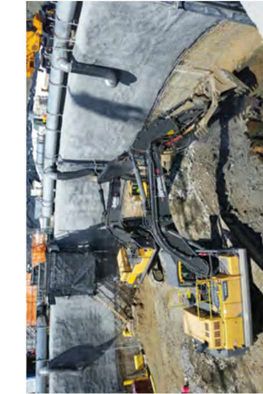
Demolishing SFP structural concrete at -14' EL to -18' EL.
