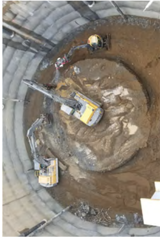
Demolishing concrete at -66' EL to -70' EL.
