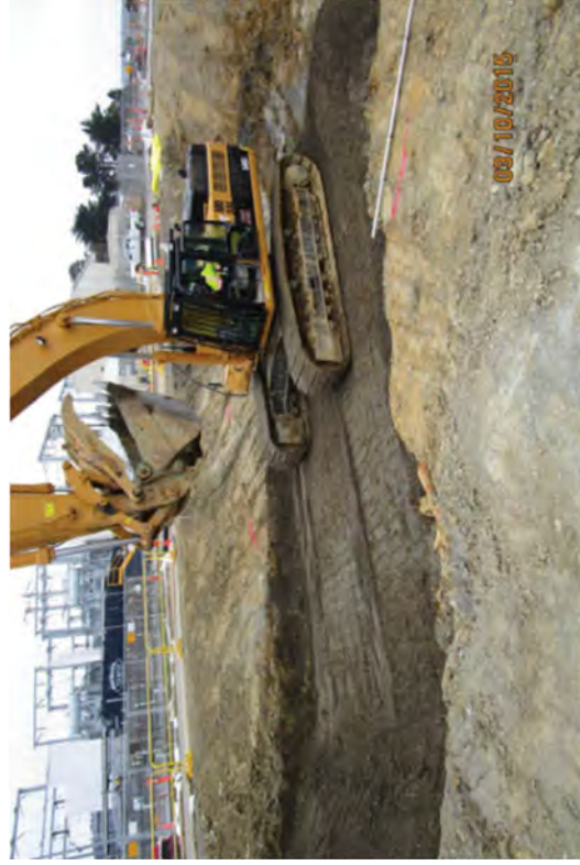
Compacting backfill using the methods of track walking and tamping with bucket.
