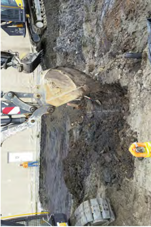
Removing pipe.
