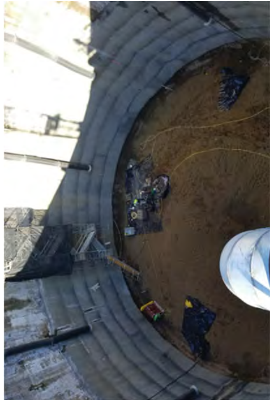
Grouting wells DW-2 and DW-3.
