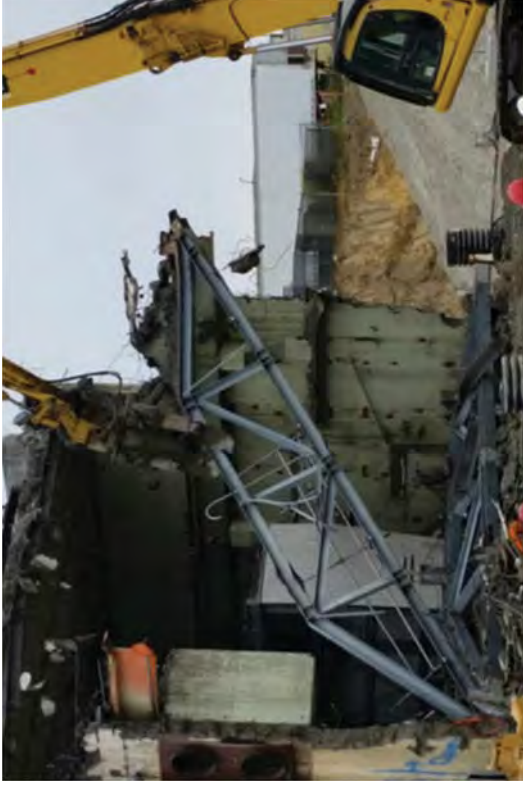
Staging the roof trusses within the RFB foot print.
