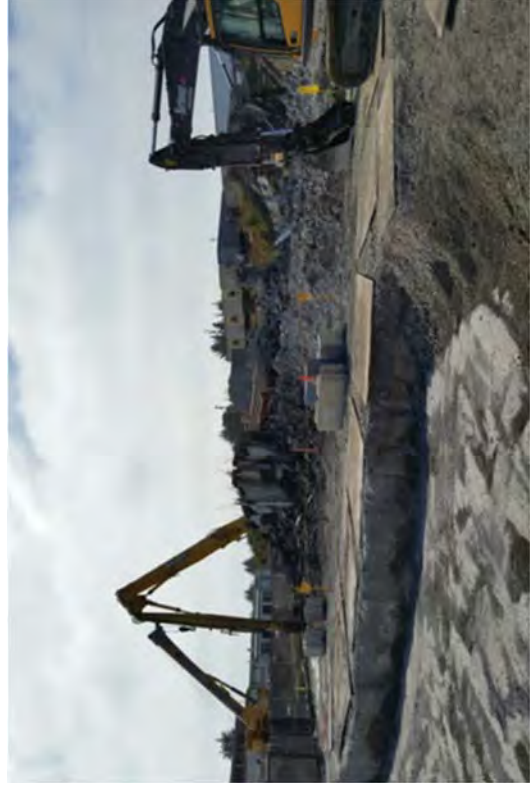
The RFB wall demolition completed.
