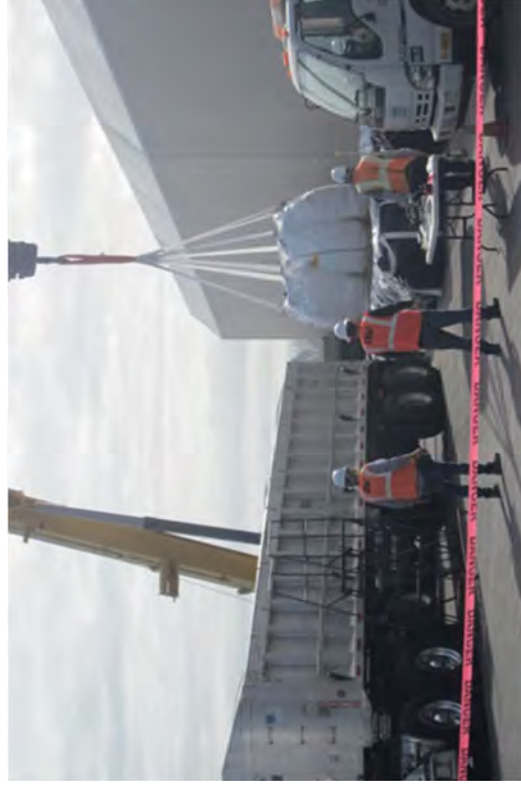
Loading trucks with IP-1 bags for shipment to Redding, CA to be loaded onto Gondola rail car.
