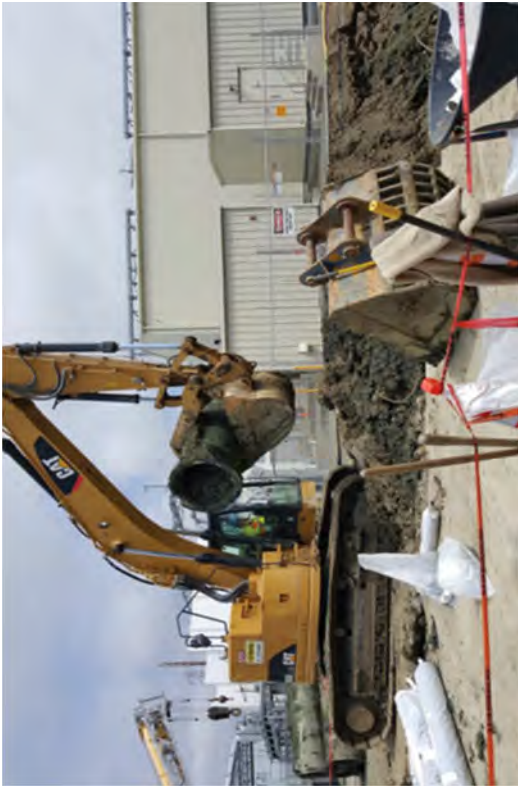
Removing commodities and piping.
