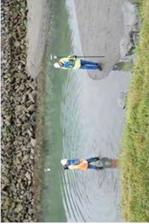
Workers were required to wear personal flotation devices and use a buddy system when working in or near water.
