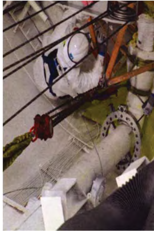
Setting up equipment to cut the feedwater line.
