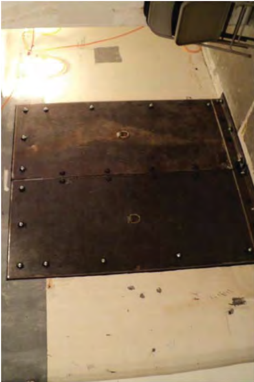
The access tunnel closed off with approved steel covers.
