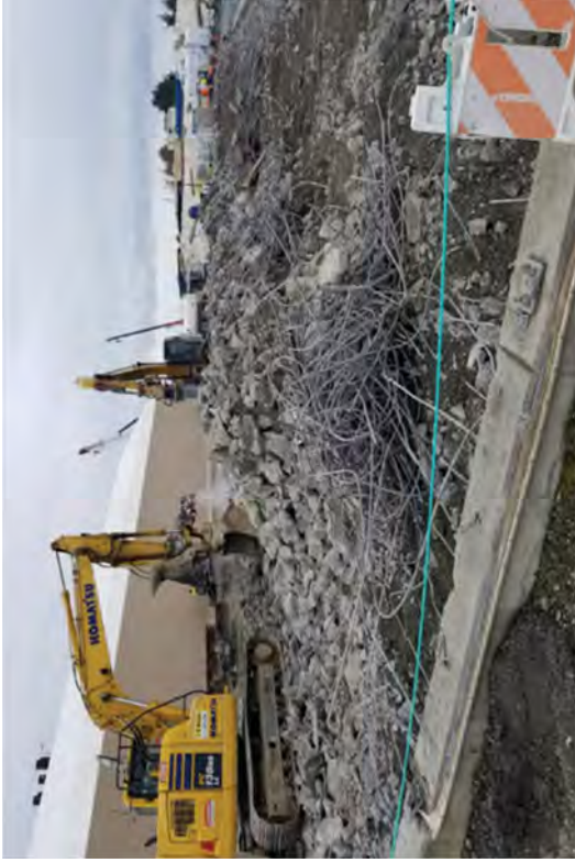
Stockpiling concrete and rebar from the SMF Tent 2 slab.
