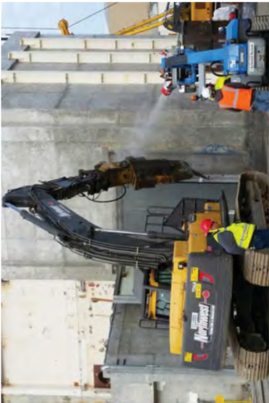
Demolishing the right outer railroad bay door.
