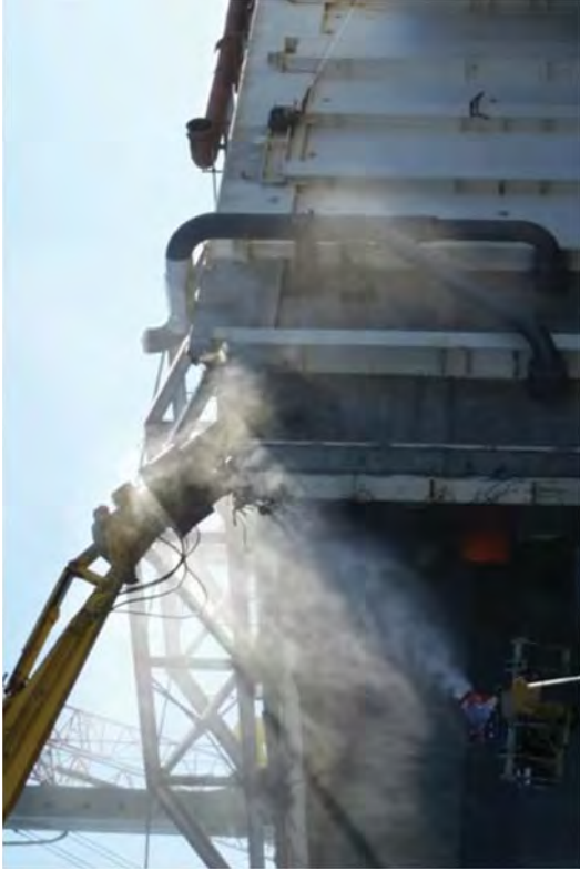
Processing the North Wall of the RFB.
