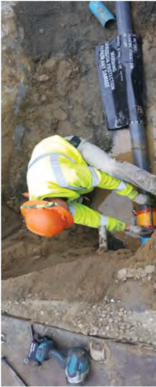
Performing the final connection to the site sewer system.
