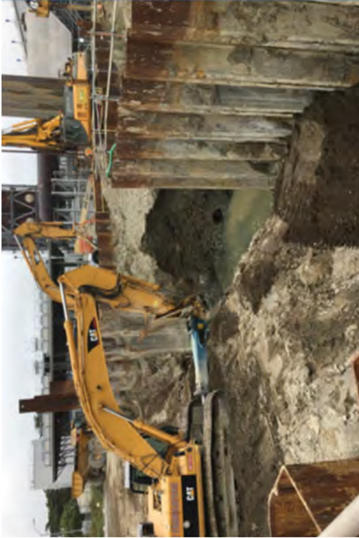
A hammer being used on the headwall.
