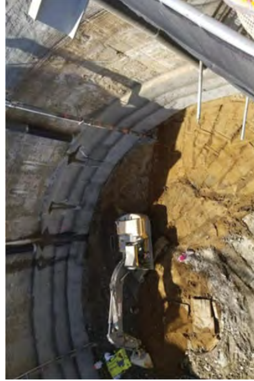
Removing material from the sacrificial layer at -52' EL.
