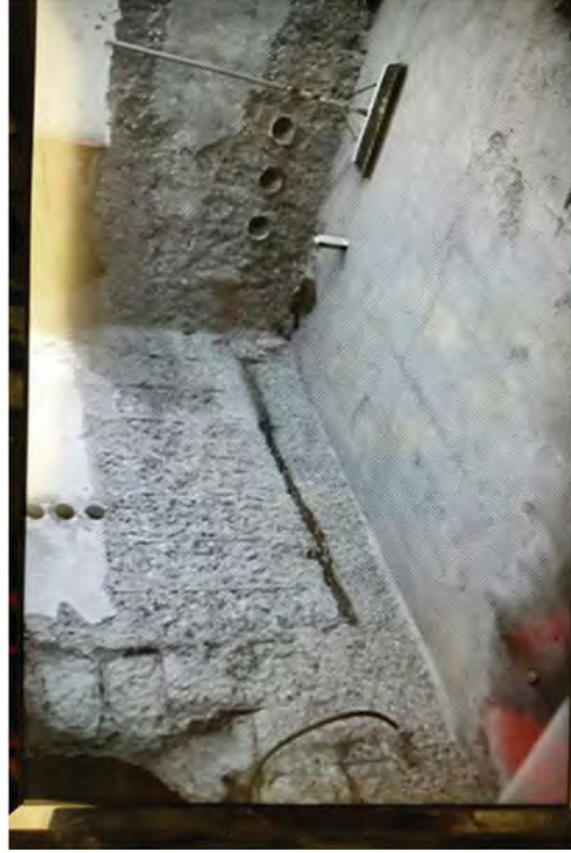
The concentrated waste tank after the scabbling was complete.
