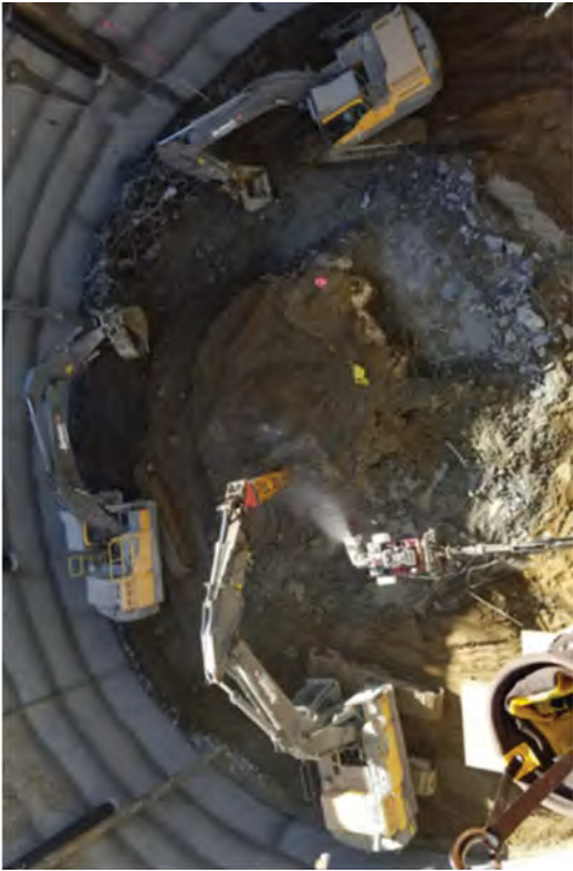
Demolishing concrete at -52' EL to -58' EL.
