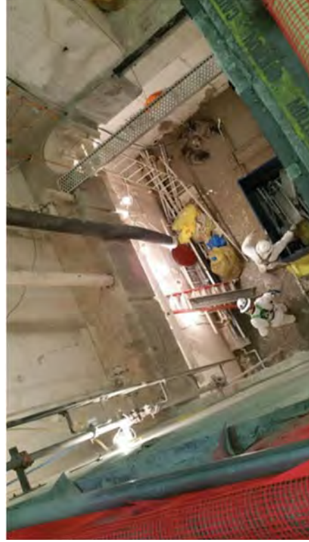
The TBDT removed.
