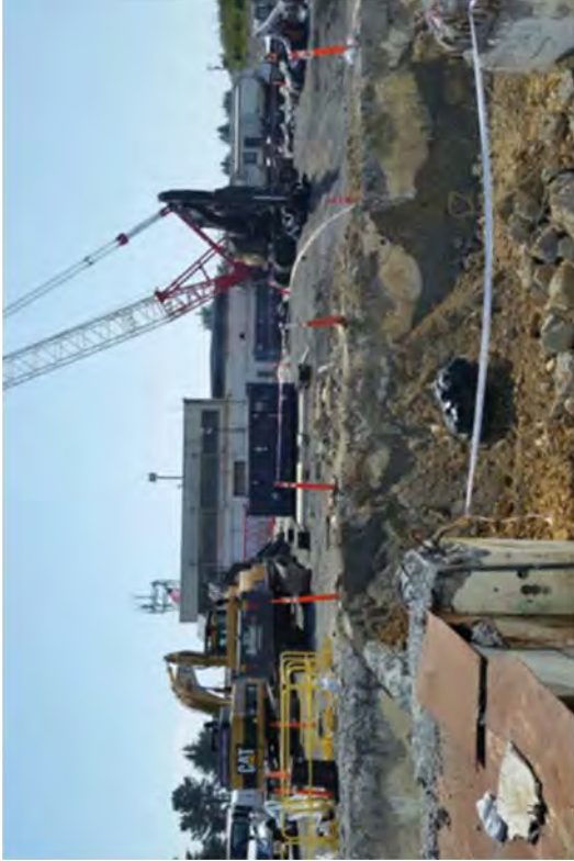
A scale and intermodal set-up to remove and process ACM debris.
