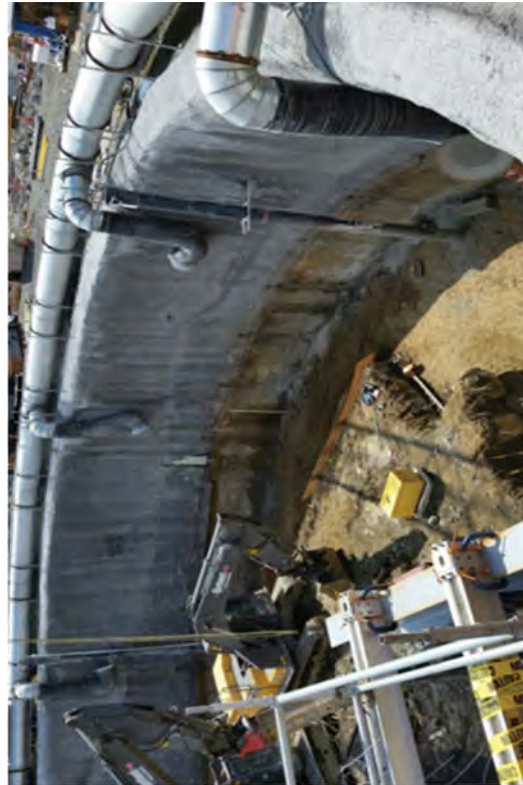
Installed WWF on the west side of the CSM wall.
