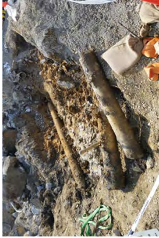
Cleaning up transite pipe debris and loading the ACM into intermodals.
