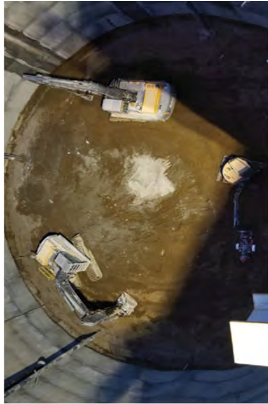
The Tremie completely removed.
