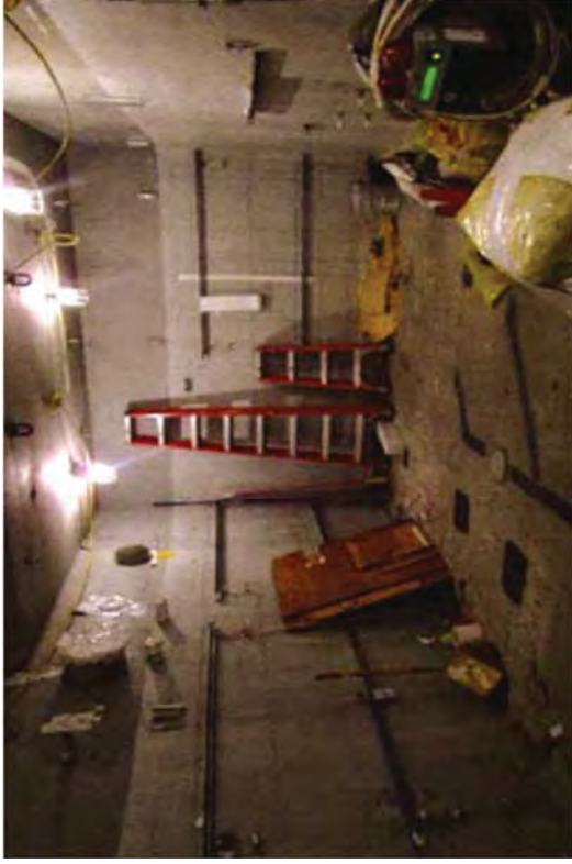
The heat exchanger room cleared out.
