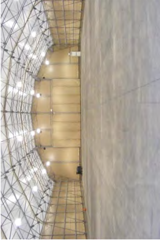
The finished interior of an SMF tent with lighting installed.
