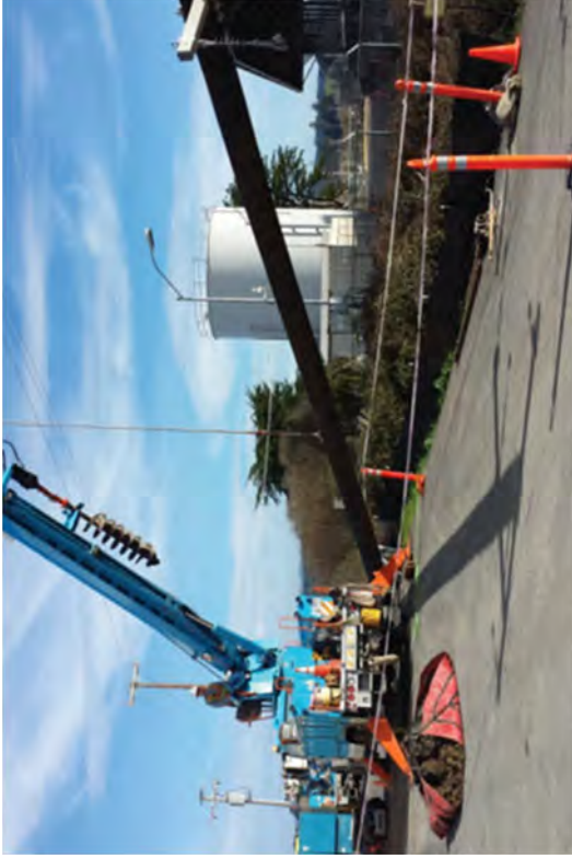
Mobilizing the GC Line and performing preparation activities such as drilling for and installing the pole anchors.
