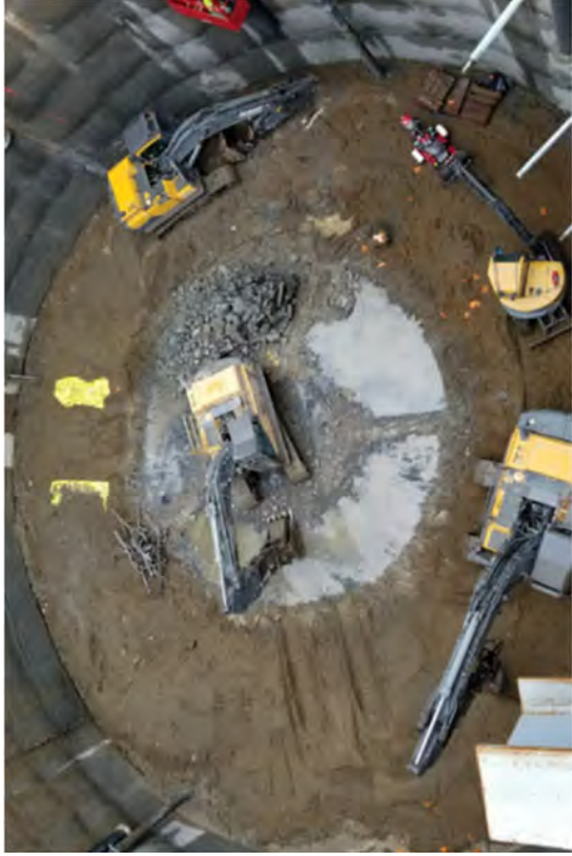
Removing the caisson floor slab.
