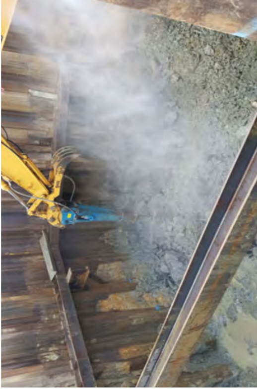
Removing the thrust block from Area C.
