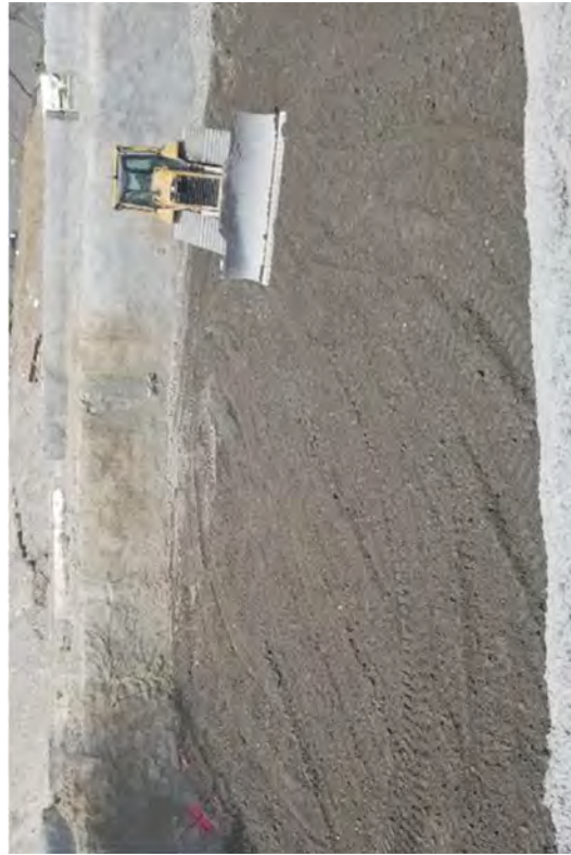
Concrete back fill leveling process
