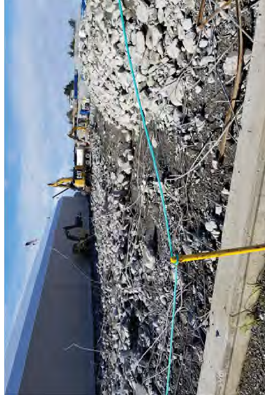
Stockpiling concrete and rebar from the SMF Tent 2 slab.
