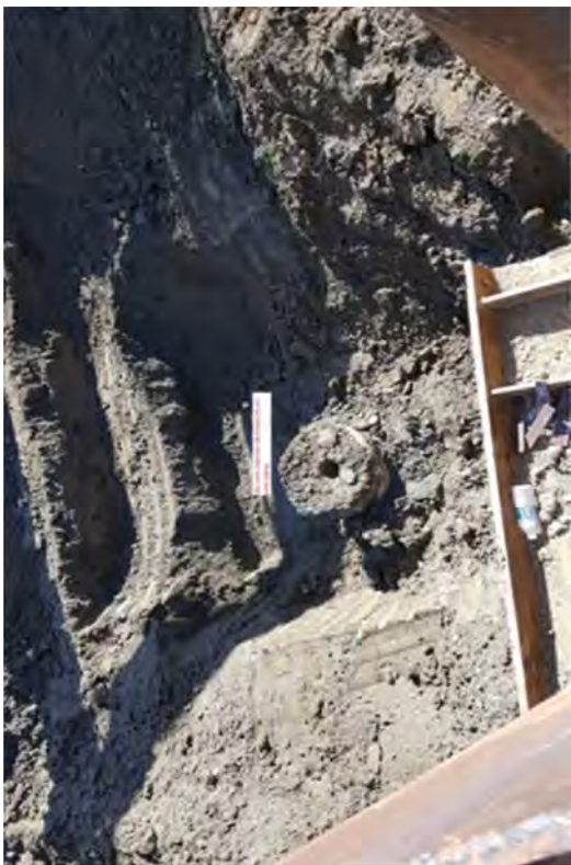
An OWS pipe line to outfall in Area C.
