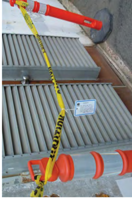
A caution area with its required information tag that gives the name of the area's owner and any specific instructions.
