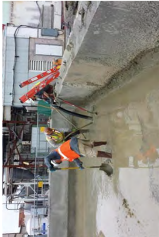
The CLSM Pond for CSM spoils.
