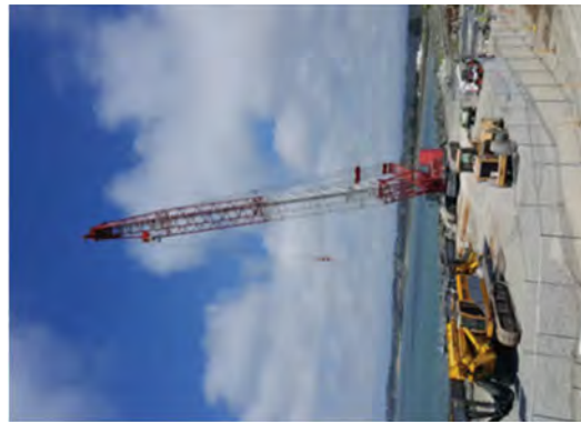
Staged cranes and materials to install sheet piles and a water supports.
