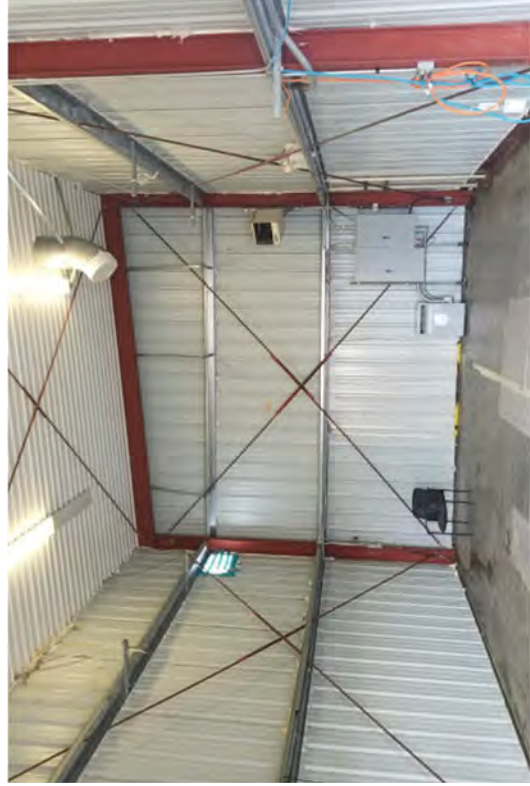
Building ready for FSS.
