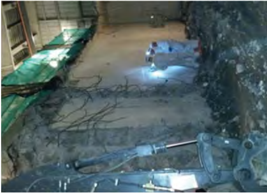
The concentrated waste tank wall opening layout and demolition
