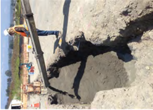
Filling a soft spot with CLSM after it was more extensively excavated than the immediate area surrounding it.
