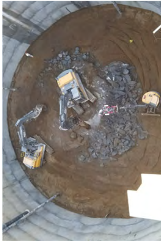
Removing the Tremie from -70' EL to -74' EL.
