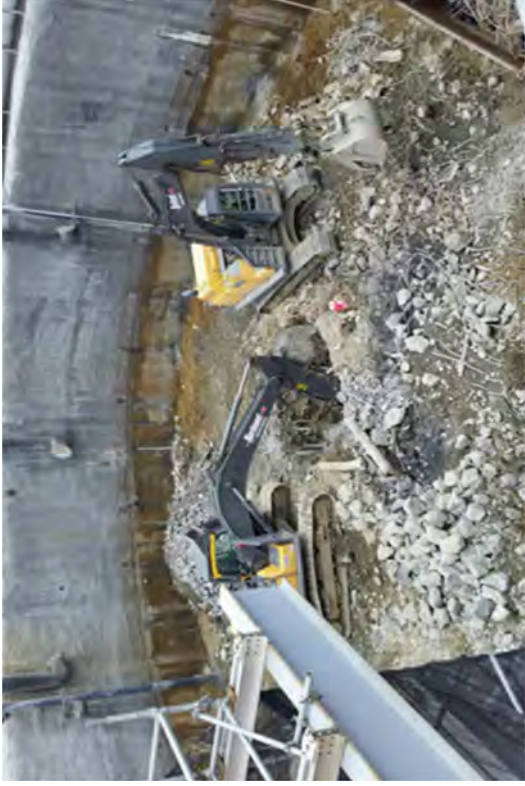
Removing Drywell to prepare for the activated region removal activities.
