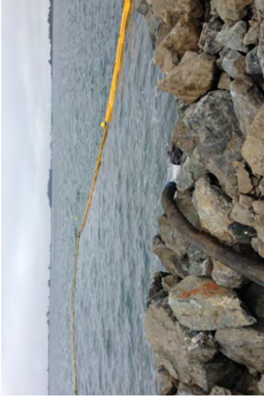
Pumping water from the Discharge Canal into Humboldt Bay. The yellow line is the Silt Curtain.
