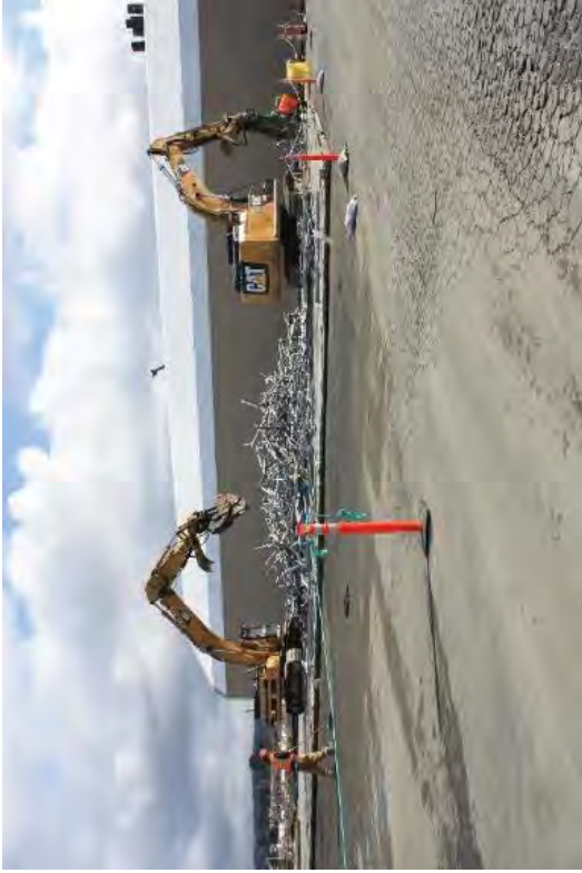
Processing steel from the SMF Tent 2.
