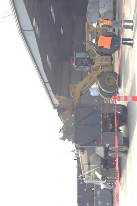
Loading concrete stored in WMF from the Intake Canal for transfer to a processor for re-use.
