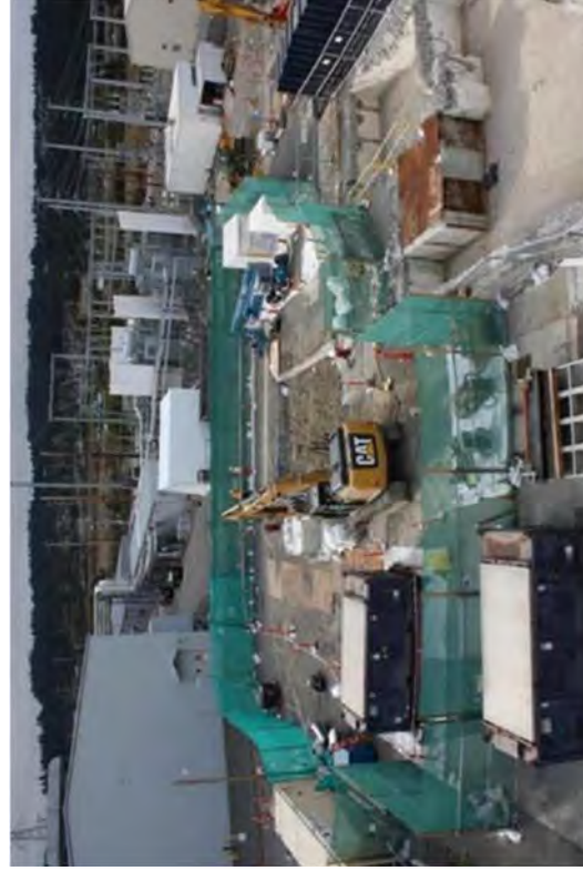
A HMS demolition safety person in a man basket keeping a mist of water on the demolition to control the risk of airborne asbestos and dust. The front of the HMS and CMU block above the overhead garage door opening and the roof deck were removed to provide access to the crane bridge seen on the ground inside the building.
