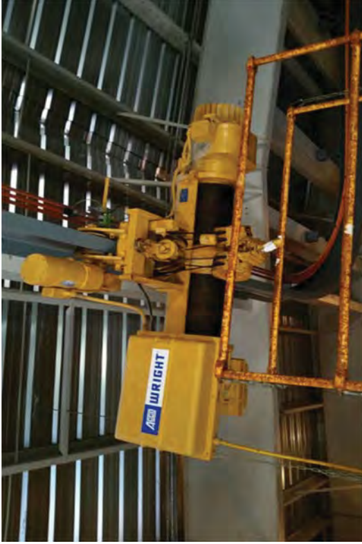
Decommissioning and draining oil from an overhead crane.
