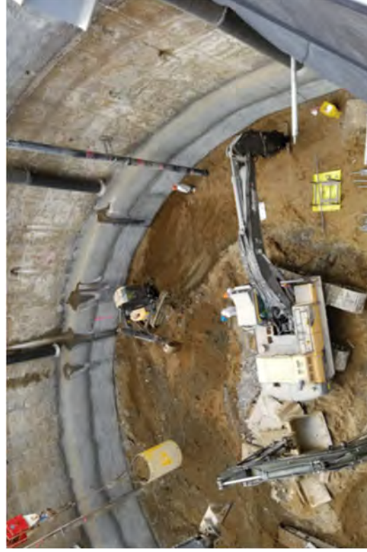
Loading out material from the sacrificial layer.
