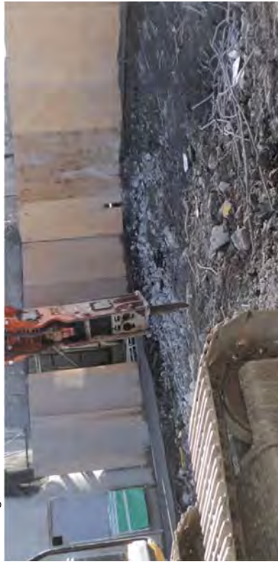
An excavator using the hammer to soften and penetrate the surface so that CLSM can penetrate after the final load out.
