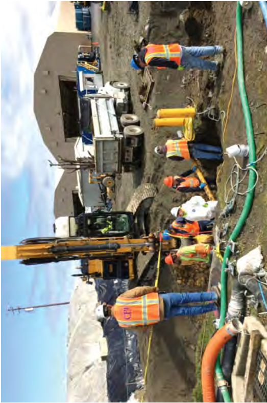
Crews sectioning out the LRW line.
