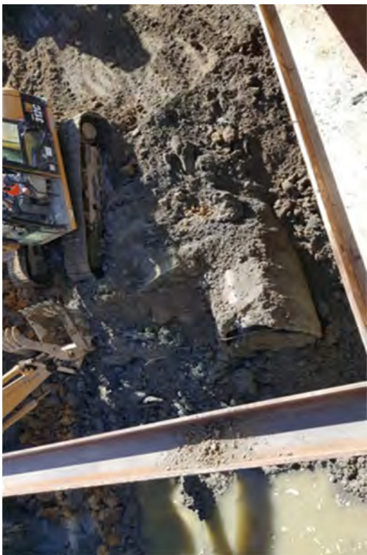
Pipe excavated for removal in Area C.
