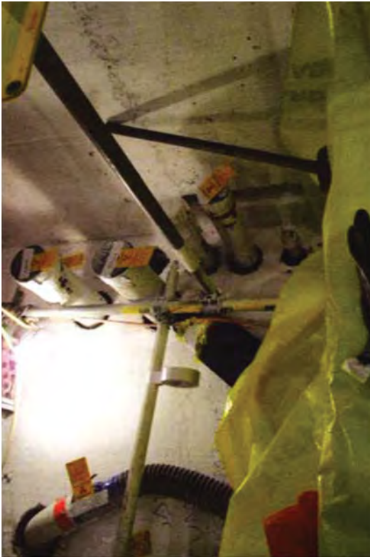
Pipes to that were to stay in-place are identified with tags.
