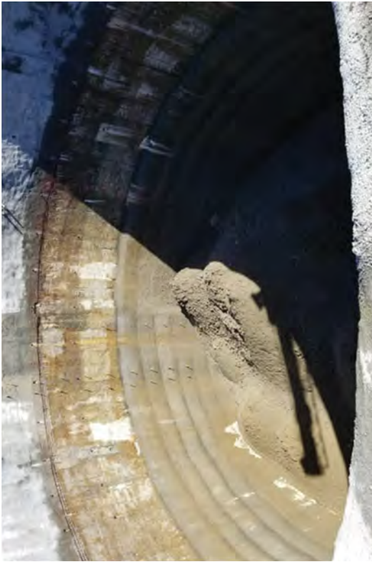
Continuing to backfill the Caisson.
