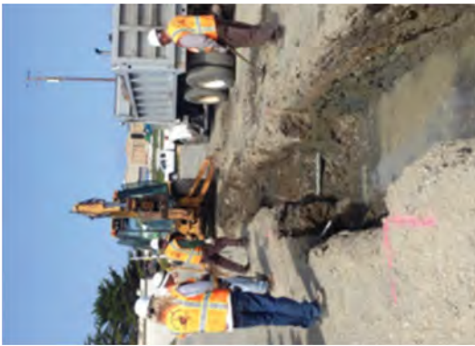
Filling a soft spot with CLSM after it was more extensively excavated than the immediate area surrounding it.
