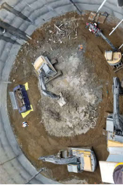
Loading out metal debris.
