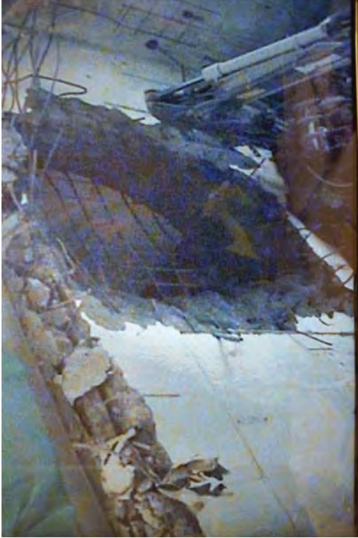
Demolishing the entrance opening to the resin disposal tank.
