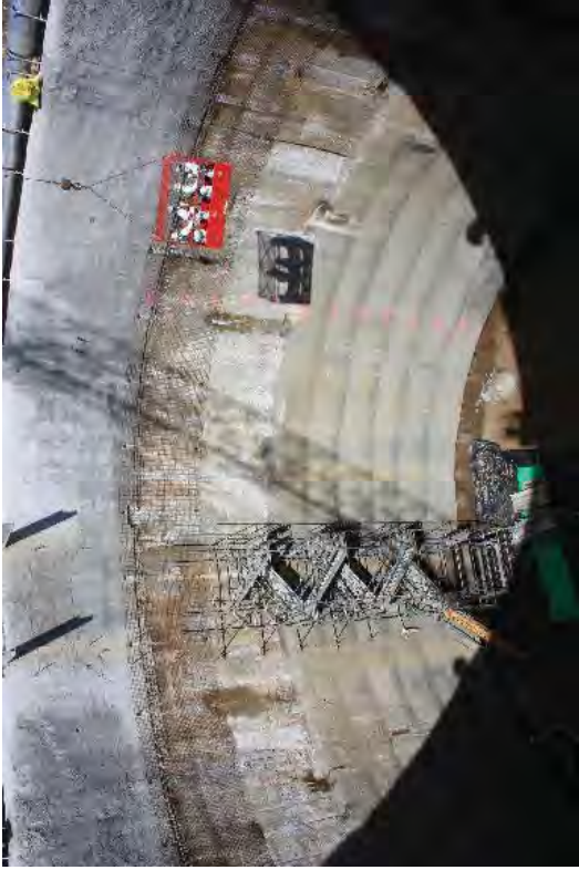
Stair tower crew exiting the caisson
