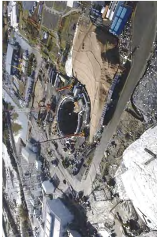
The site layout at completion of Caisson removal.
