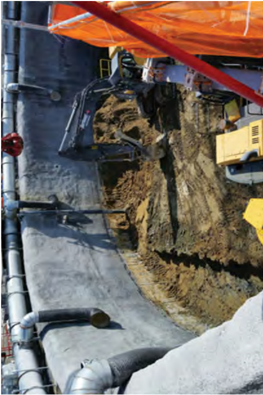
Caisson Excavation -10' EL to -14' EL
