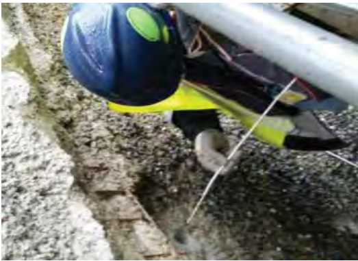
An engineering technician drilling and preparing anchor-bolt holes.
