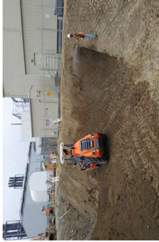
Continuing to backfill Area A.
