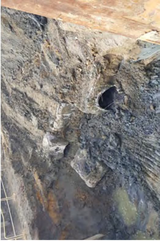
Circulating Water Lines Removal
