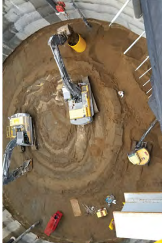
Excavating re-use soils from beneath the stairway at -70' EL.
