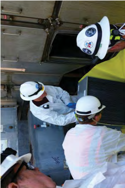
Removing MPEF HEPA filters.
