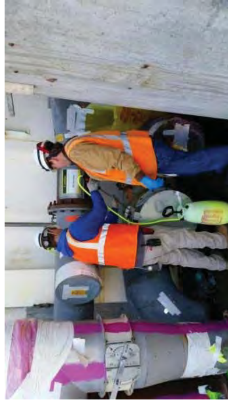
Applying fixatives.
