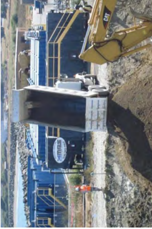
Unloading CSM Spoils from GARDIAN into the Canal.
