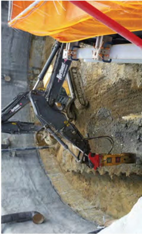
Demolishing SFP structural concrete at -14' EL to -18' EL.
