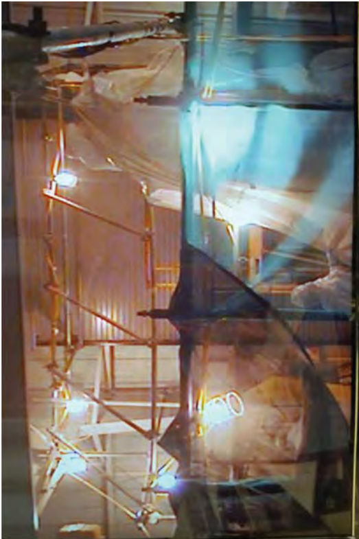
Removing the containment measures from the interior of the LRWB.
