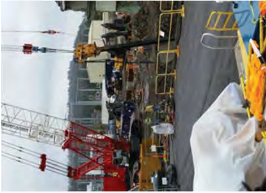
Removing H-Piles.
