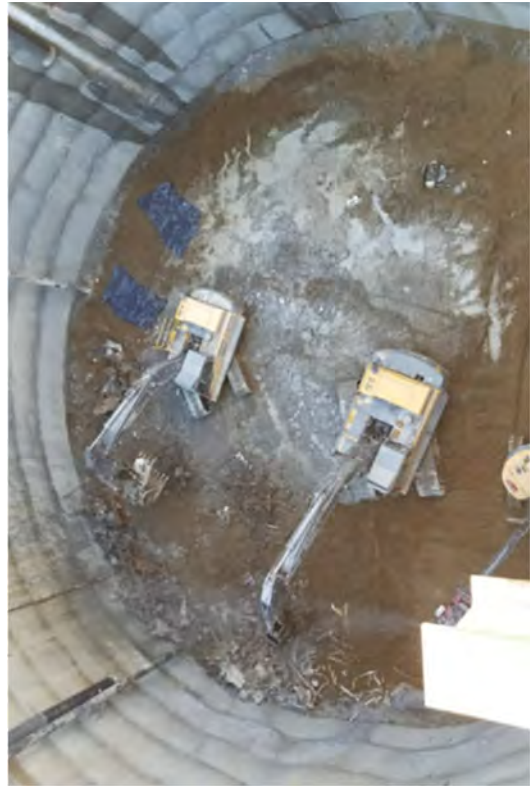
Shearing apart and loading out steel debris.
