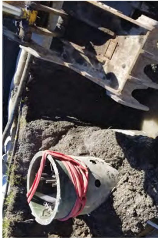
Lift station removal.
