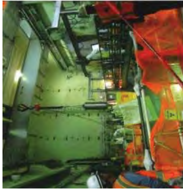
Lifting the solids collection filter from the SFP before plugging its drain and moving it to the decontamination and wrapping area.
