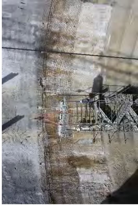
Scaffold materials being removed from Caisson
