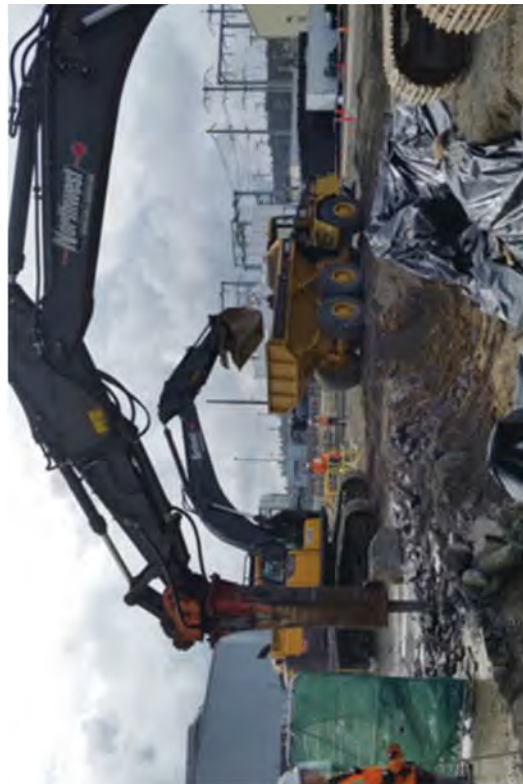
Removing the Feed Pump slab and footings.
