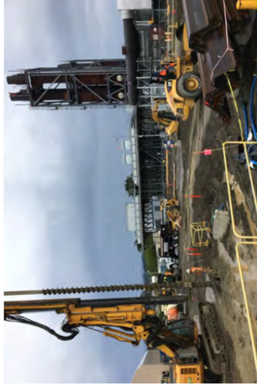
Continuing to pre-drill for the west sheet pile wall.
