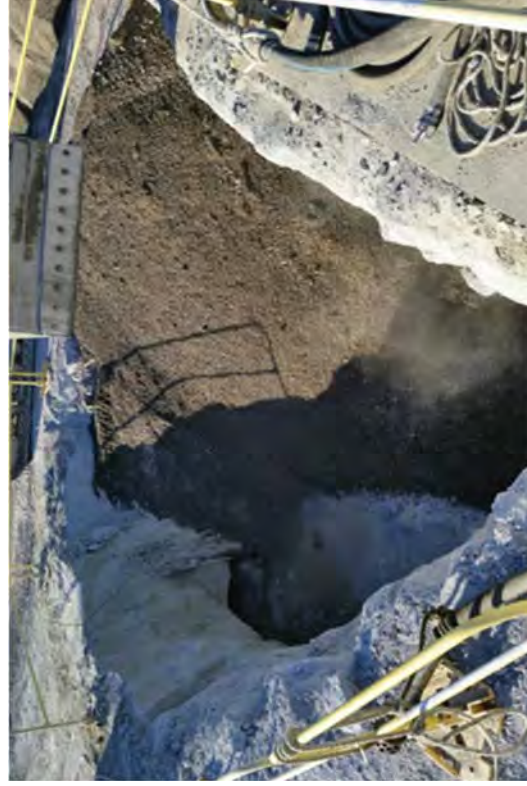
The interim backfill of the FSS deep feature excavation.
