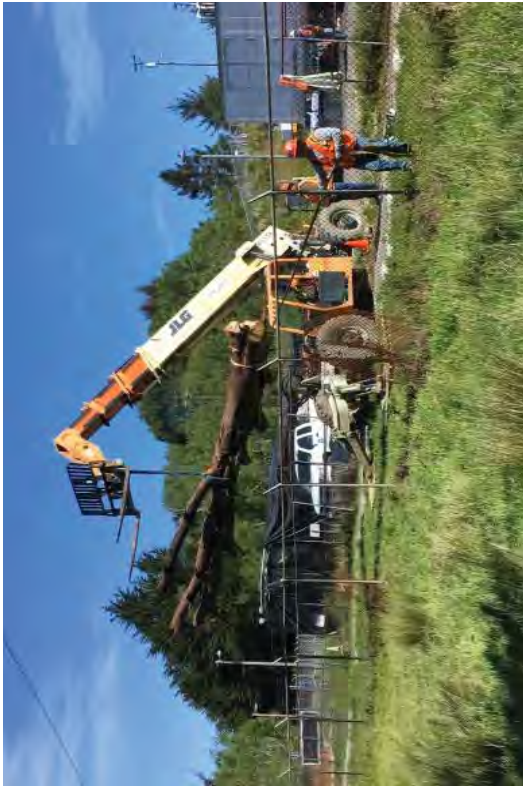
Snag features recovered from the site for Intake Canal restoration.
