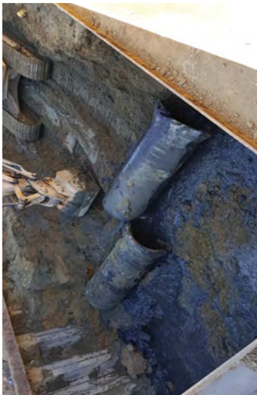
Removing pipe in Area C.
