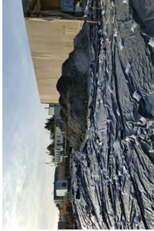
Soils stockpiled in the Upper Yard for re-use after being scanned with the GARDIAN.
