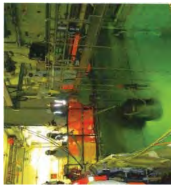
Removing the demineralizer from SFP.
