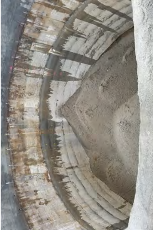
Backfilling the Caisson.
