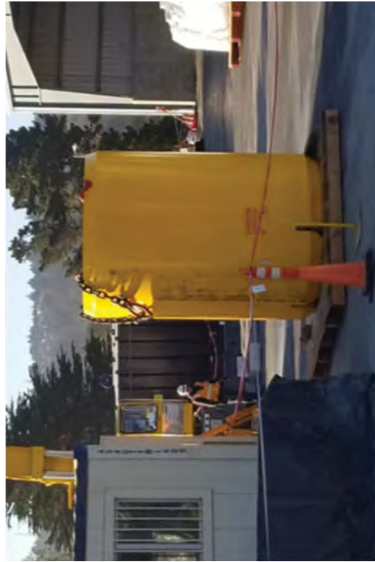
A new and larger muck bucket.
