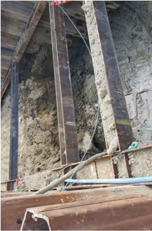
A water installed on Area C sheet piles.
