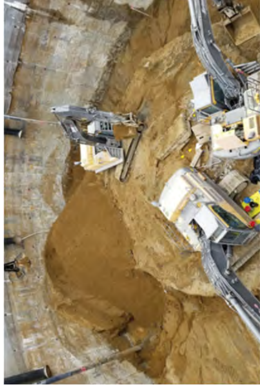
Removing soil from -34' EL to -40' EL
