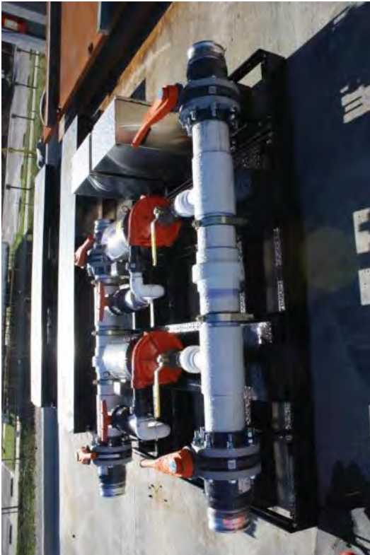
The new skid for the relocated receiver tank.
