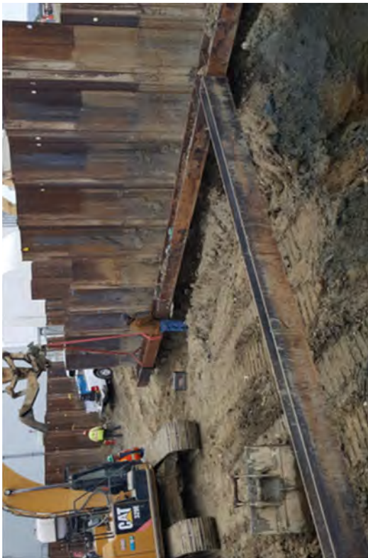
Installing walers in Area C.
