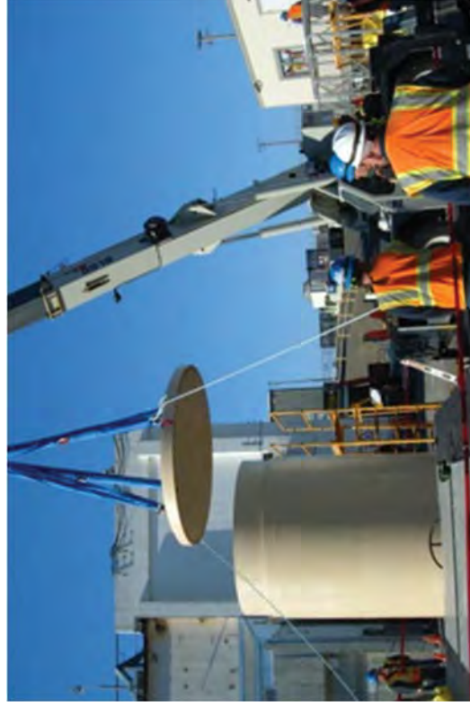
Tag lines were always used and required on lifted loads to prevent unwanted movement.
