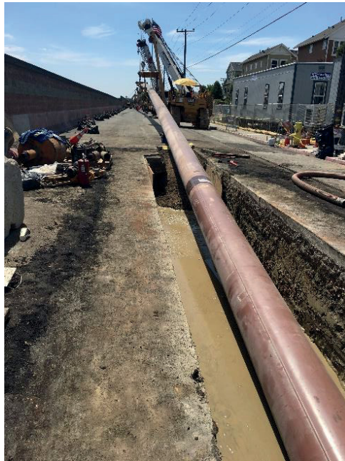
Figure 29 – Vintage Pipe Replaced in San Mateo
