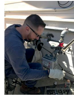
Figure 19 – PG&E Employee Working on CCE
