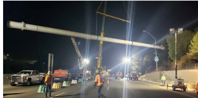
Figure 15 – Transmission Pipe L-153 Span Removed From I-880
