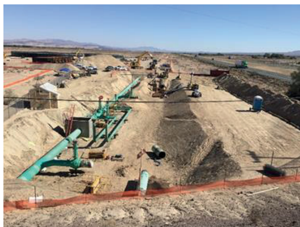
Figure 28 – Strength Test in Progress
