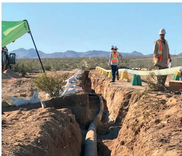
Figure 33 – Pipeline Replacement after the July Ridgecrest Earthquake
