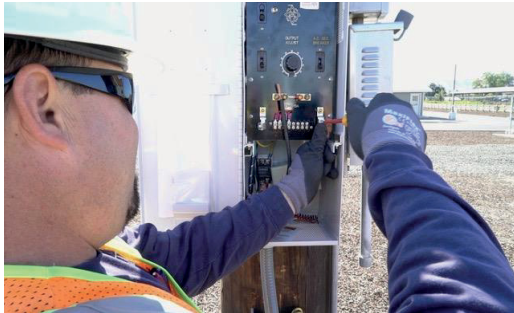
Figure 32 – PG&E Employee Installing a Cathodic Protection Rectifier
