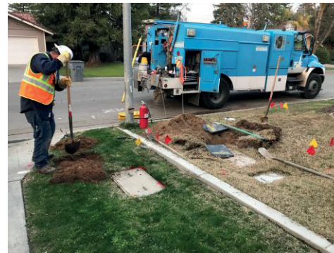
Figure 34 – PG&E's Maintenance & Construction Crew at Work
