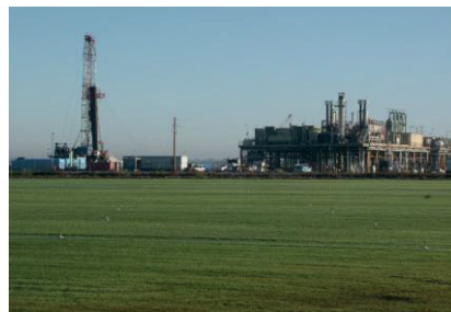
Figure 13 – Rig and Well Platform
