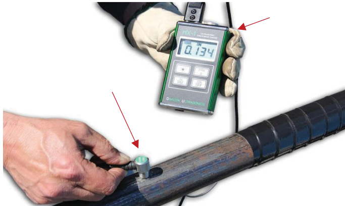
Figure 1. Checking Pipeline Wall Thickness
