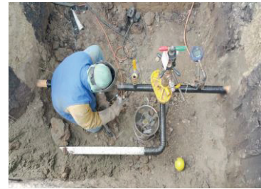
Figure 18 – Employee Working on Distribution Service
