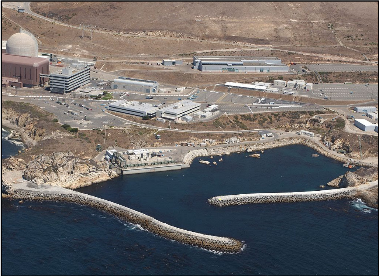
Figure 3. Intake Structure and Breakwaters/Marina
