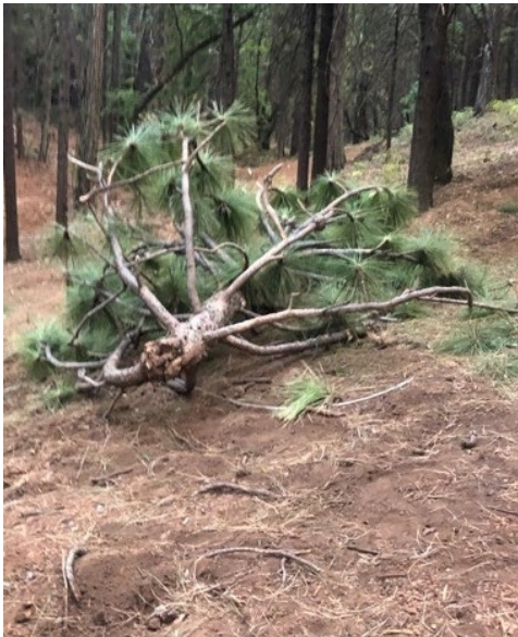
Figure 12: Image of Vegetation Related Damage in Butte County – Falling Treetop Damaged Overhead Conductor
