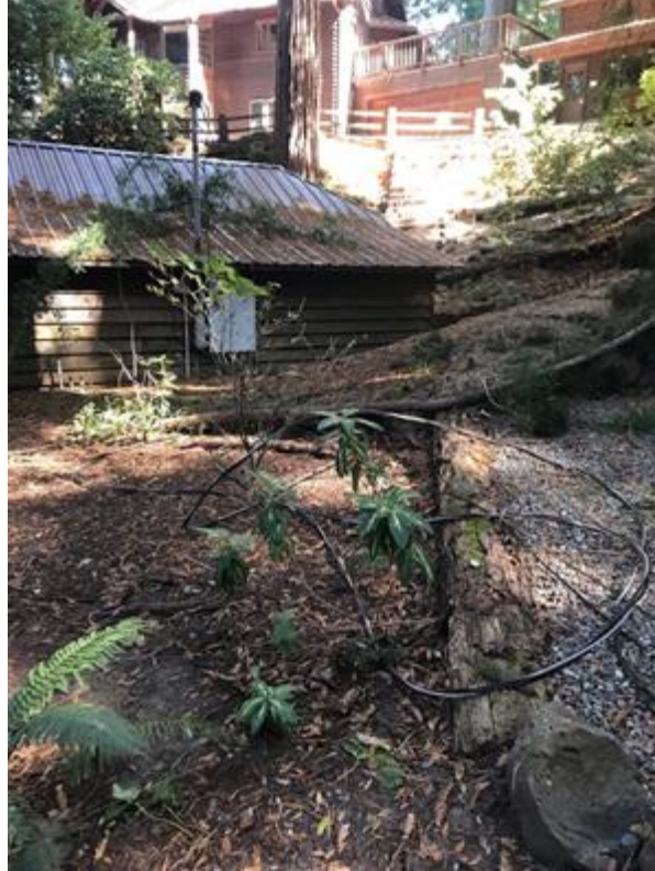
Figure 1 – In Los Gatos, Santa Clara County Branch Fell Onto Secondary Conductor Bringing Down the Lines
