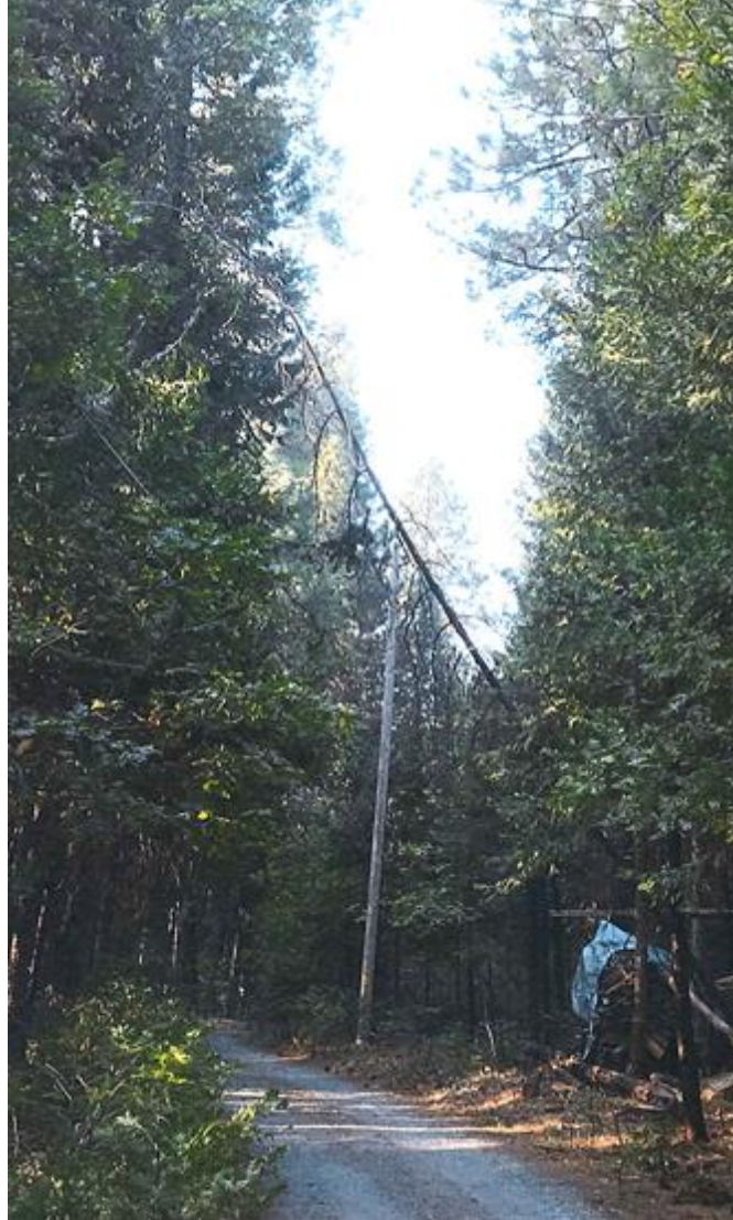
Figure 17 – In Georgetown, El Dorado County Branch in Contact With Primary Conductors
