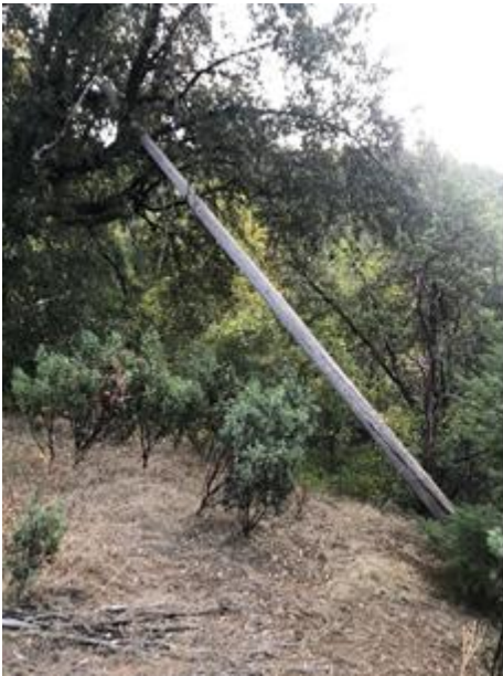
Figure 8 – In Unincorporated area of Shasta County Tree Failed Onto Primary Conductors and Took Down Pole
