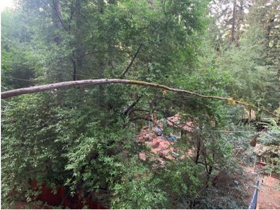
Figure 15 – Near Ben Lomond, Santa Cruz County Branch Failed Into Primary Conductors
