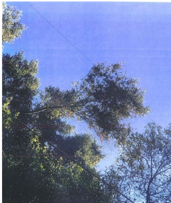
Figure 10 – In Kelseyville, Lake County Branch Fell Onto Primary Conductors
