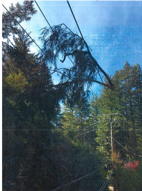
Figure 14 – In an unincorporated area of San Mateo County Branch Flew Onto Primary Conductors
