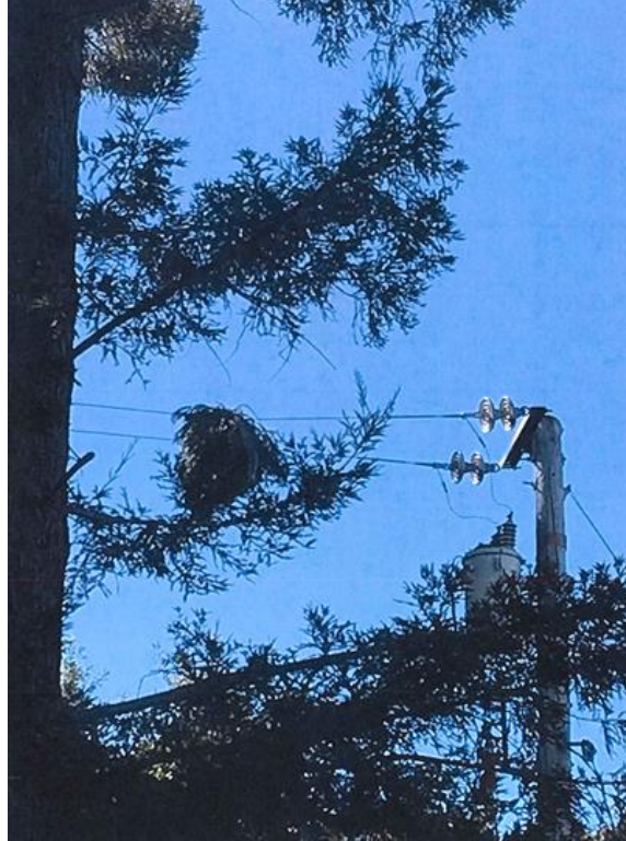
Figure 14 – In an unincorporated area of San Mateo County Branch Flew Onto Primary Conductors
