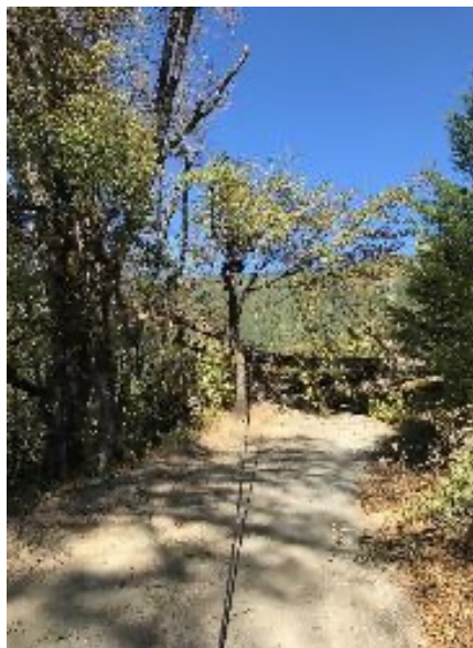
Figure 17: Vegetation-Caused Damage in Trinity County – Tree Fell and Broke Pole
