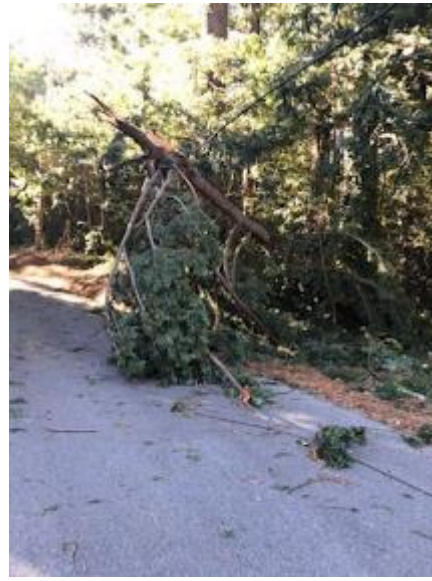
Figure 15: Vegetation-Caused Damage in San Mateo County – Broken Pole, Wire Down, Fallen Tree
