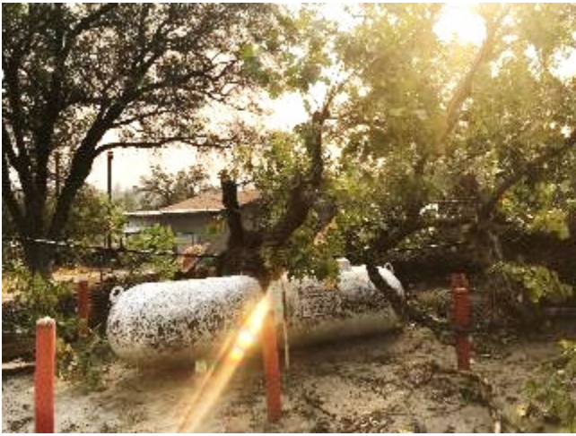
Figure 19: Vegetation Related Damage in Madera County – Tree Fell, Broke Neutral Conductor
