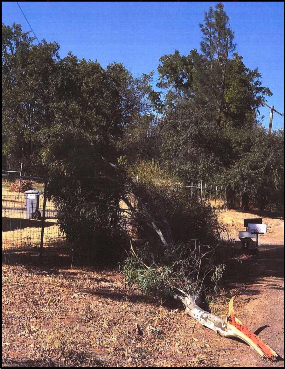
Figure 4: Tree fell, broken conductors; Unincorporated area of Butte County
