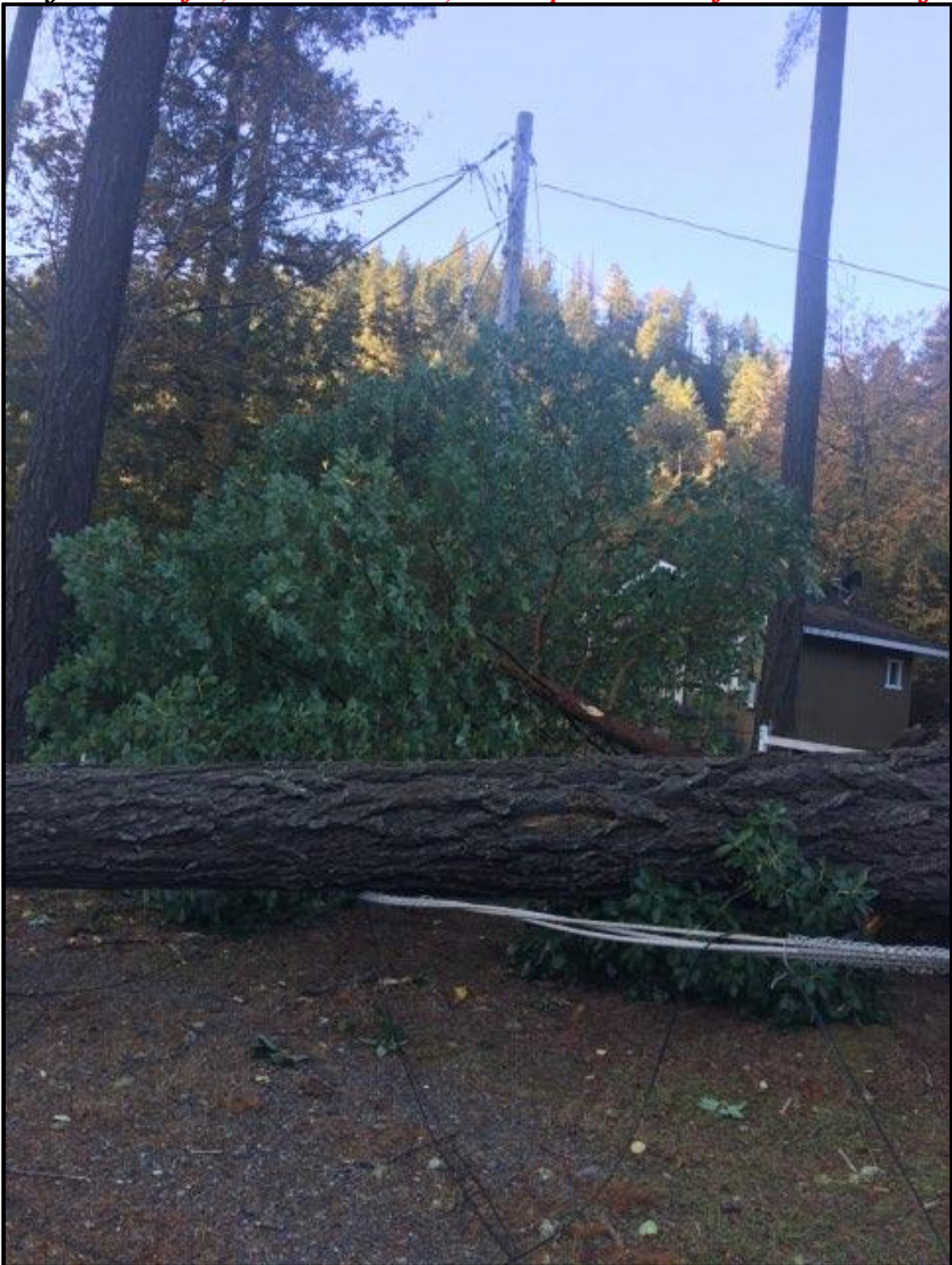
Figure 2: Tree fell, conductors broken; Unincorporated area of Humboldt County
