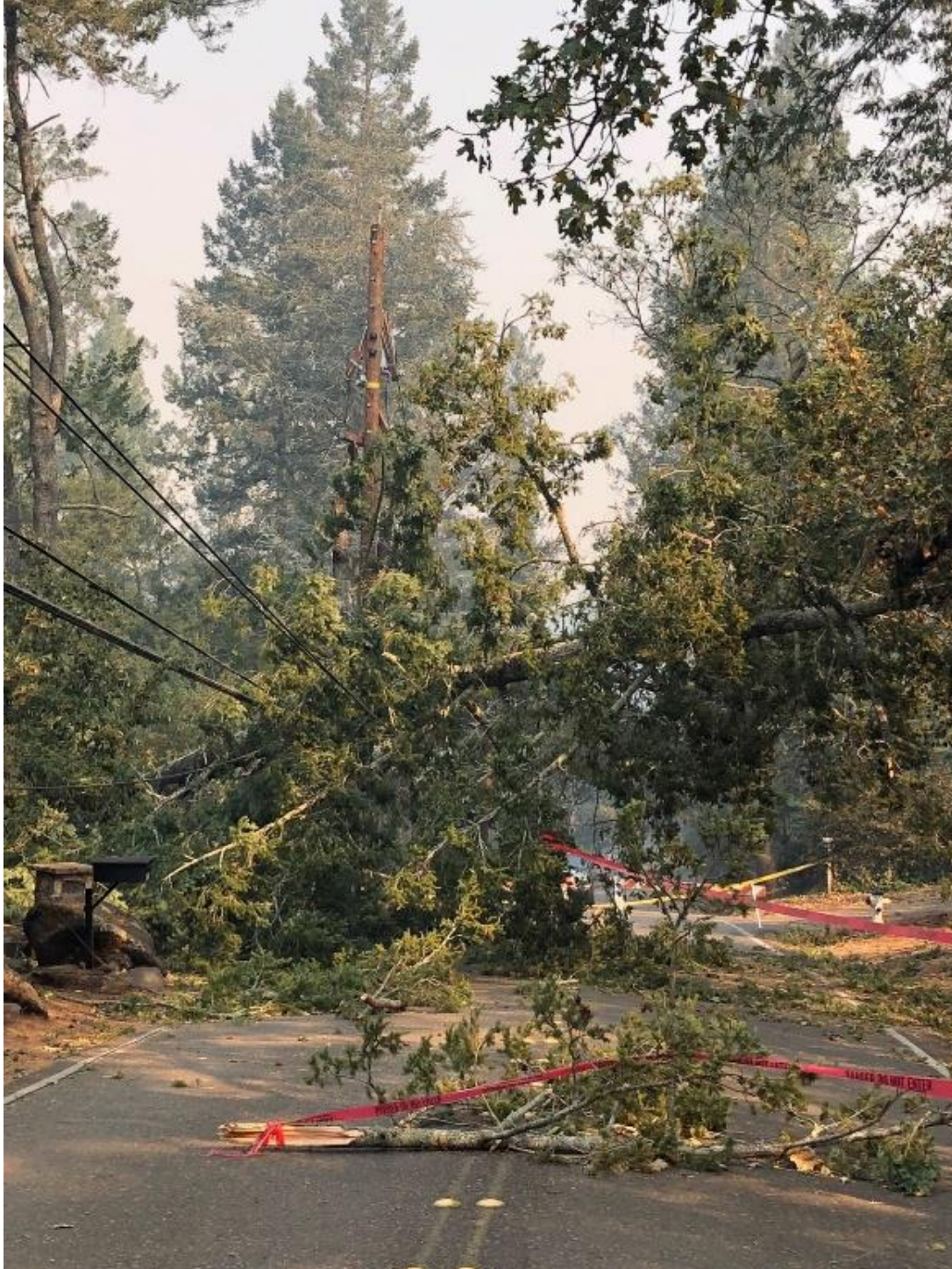
Figure 3: Tree fell, broken conductors; Unincorporated area of Sonoma County
