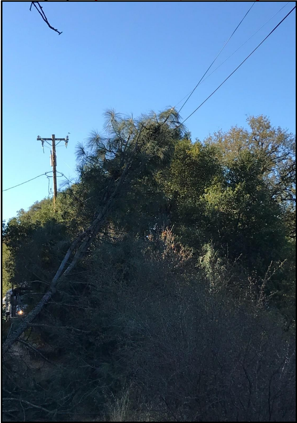
Figure 5: Tree fell onto conductors; Clearlake, County
