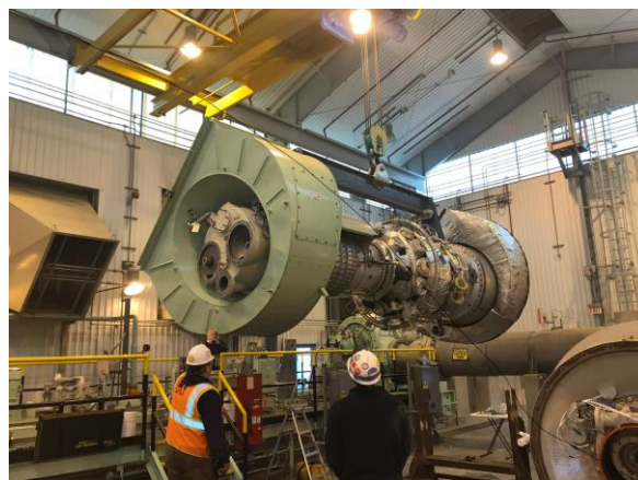
Figure 17 – Delevan Compressor Station Turbine Exchange
