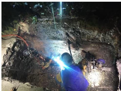
Figure 39 – PG&E’s Maintenance & Construction Crew at Work
