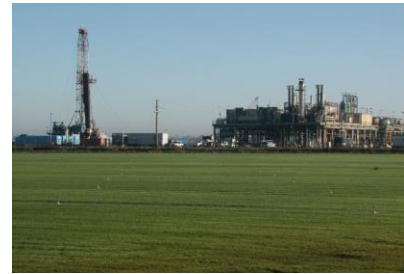
Figure 16 – Rig and Well Platform
