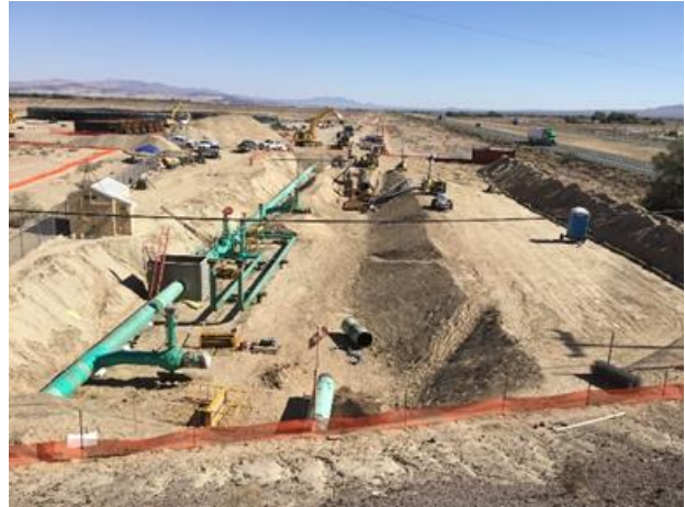
Figure 34 – Strength Test in Progress
