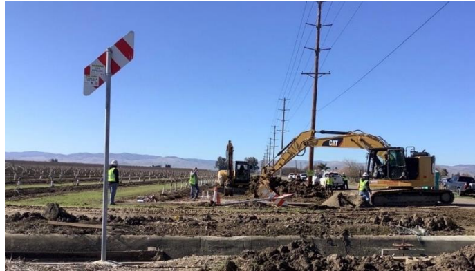
Figure 30 – Pipeline Marker Near Excavation Site
