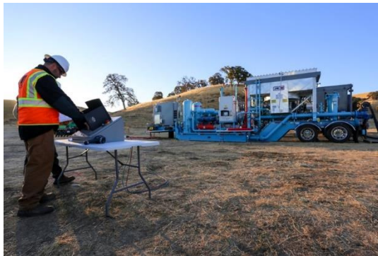
Figure 23 – Portable Cross Compression Degassing Isolated Segment of Pipeline into Adjacent Line
