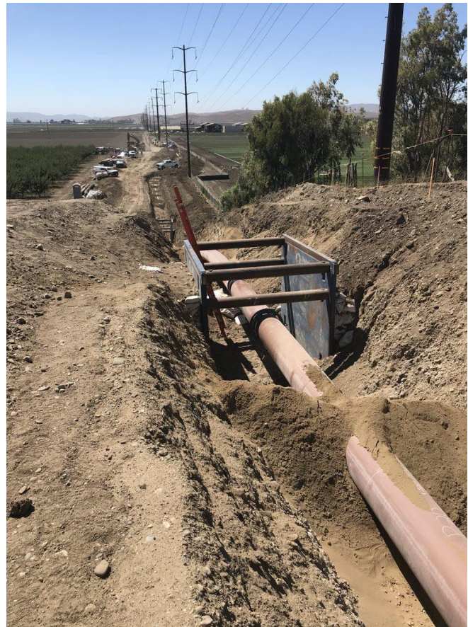
Figure 38 – L-301A Fault Crossing Pipe Replacement
