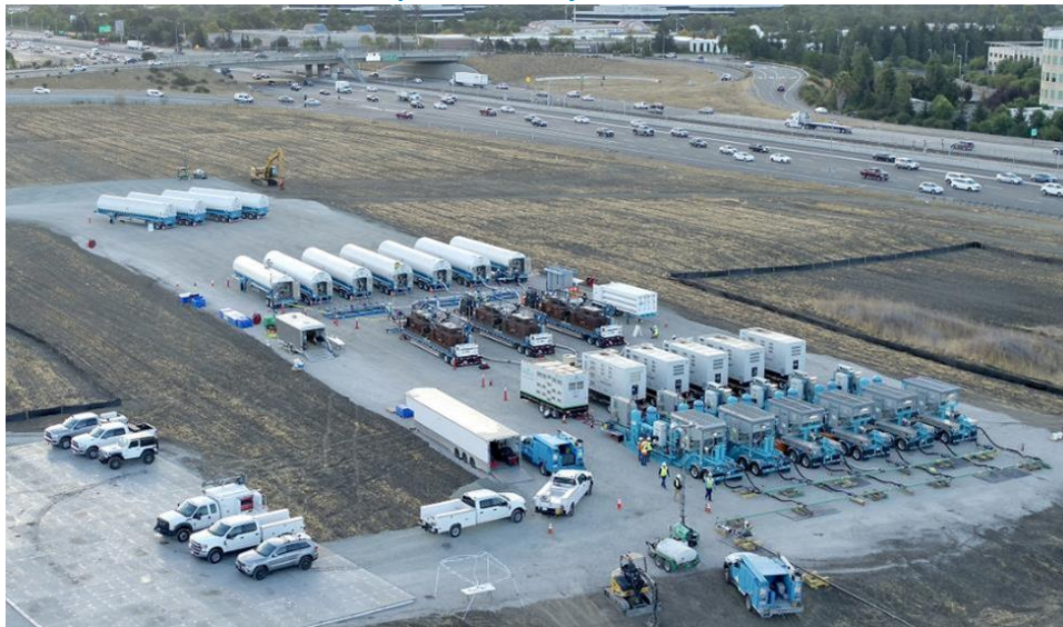
Figure 24 – A Large-scale LNG injection Site in Dublin, CA supporting a planned gas outage
