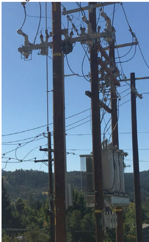
Figure 12 Shoofly installed outside fence at Calistoga substation
