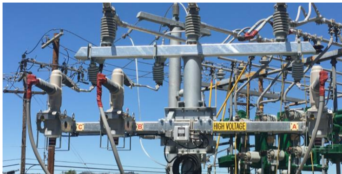
Figure 19 3-phase Viper recloser on GFN riser
