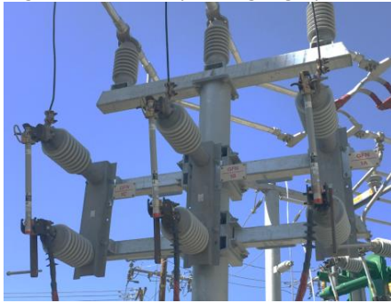
Figure 18 Fused cutouts on GFN riser
