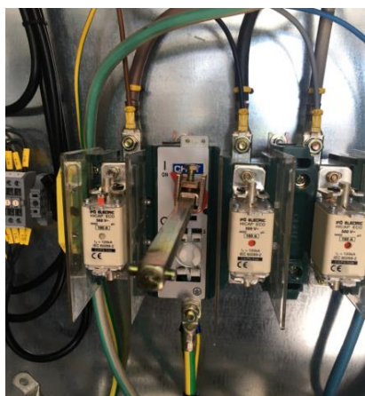
Figure 15 L1 fuse supplying RCC inverter blew
