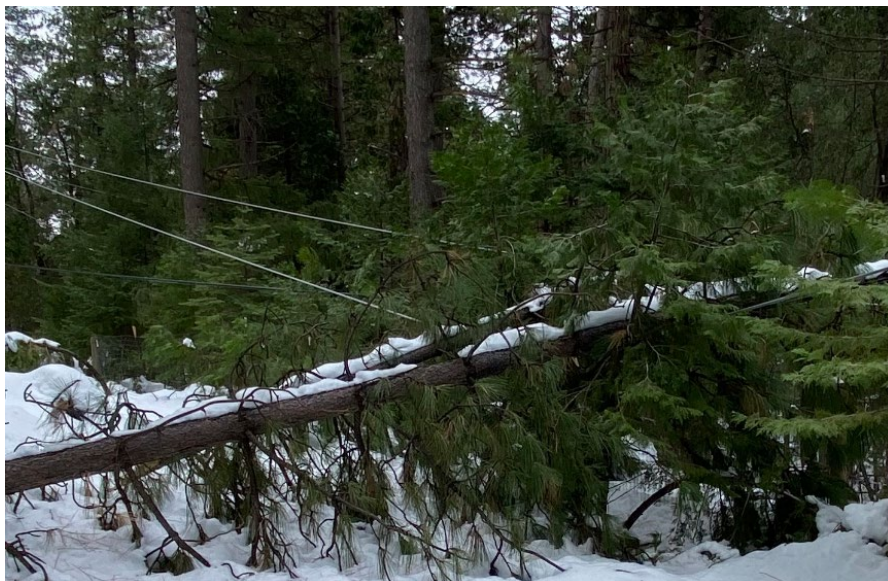
FIGURE PG&E-22-11-3: COVERED CONDUCTOR EFFECTIVENESS – EXAMPLE 3
