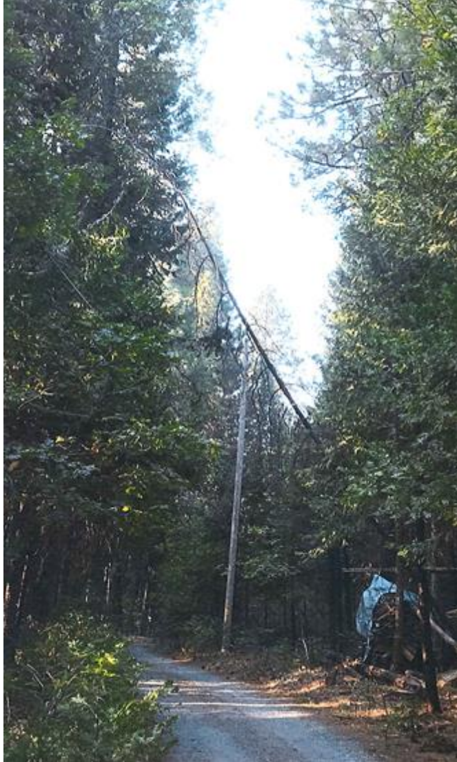
Figure 11 – In Georgetown, El Dorado County Branch in Contact With Primary Conductors
