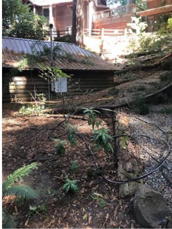
Figure 1 – In Los Gatos, Santa Clara County Branch Fell Onto Secondary Conductor Bringing Down the Lines
