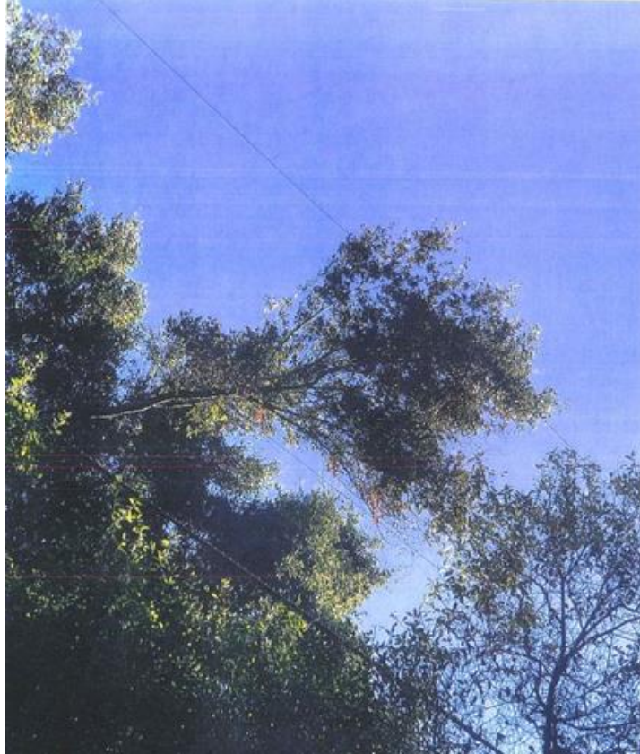
Figure 7 – In Kelseyville, Lake County Branch Fell Onto Primary Conductors
