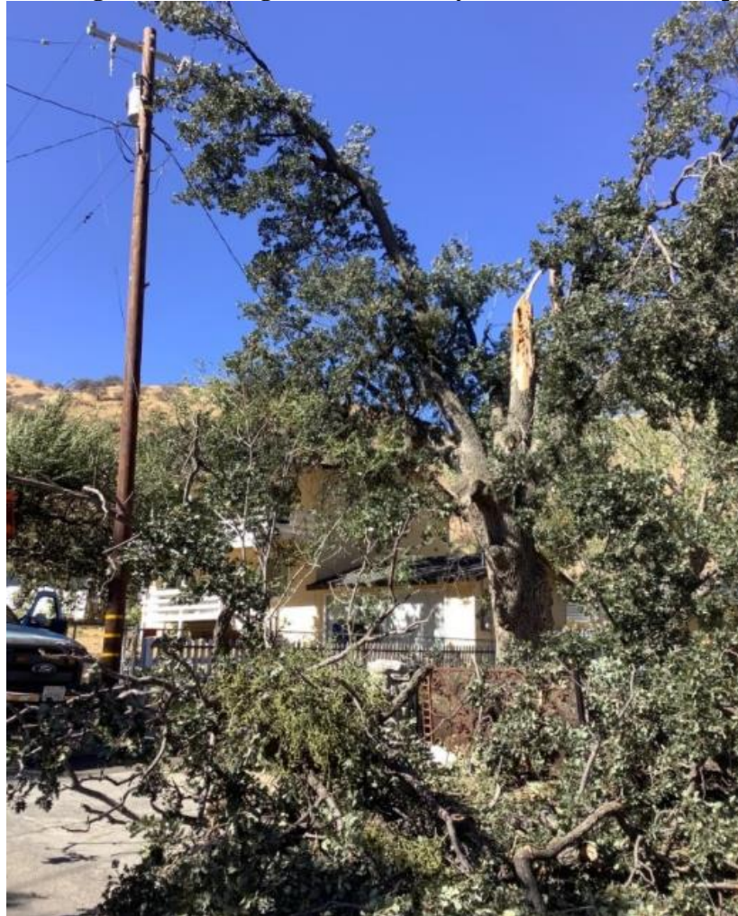
Figure 23: Vegetation-Damage in Kern County – Tree Limb fell onto primary
