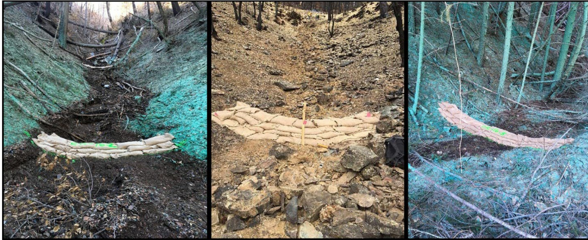
Figure 3.1.3-12. Examples of installed hydro mulch and gravel bag check dams (2021).
