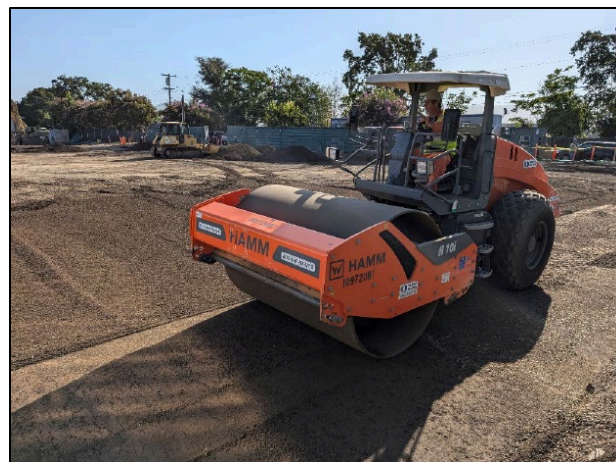
A compactor smoothed out clean soil used to backfill excavation areas.
