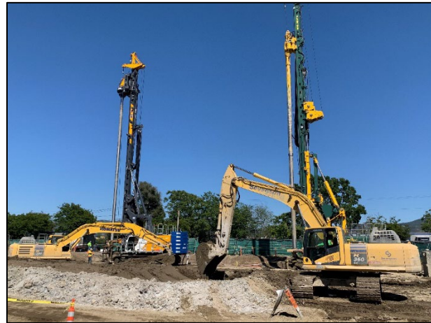
Large drill rigs were used to treat deeper soils on-site.
