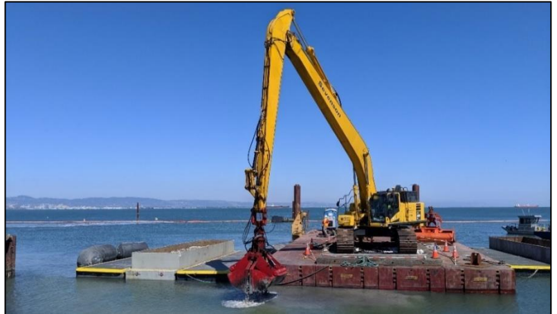
Example of offshore material dredging work
