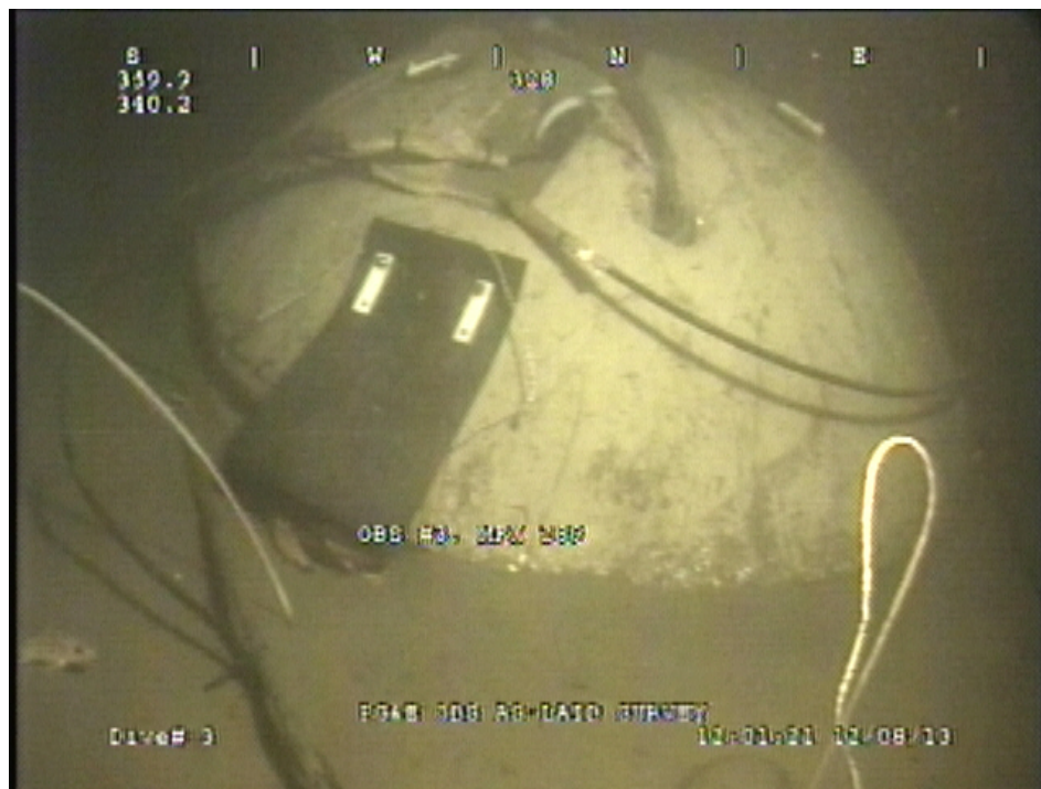
Figure 6. Video-Still of OBS-3 and Installation Bridle (Water Depth 340 ft. [104 m])
