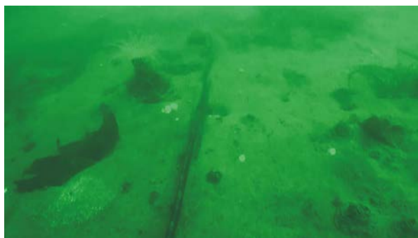
Segment 2 at 29:30 run time with cable crossing over a sand pocket area.
