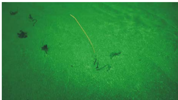
Segment 1 at 00:40 run time with cable buried under sand with tie-wrap protruding.
