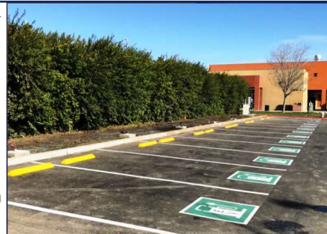
Completed striping and preparation for EV charger installation at first site, Merced Community College, Los Banos
