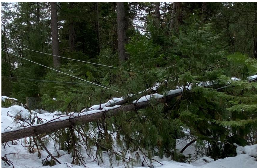
FIGURE PG&E-22-11-3: COVERED CONDUCTOR EFFECTIVENESS – EXAMPLE 3
