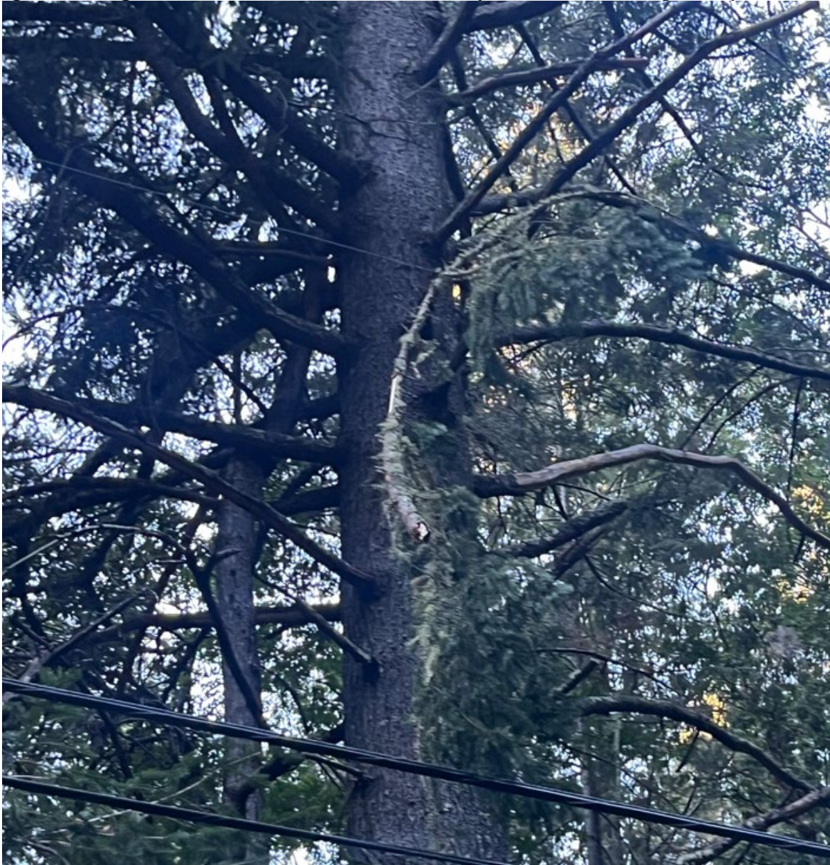
Figure 18: Vegetation-Hazard in Santa Cruz County – Tree branch on primary conductor
