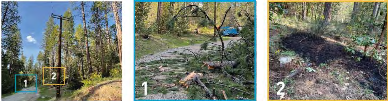
FIGURE PG&E-22-11-2: COVERED CONDUCTOR EFFECTIVENESS – EXAMPLE 2
