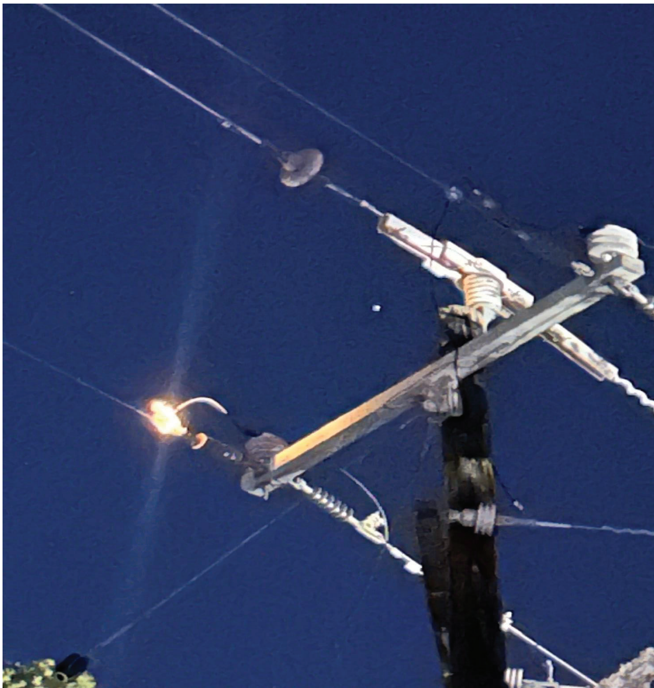
Figure 5 – Close-up view of the arcing and burnt jumper at the dead-end strain bolted clamp shoe attached to the insulator. Picture taken by the troubleshooter on June 25, 2024
