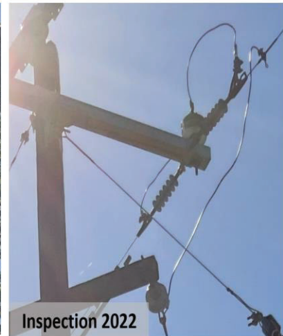
Figure 7 - The vegetation fire was ignited by molten material dripping from a failed H-connector that linked the copper jumper to the Aluminum Conductor Steel-Reinforced (ACSR) conductor.
