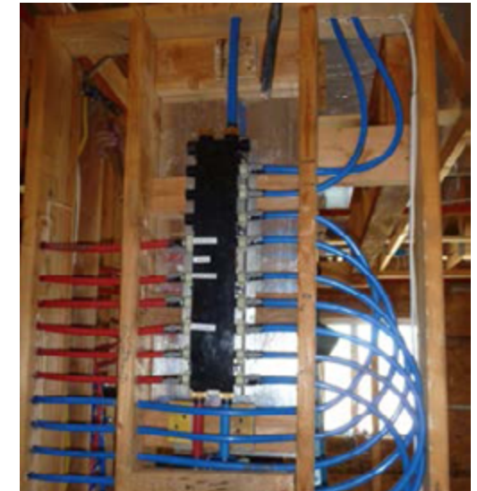
Figure 5-2. Water distribution manifold and installation schematic (Courtesy of Habitat for Humanity – San Joaquin)
