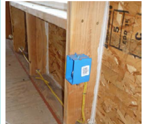
Figure 3-12. Studs pre-drilled for wiring
