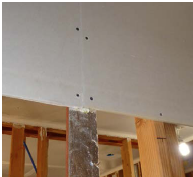
Figure 3-11. Drywall splicing
