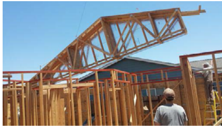
Figure 3-10. Ground-constructed gable-end truss assembly being craned into place
