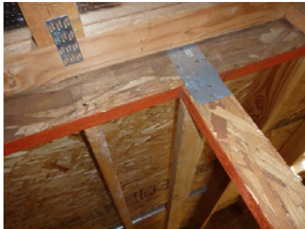
Figure 3-7. Engineered single top plate, from above
