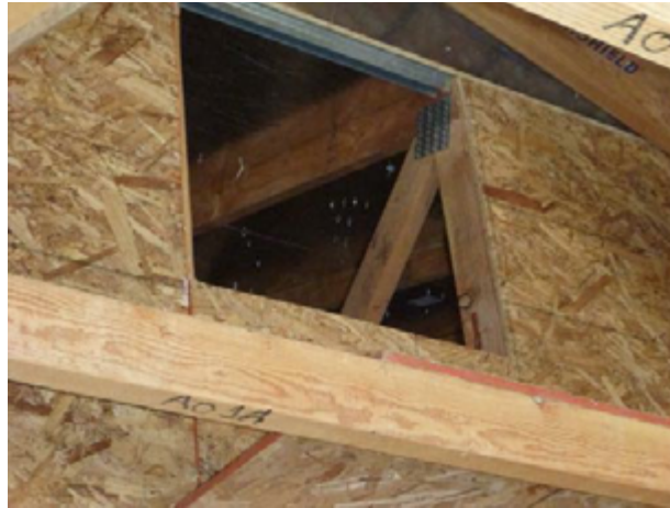
Figure 3-6. Attic access in garage – not penetrating ceiling insulation
