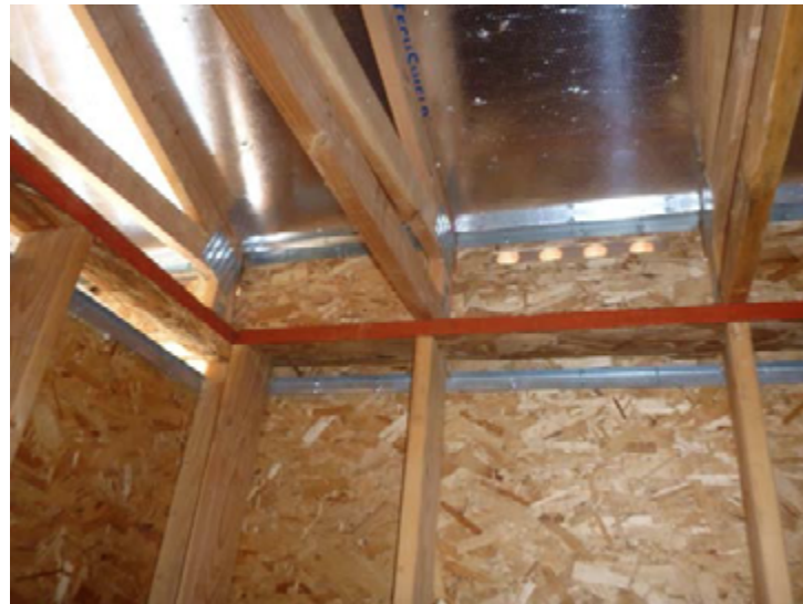
Figure 3-5. Raised heel trusses
