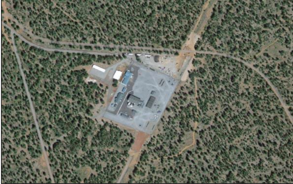
Figure 3.1.2-35. Burney compressor station satellite imagery (Google, 2022).
