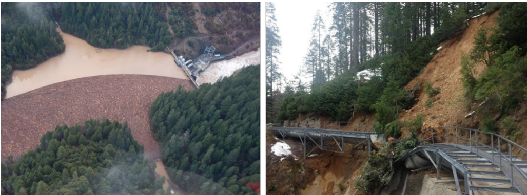
Figure 3.1.3-4. Woody tree debris captured by log boom in 2017 at the Pit 6 dam (left); landslide damage to PG&E's water conveyance (right).
